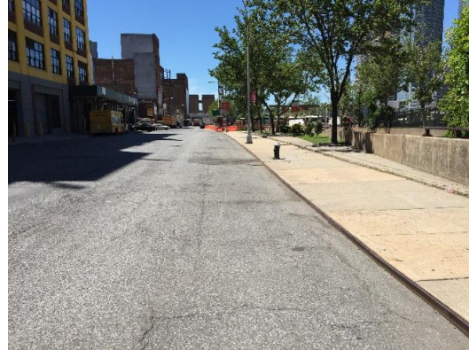
North side of 39 th St., west of 10 th Ave
