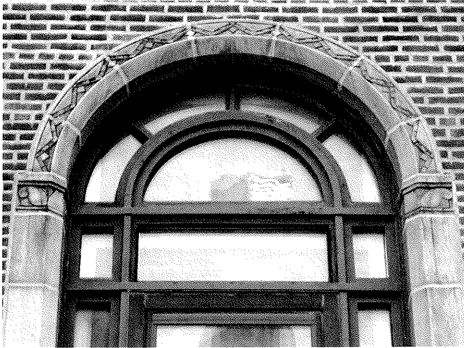
17. North façade arched terra cotta window head.
