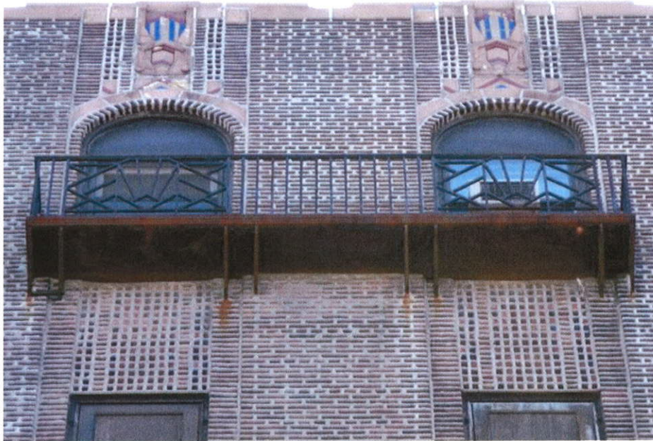
15. North façade balcony and arched windows with terra cotta motif above.
