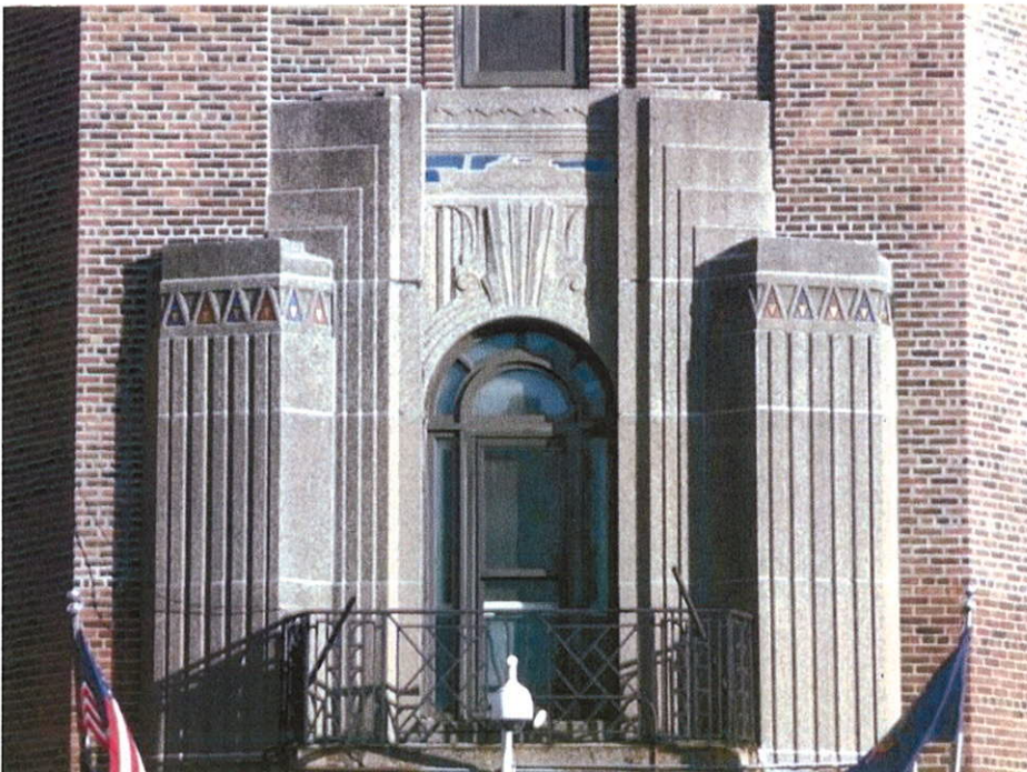
6. Upper entrance detail.
