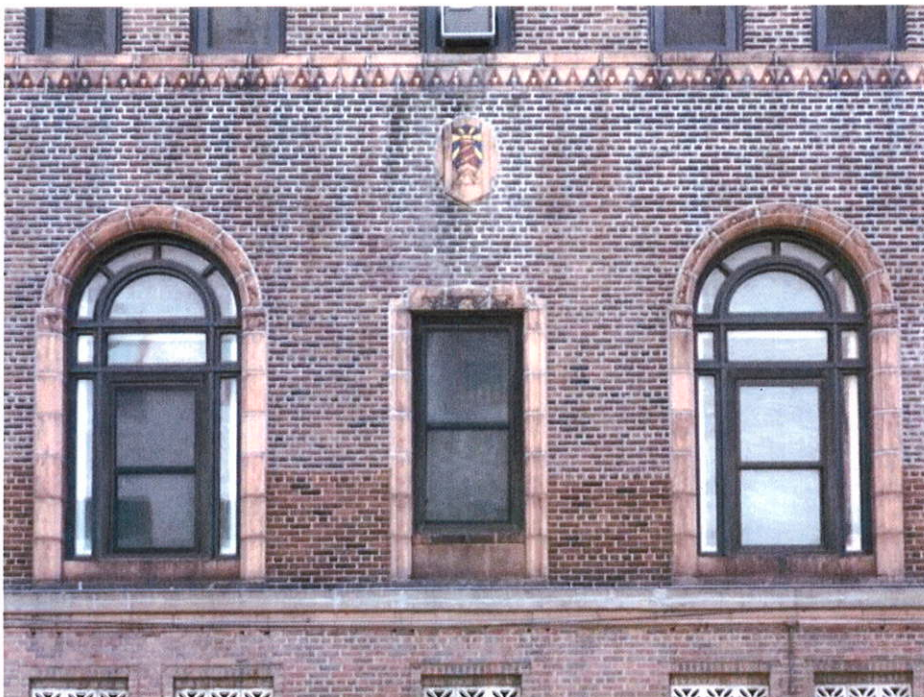
16. North façade window grouping with terra cotta string course, lighthouse medallion and modeled window surrounds.
