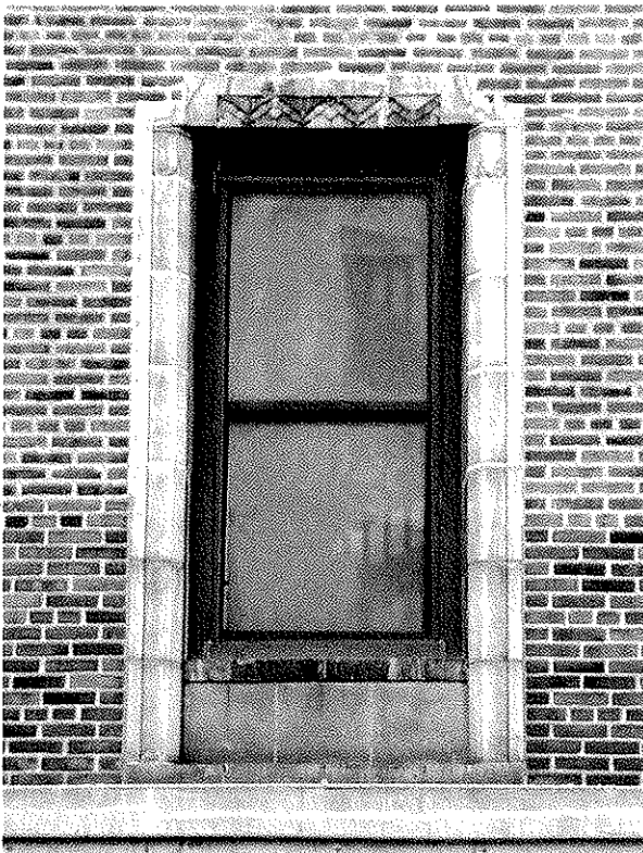
18. North façade terra cotta window surround.
