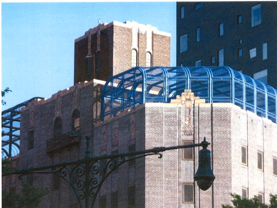
20. Penthouse view from northwest.
