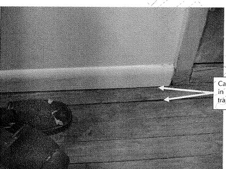
Caulking the cracks in the floor in 1D will also reduce the sound transmission of people's voices.
