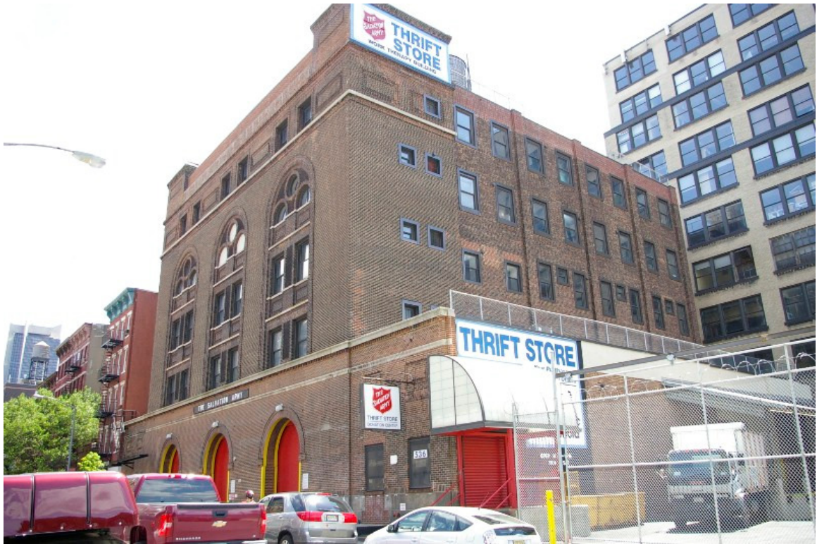
Acker, Merrill & Condit Company warehouse, 536 West 46th Street – S/NR-eligible
