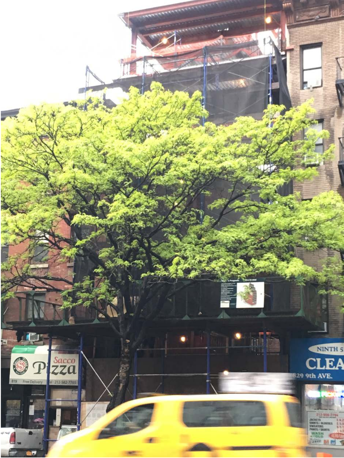
APPENDIX A – Pictures of 821 9 th Avenue, dated May 6, 2016
