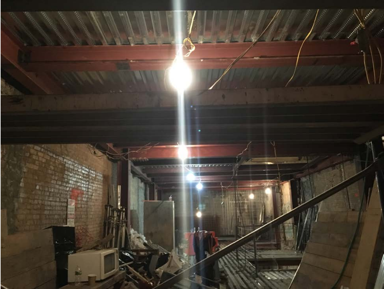
APPENDIX A – Pictures of 821 9 th Avenue, dated May 6, 2016
