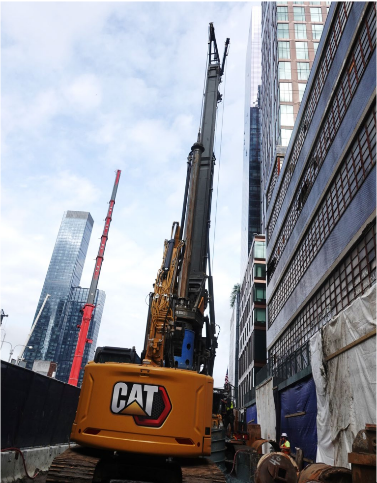
Interim Ramp W99 (8/18/2026)
