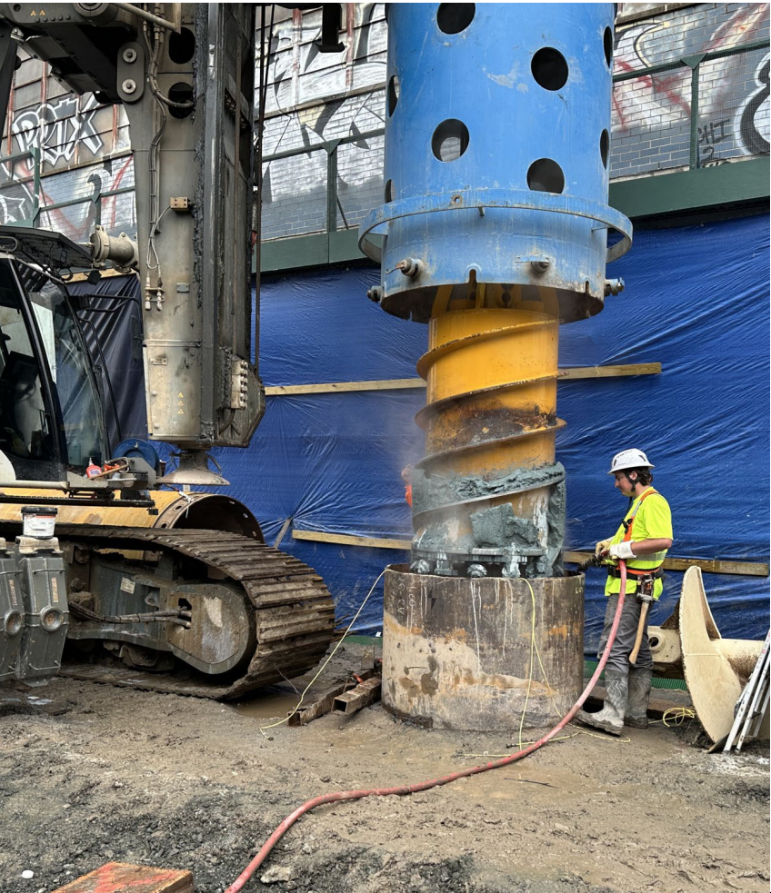
Interim Ramp W99 (8/17/2026)
