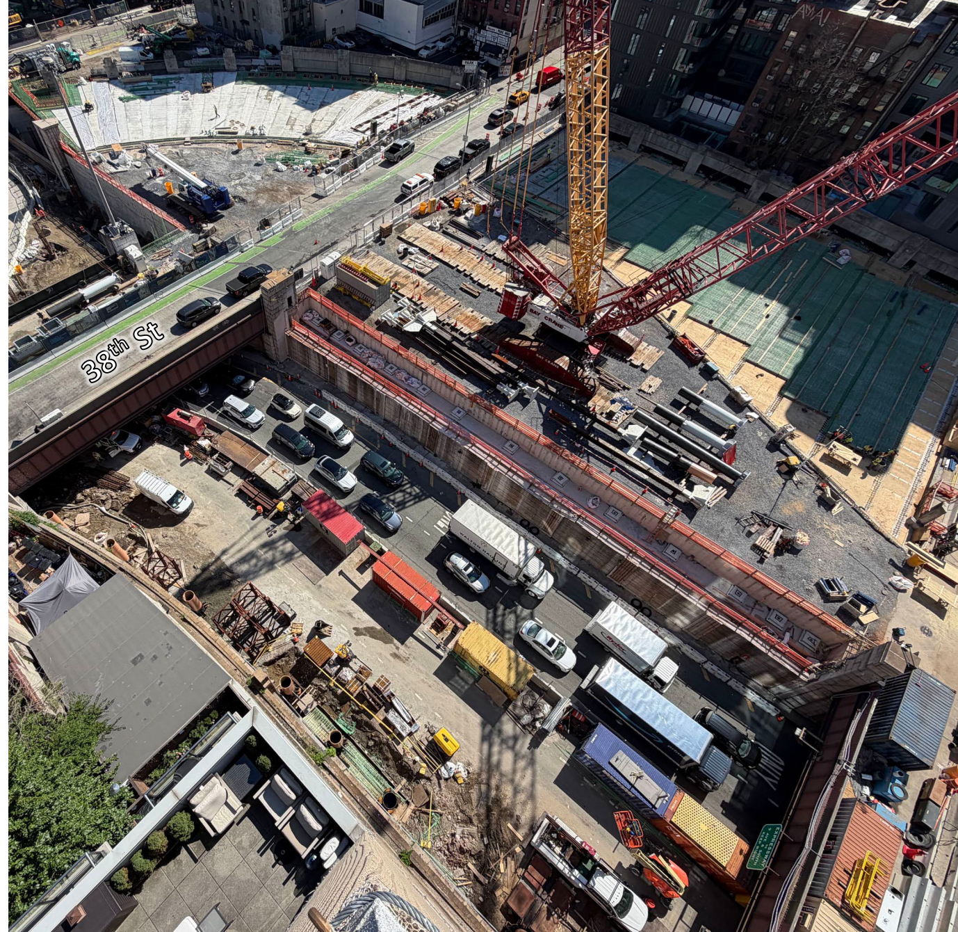
Aerial view of the Dyer Deck Overs work site (8/19/26)
