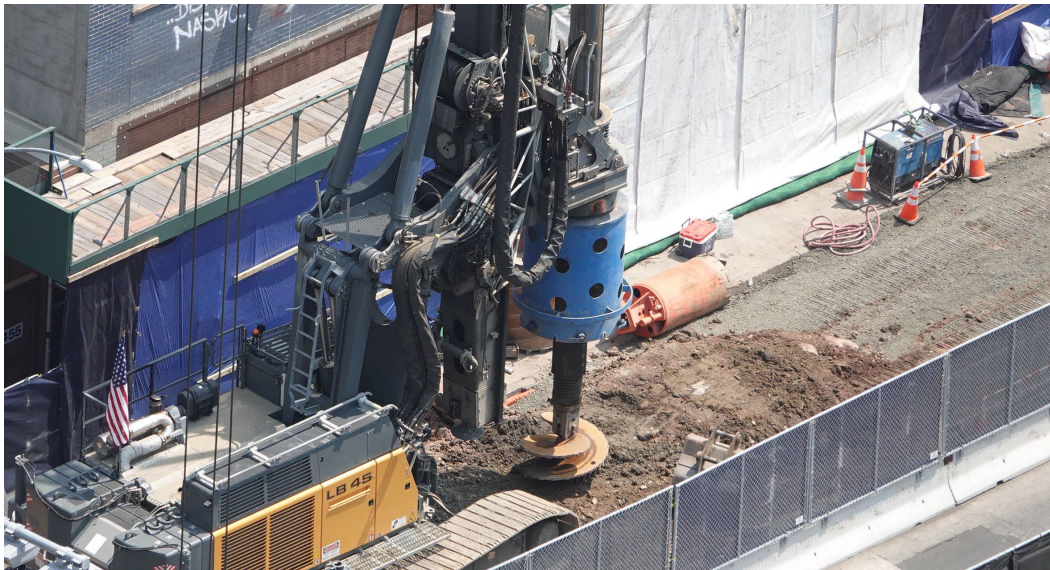
Drilling Operations on 40 th Street July 27
