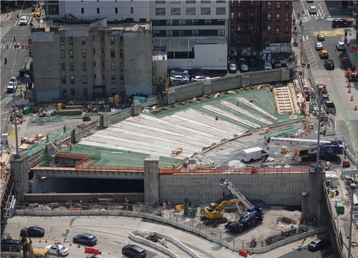
Cast in Place Concrete Operations at LTE North July 27
