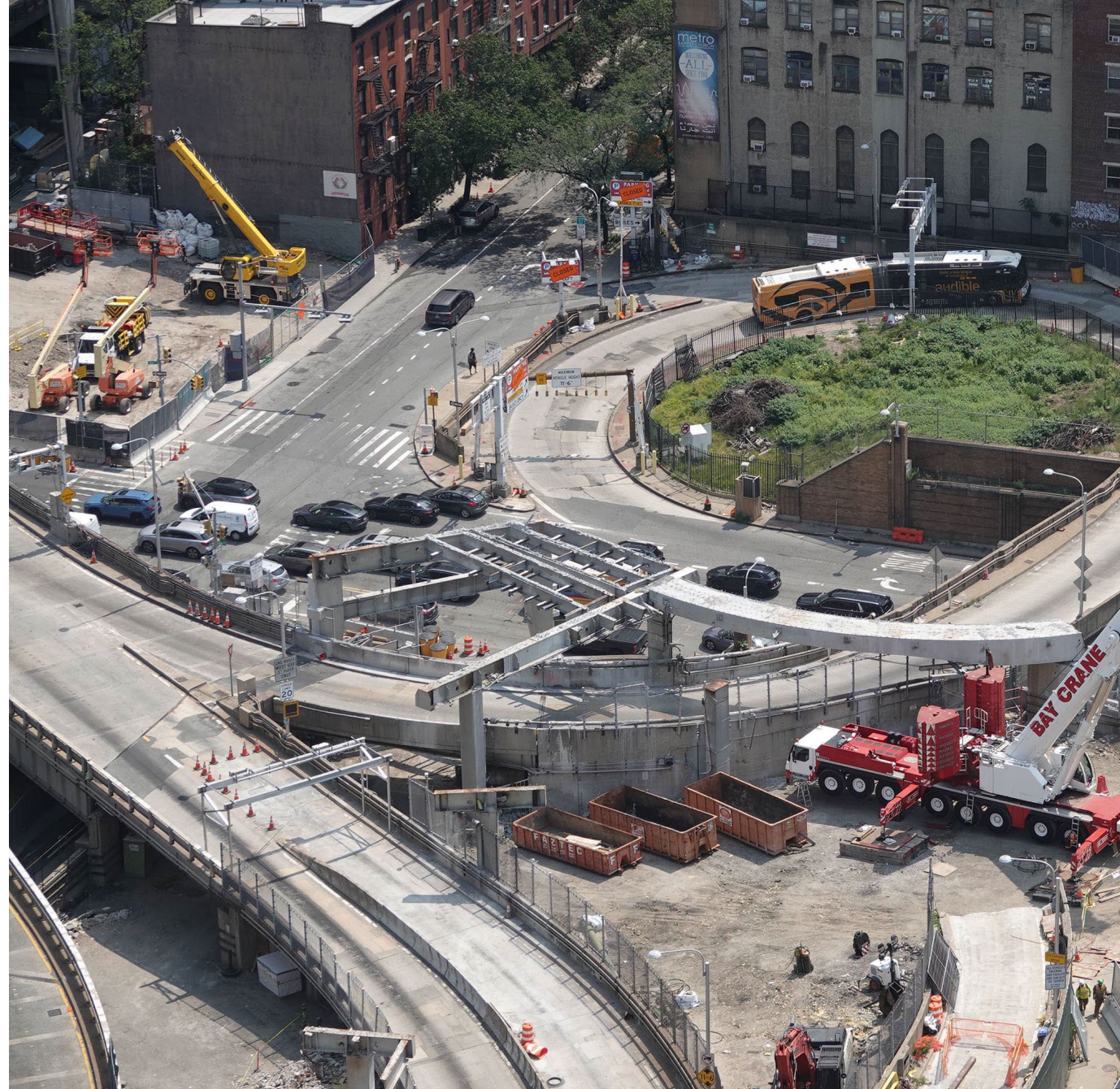
Aerial view of the Kinney Ramps Demolition progress (7/27/26)
