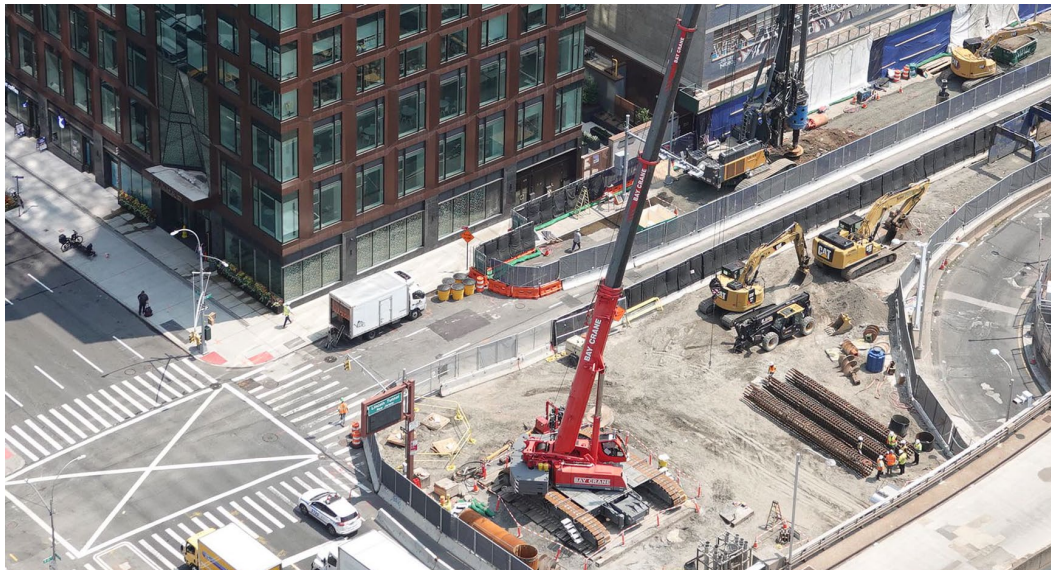
Drilling Operations on 40 th Street and Lot E July 27
