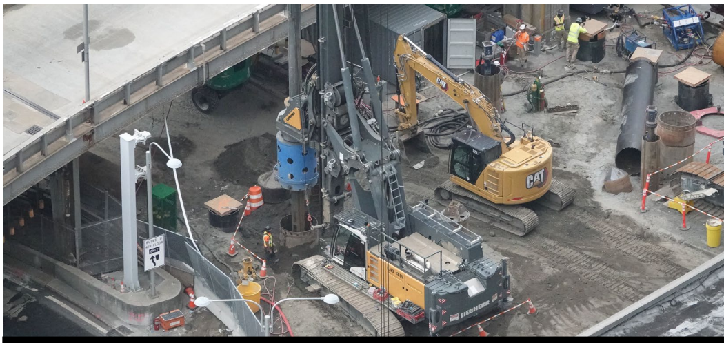
Drilling Operations in Lot E July 27
