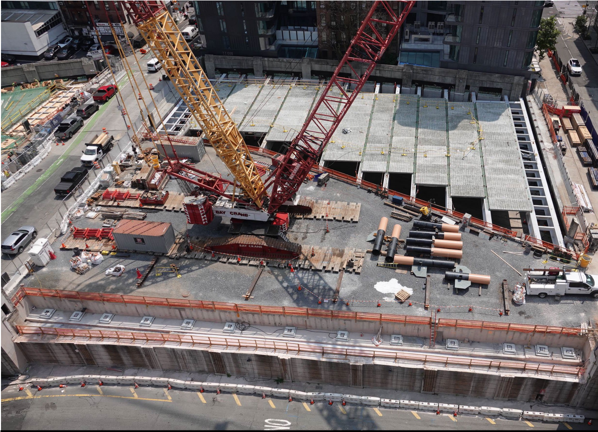
Steel Girder Erection and Precast Panels at LTE South July 27
