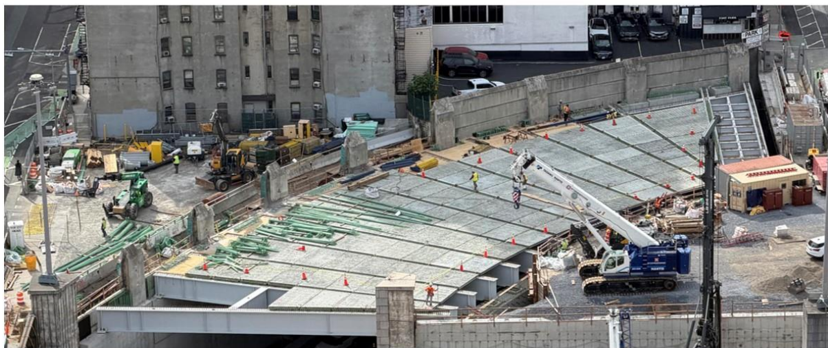
Precast panels on Steel girders over LTE (6/17/26)
