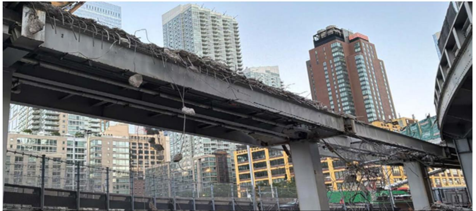
Removing Slabs and Decks next to active ramps (6/17/26)
