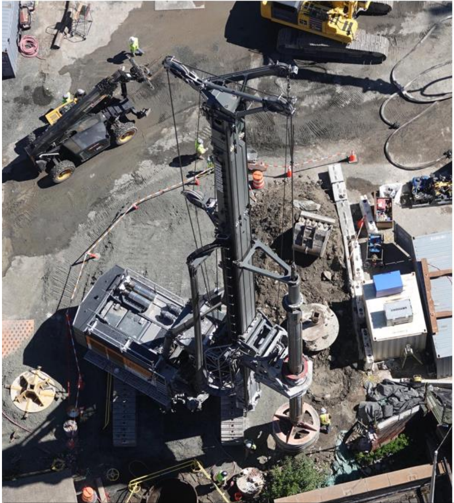
Caisson Installation in Lot F (6/17/26)
