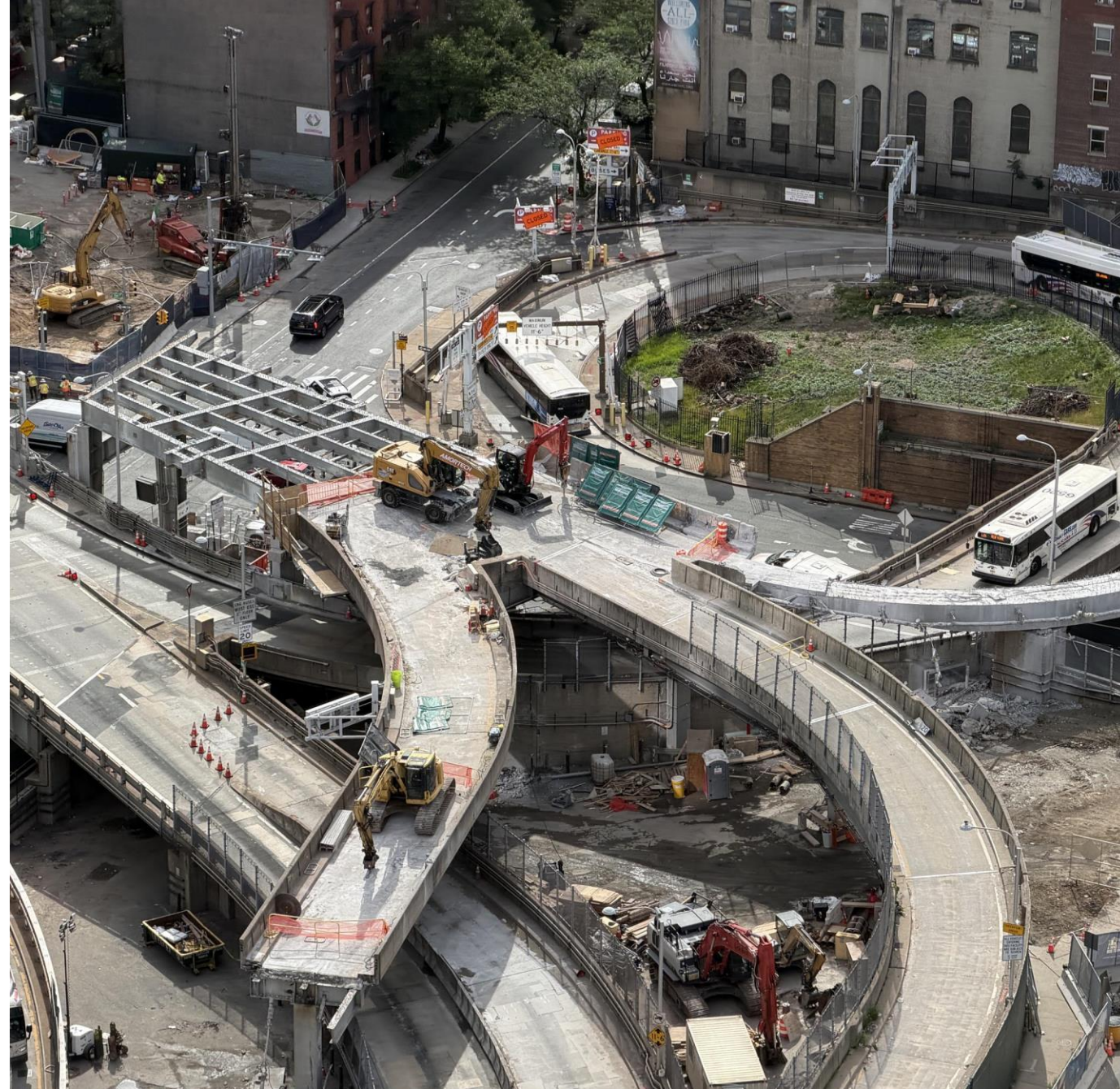
Aerial view of the Kinney Ramps Demolition progress (6/19/26)
