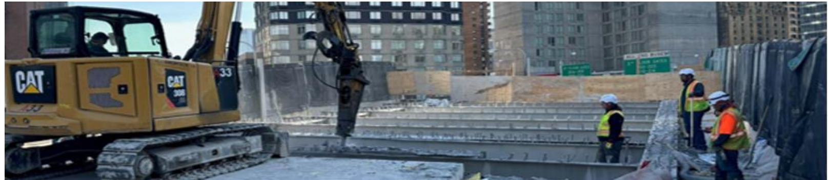
Removing Slabs and Decks (6/17/26)
