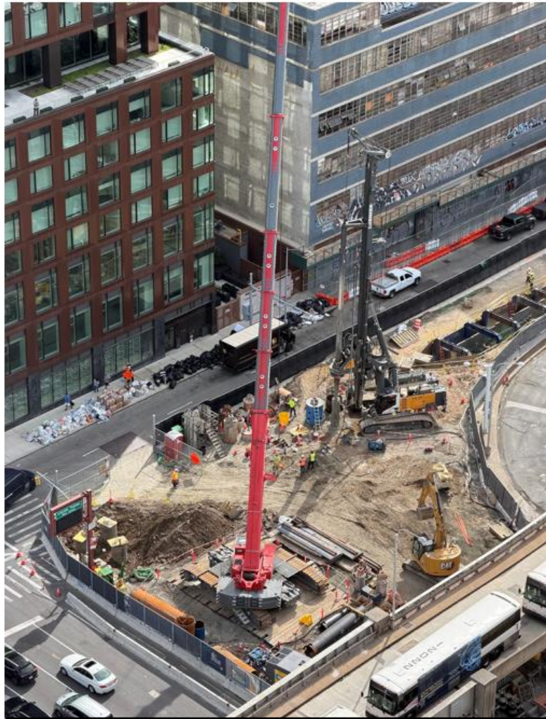
Caisson Installation in Lot E (6/19/26)
