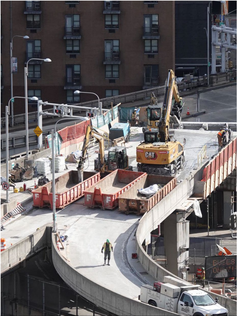
Slab and Deck Removal at Kinney Ramps (5/26/26)
