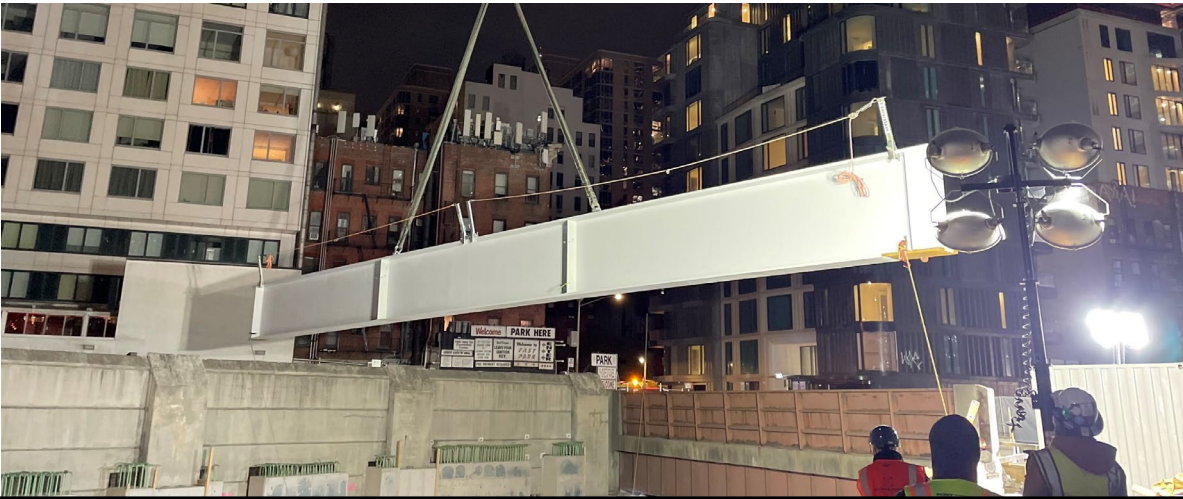
The first Steel Girder installed over the LTE (4/21/26)
