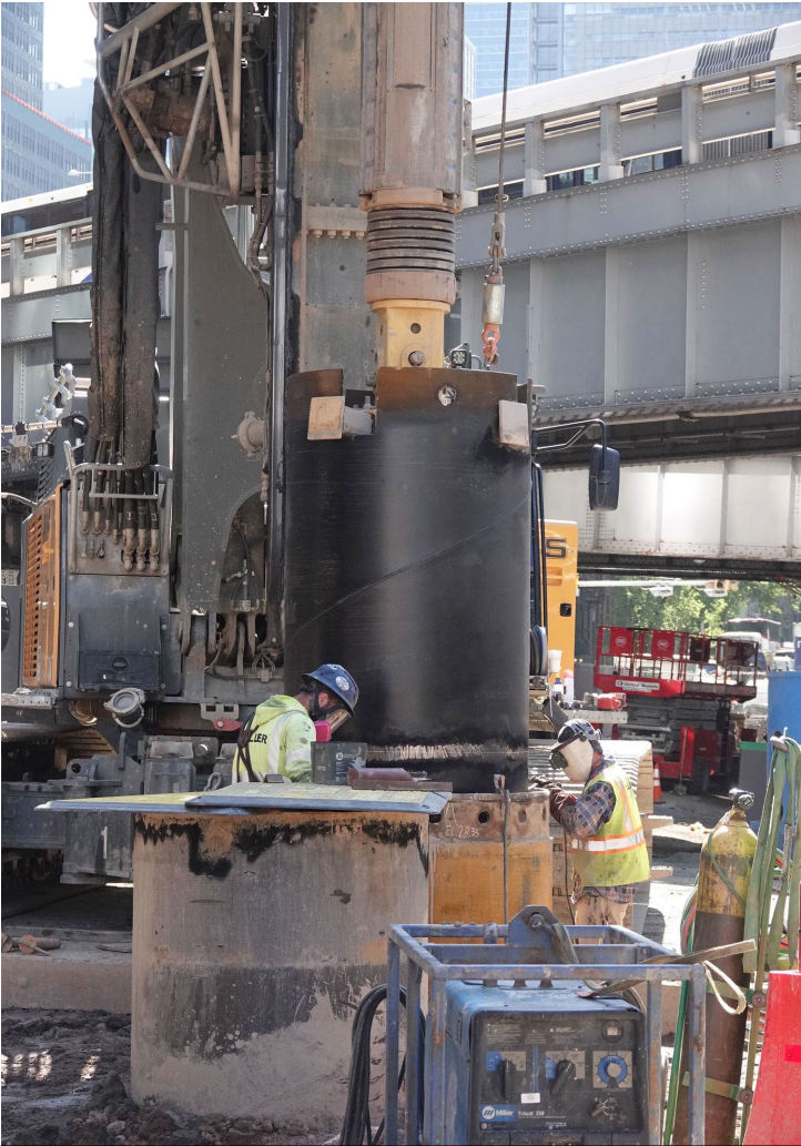
Drilling Production Shafts in Lot E (5/19/26)
