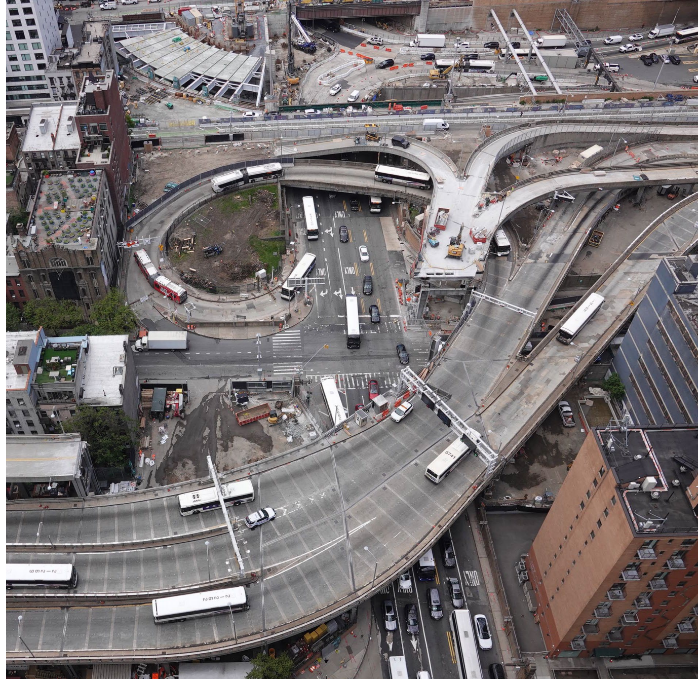
Aerial view of the Kinney Ramps along Dyer Avenue looking south (5/19/26)
