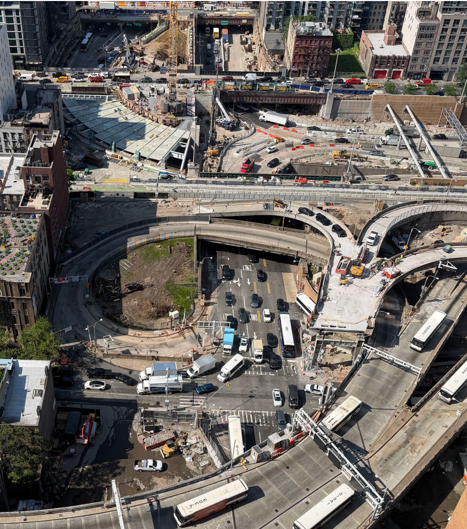
Deconstruction at the Kinney Ramps (5/19/26)
