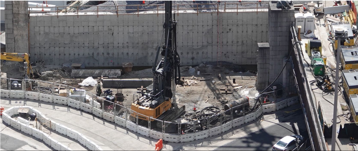
Drilled Shafts in Dyer Plaza (5/8/26)
