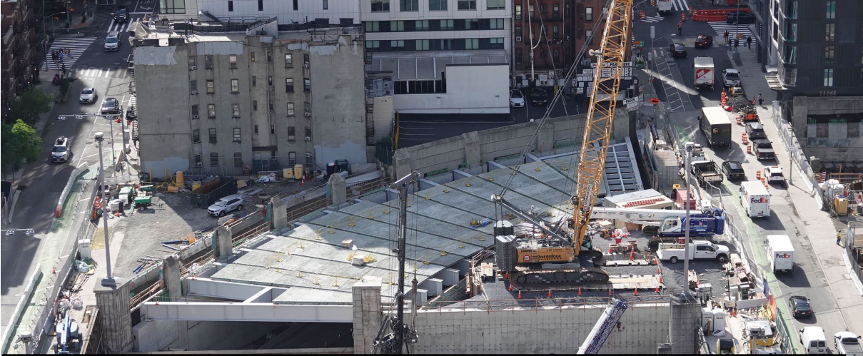
Precast panels on Steel girders over LTE (5/26/26)
