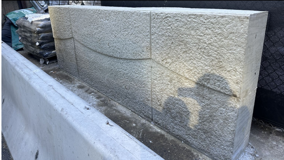
Concrete Parapet Mock-up
