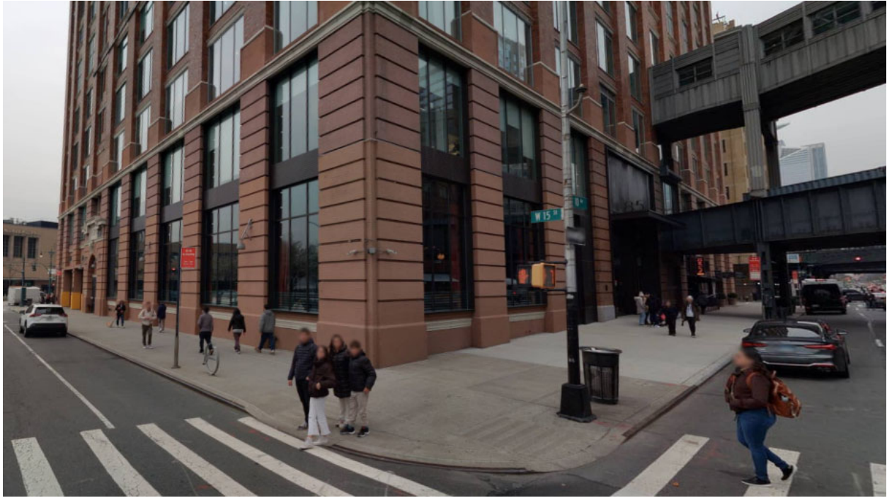
Photo 1: View of Site, looking northwest along 10 th Avenue and W. 15 th Street
