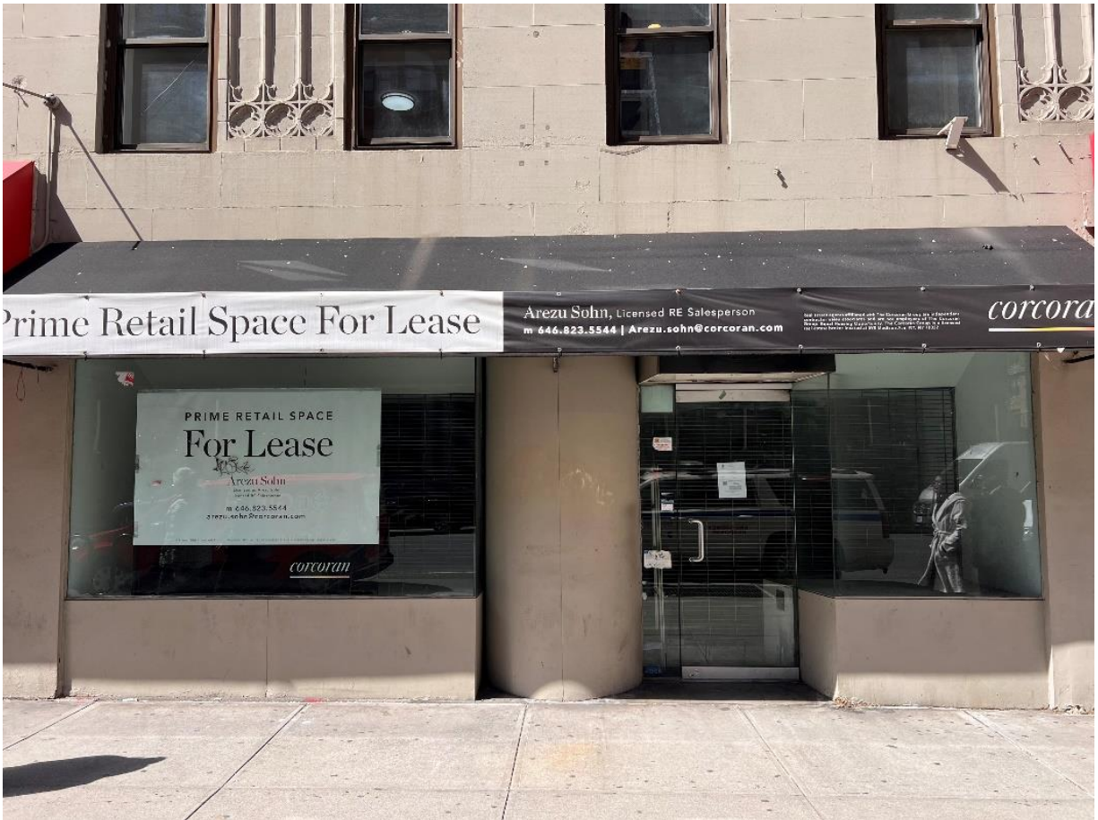
Photo 1: View of Site from Seventh Avenue
