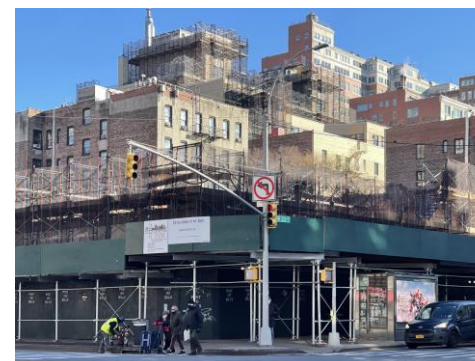
Existing site, demolition underway as of April 2022
