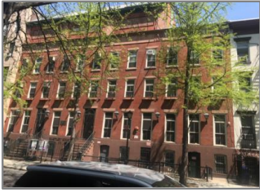
413 W 46 th Street: Hartley House
