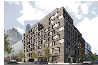
806 9th Avenue: MTA Site
