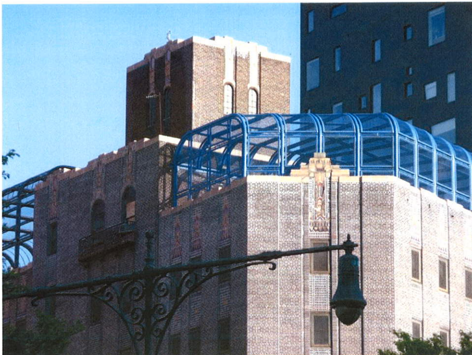
20. Penthouse view from northwest.
