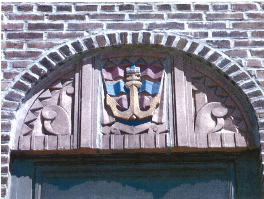
12. West façade terra cotta window head with anchor motif.
