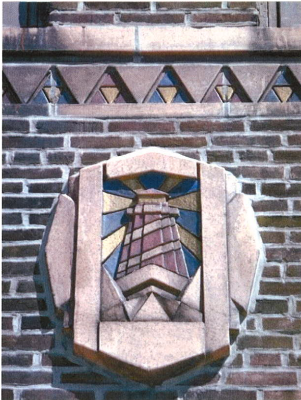
11. West façade terra cotta string course and lighthouse medallion.
