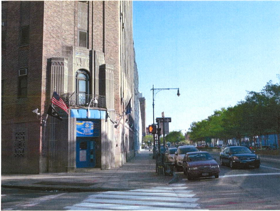
5. Entrance view from north.
