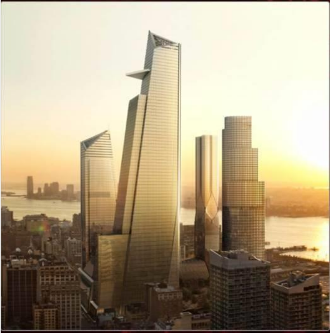
Exterior of Premises
