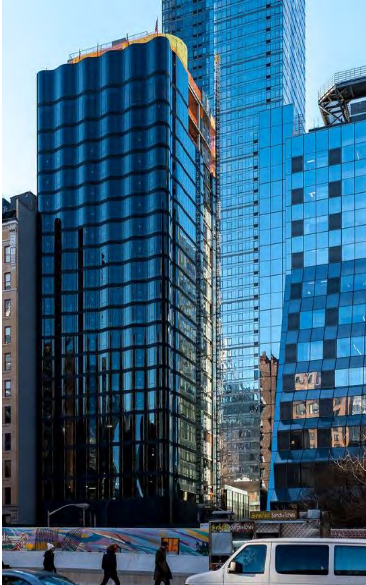
View from West 33 rd Street
