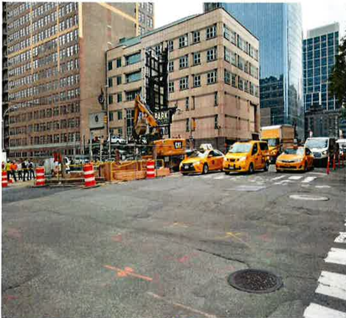
9 th Avenue, between W. 30 th & W. 31 st Streets (36" / 48" TWM installation)
