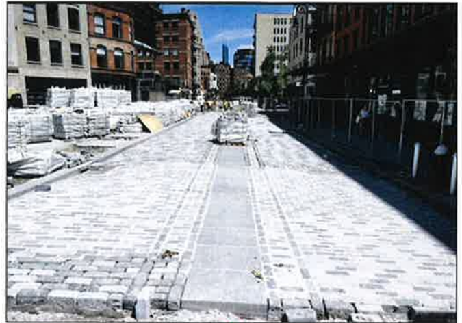
COBBLESTONE INSTALLATION ON GANSEVOORT STREET
