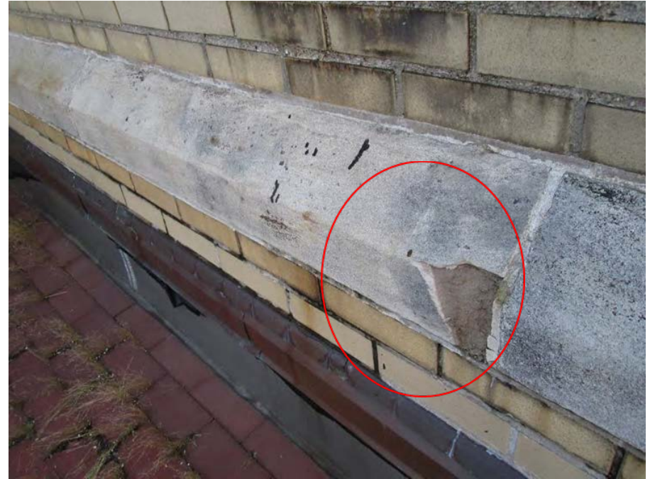
Photo: P12 Date 10/5/2015
