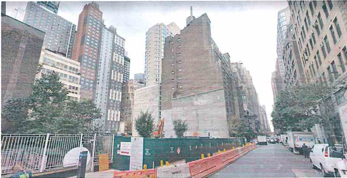
Photo 1: View of Site on W 38 th St – Looking East
