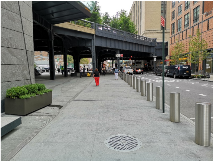
3. Looking eastward on the W. 30 th St. Street frontage from midblock btwn 10 th and 11 th Ave.
