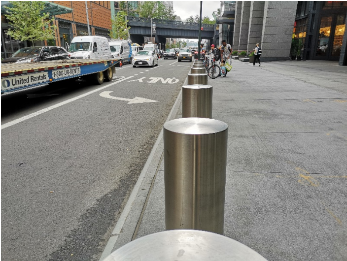
1. Looking at bollards and curb line along W. 30 th St.
