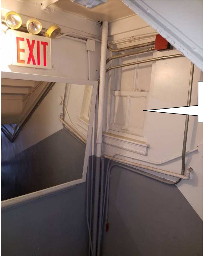
1 st floor stairwell landing, with window to courtyard shut.
