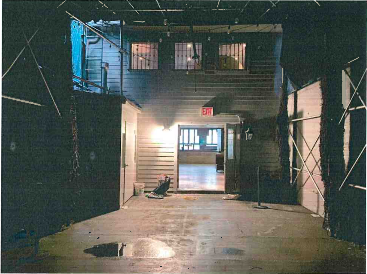
Exterior Roof to be enclosed
