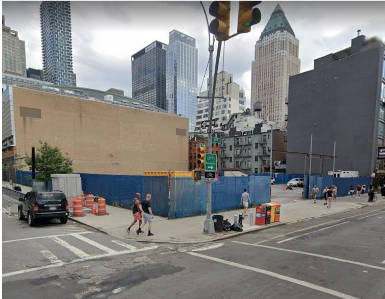
Site from corner of 9 th Ave & 54 th St
