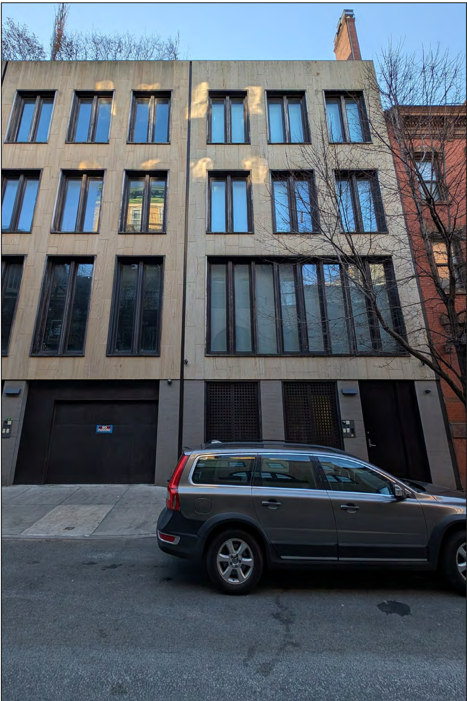
3 PHOTO EXISTING CONDITION
