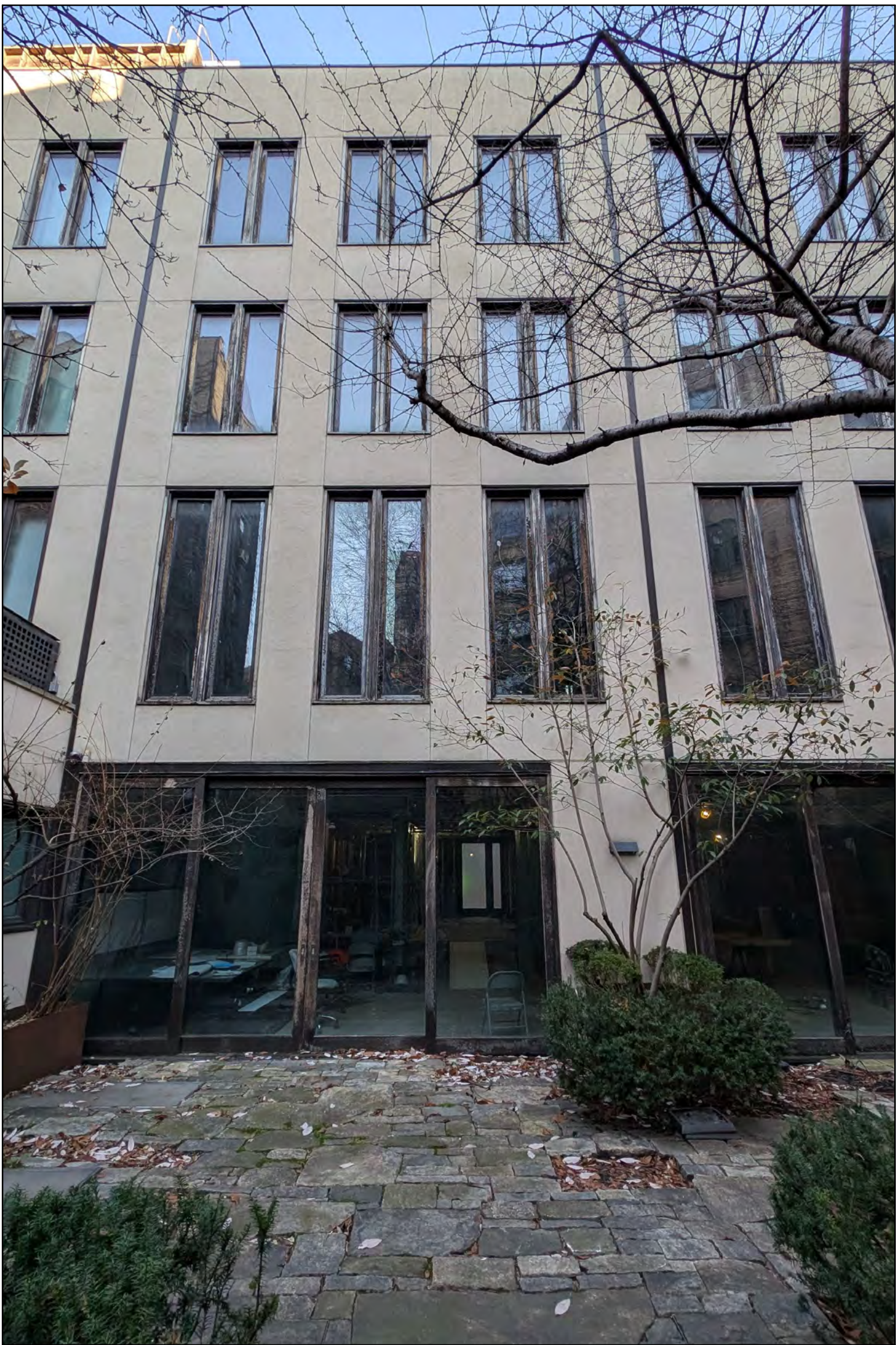
7 PHOTO EXISTING CONDITION
