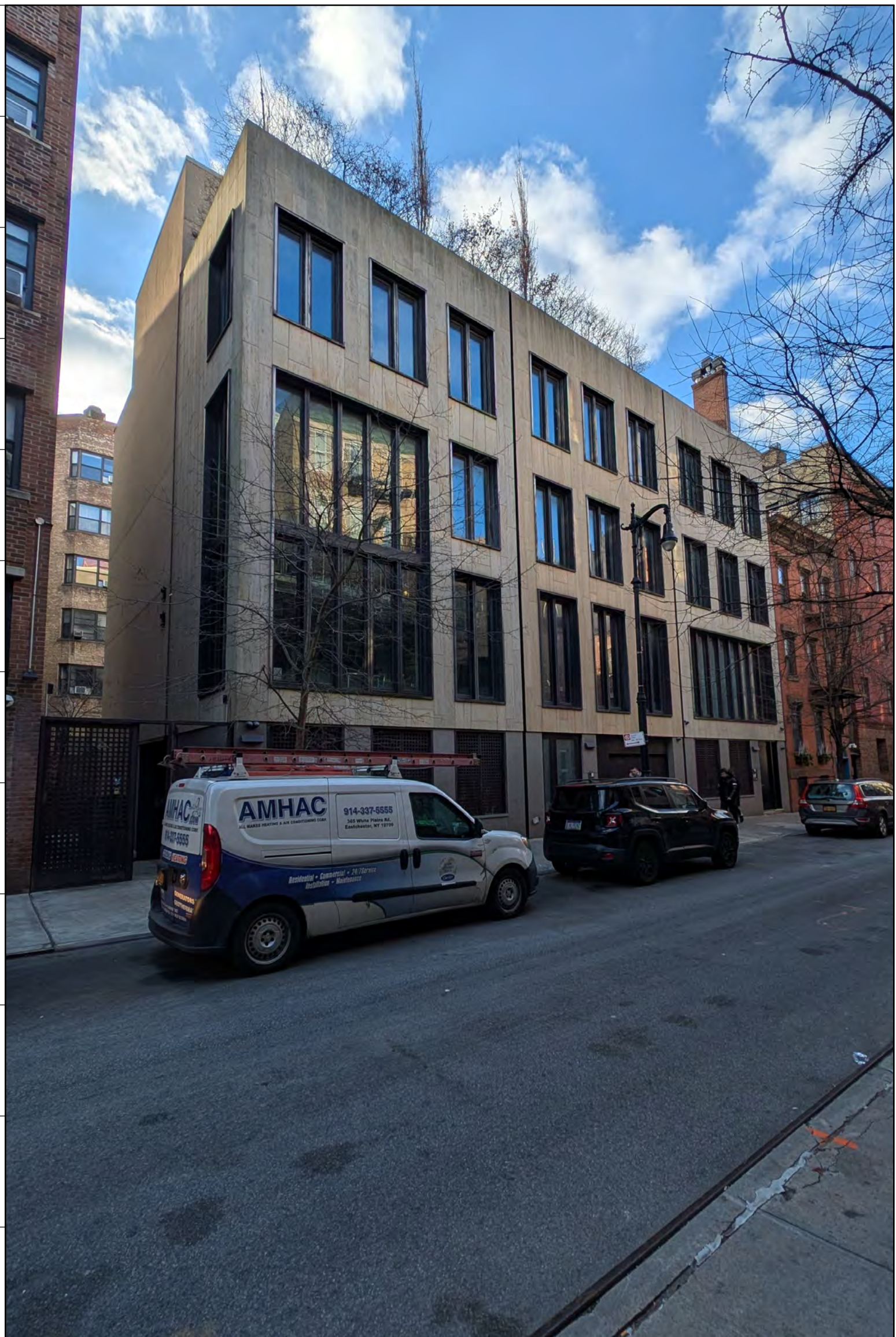
4 PHOTO EXISTING CONDITION
