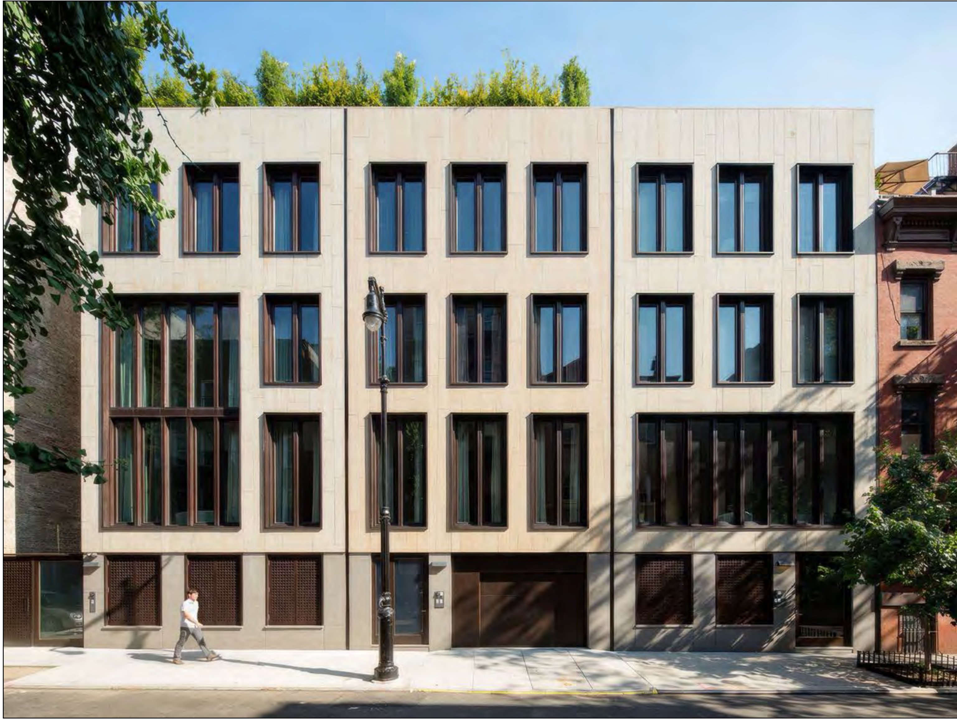
1 PHOTO EXISTING ELEVATION
