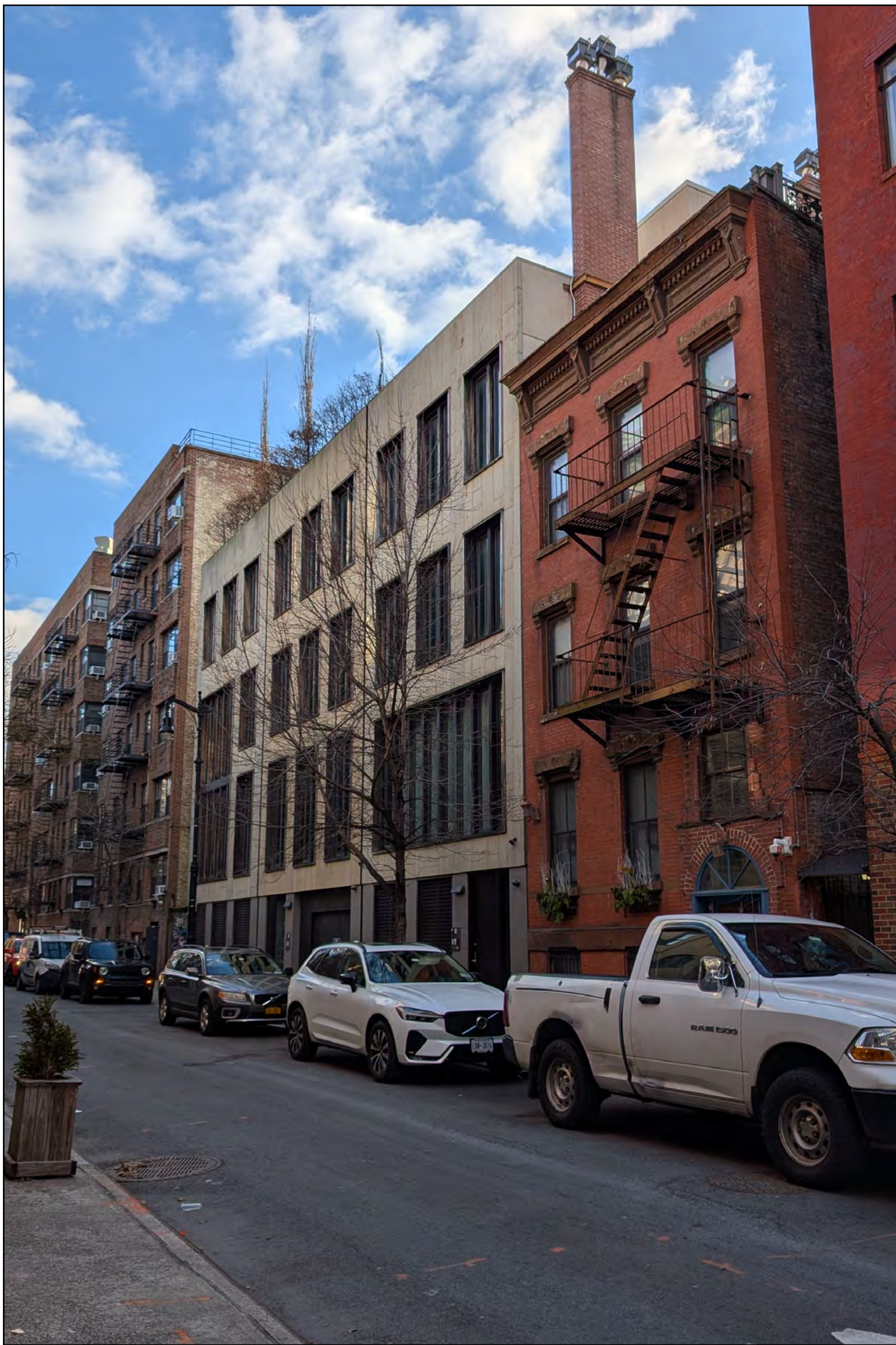
6 PHOTO EXISTING CONDITION
