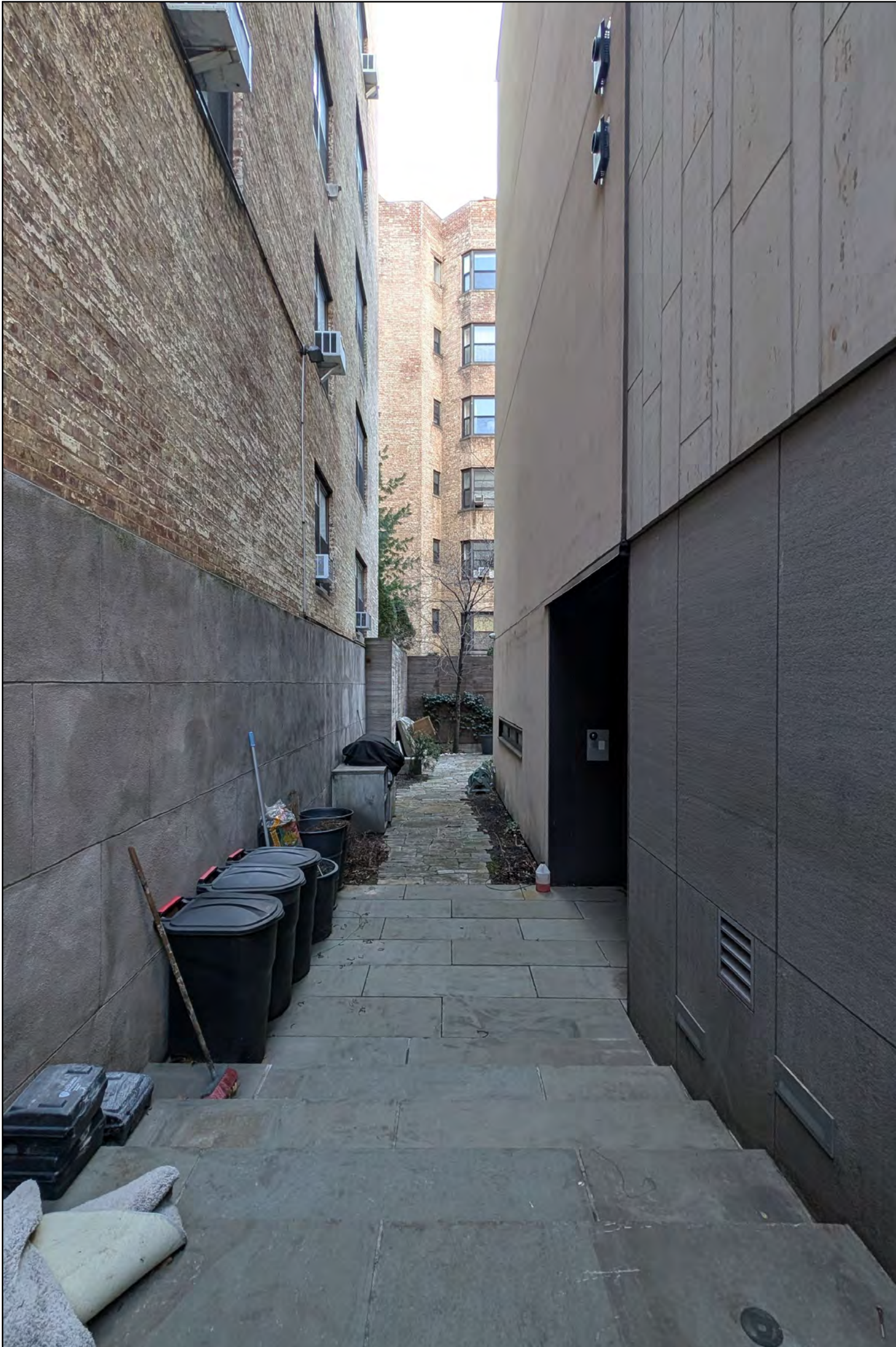
3 PHOTO EXISTING CONDITION
