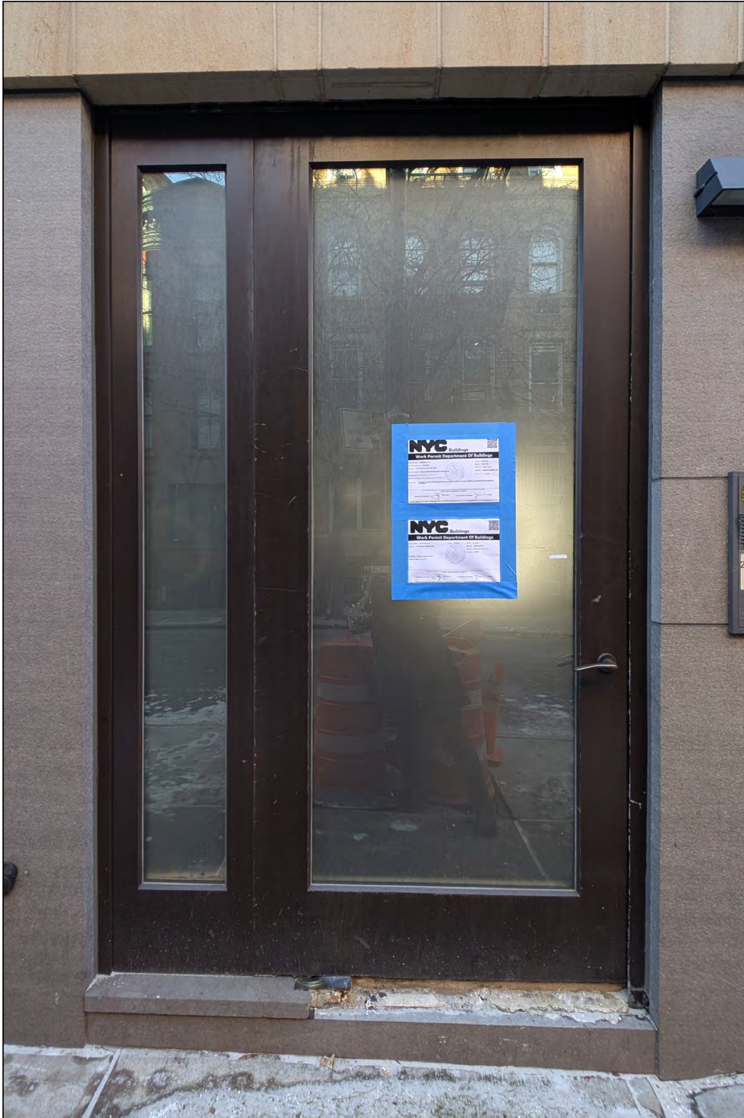
2 PHOTO EXISTING CONDITION
