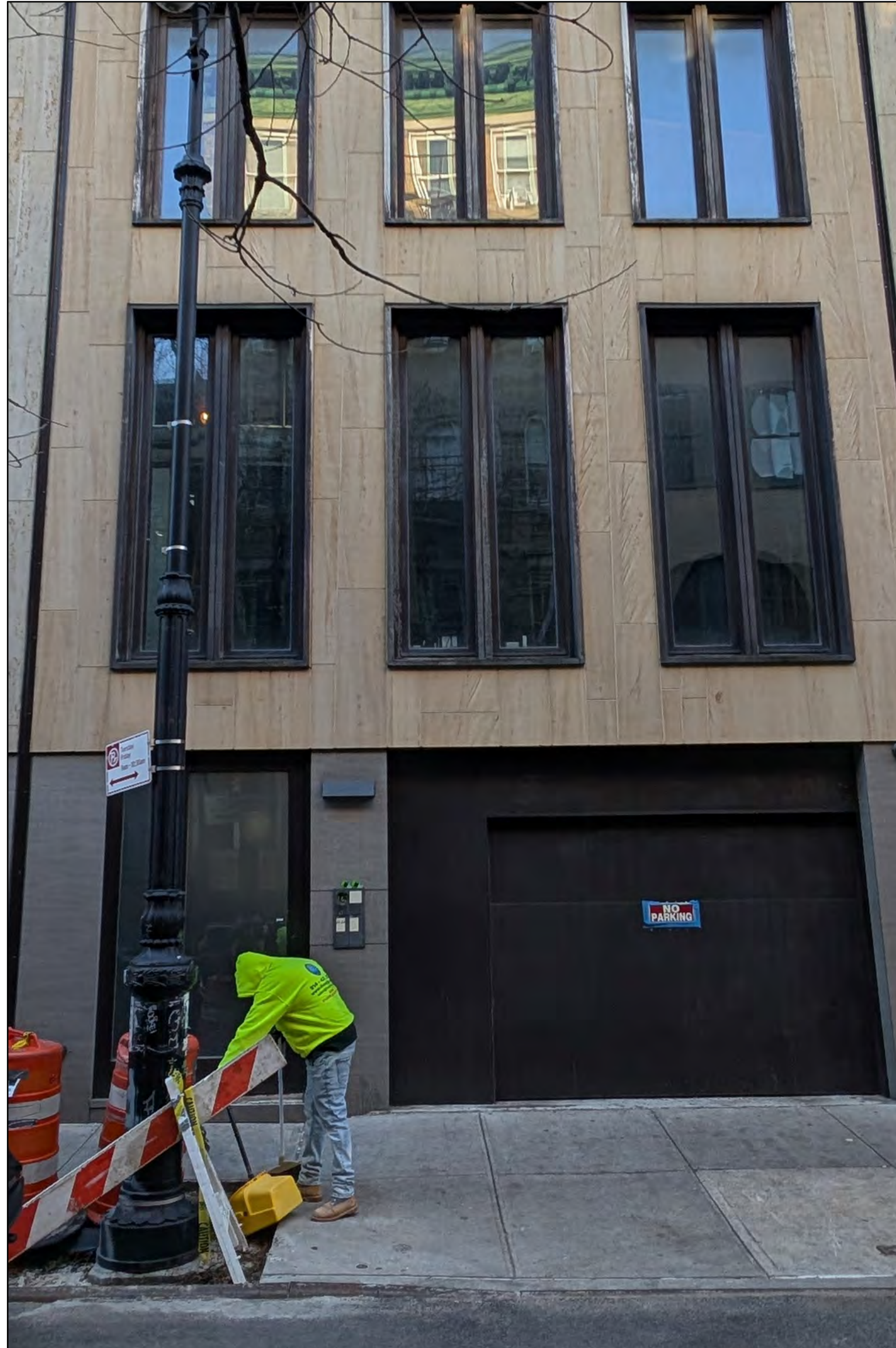
1 PHOTO EXISTING CONDITION
