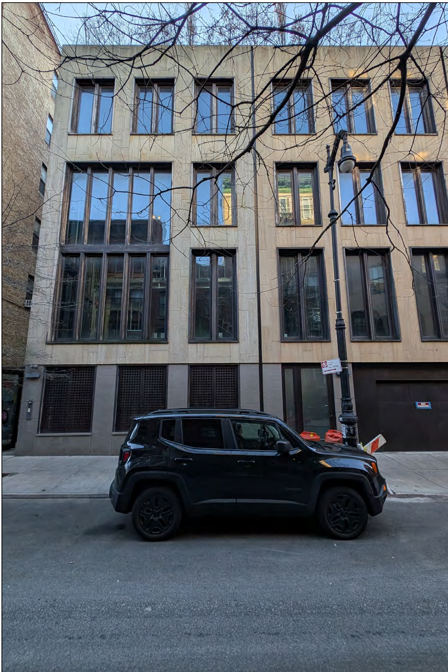
2 PHOTO EXISTING CONDITION
