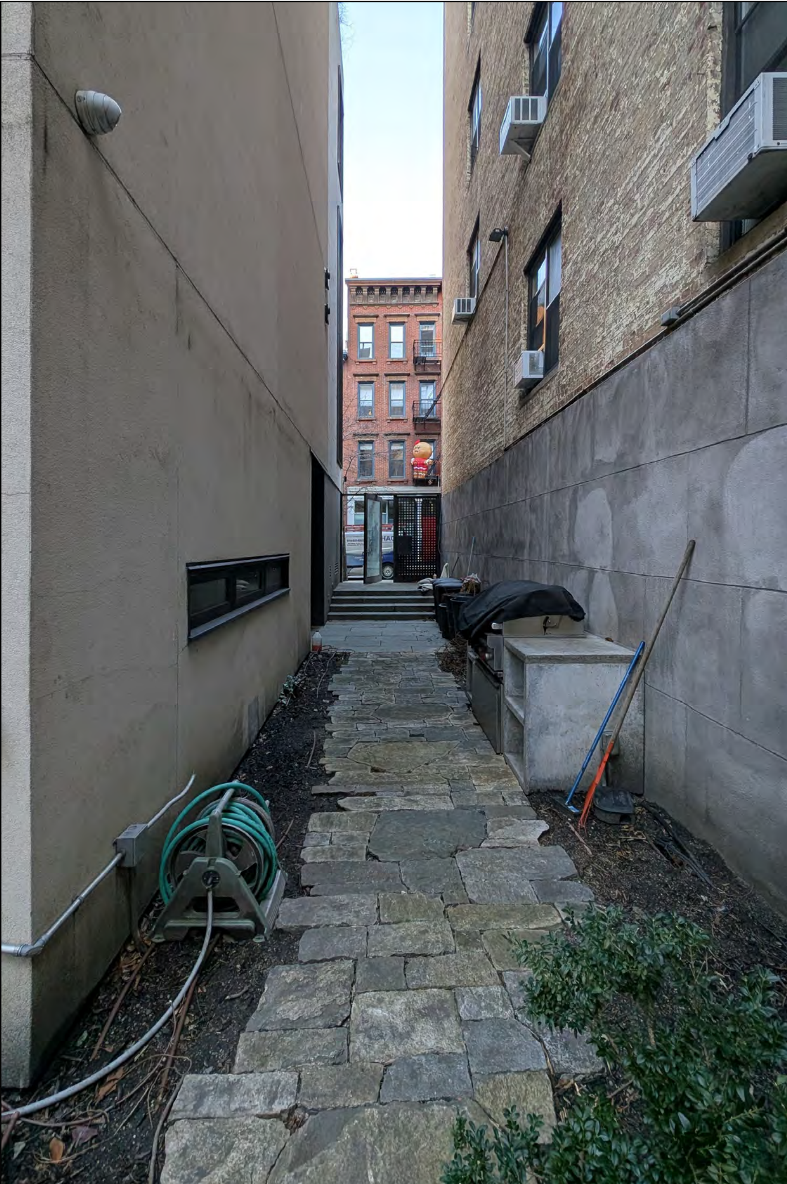
4 PHOTO EXISTING CONDITION
