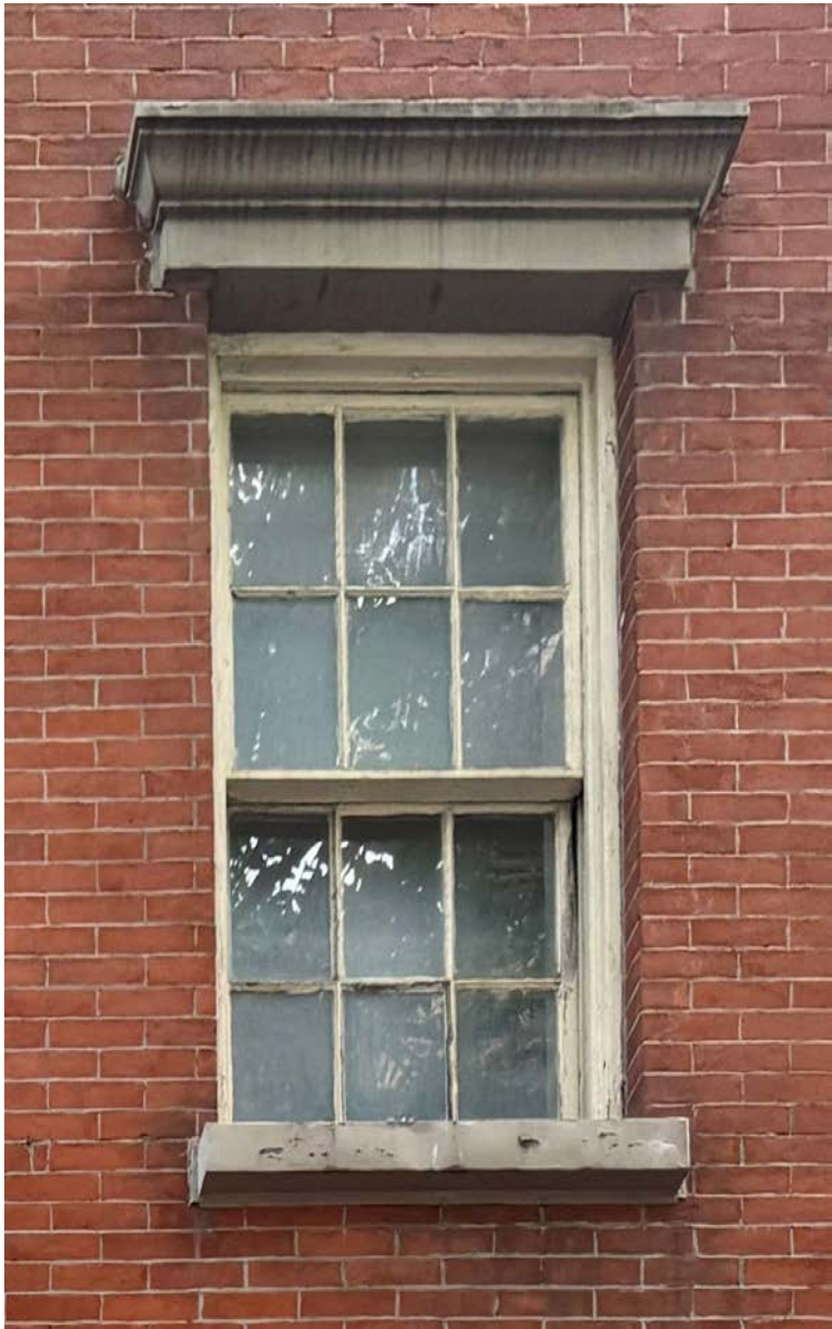
56 WEST 12 ST EXISTING DOUBLE-HUNG WINDOW
