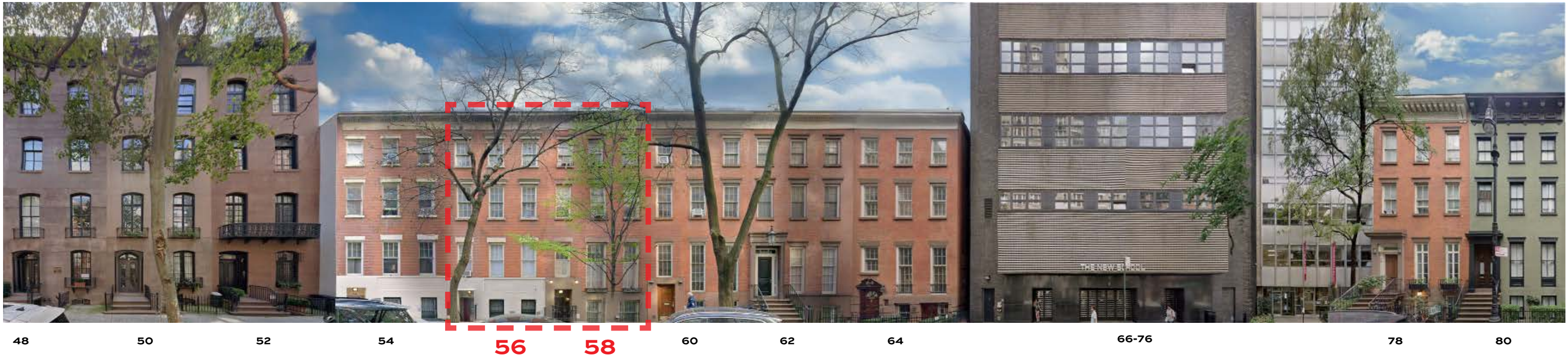
Existing Conditions: South Elevation of West 12th St
