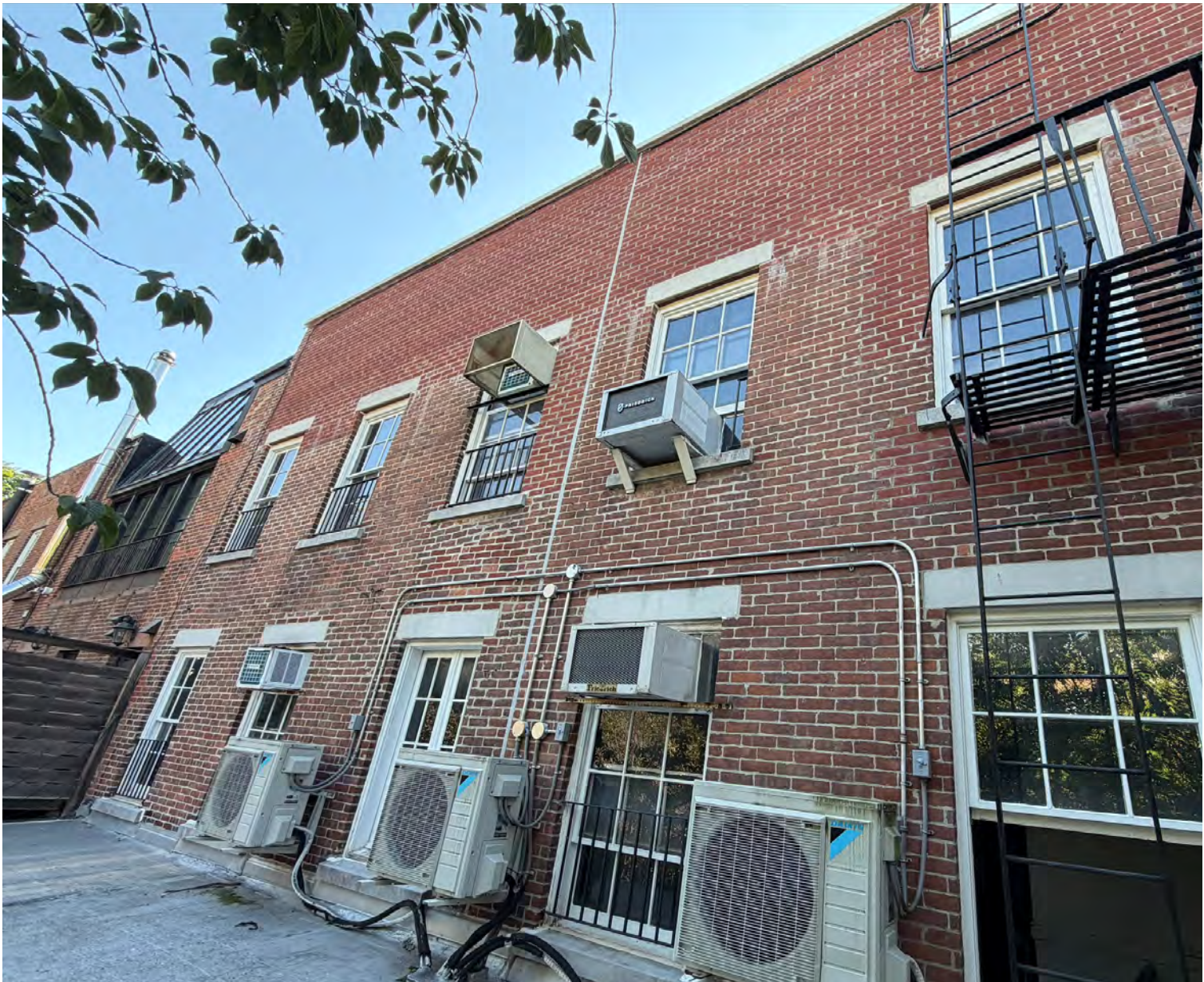
UPPER REAR FACADE LOOKING EAST (TOWARDS #42)
