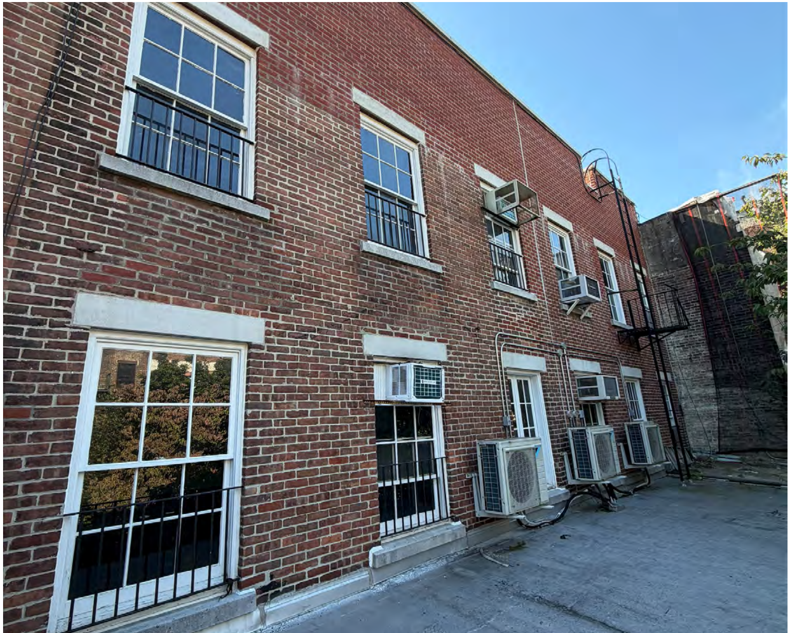
UPPER REAR FACADE LOOKING WEST (TOWARDS #48)
