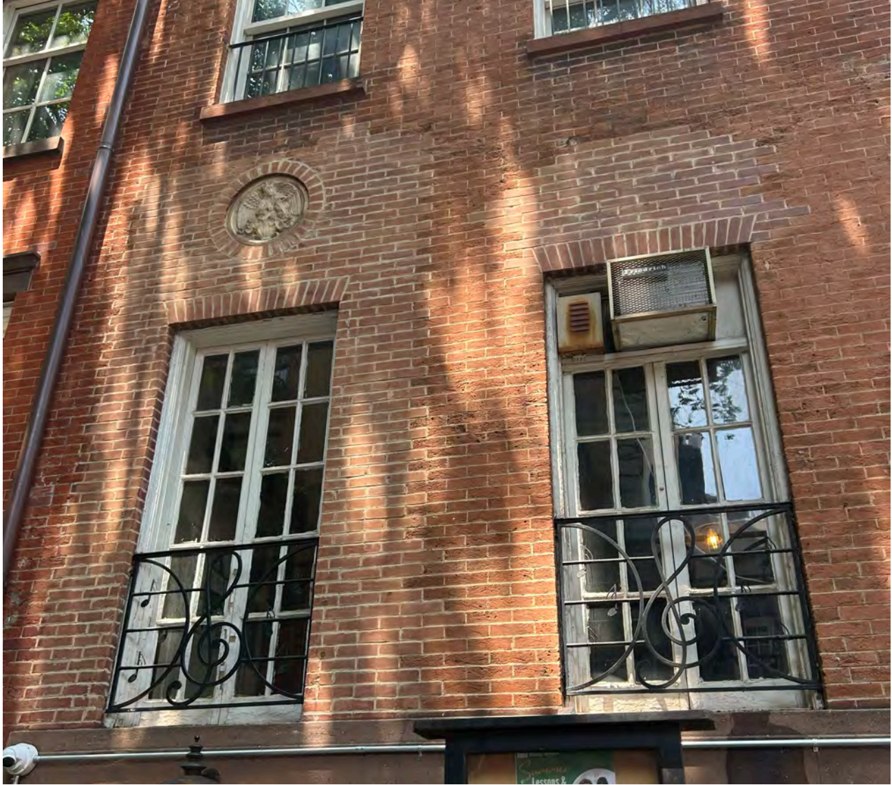
PARLOR FLOOR WINDOW WITH MEDALLION AND TREBLE CLEF RAILING PHOTO SHOWING BRICK INFILL AT HISTORIC DOOR (LEFT) AND PARLOR WINDOW (RIGHT) OPENINGS
