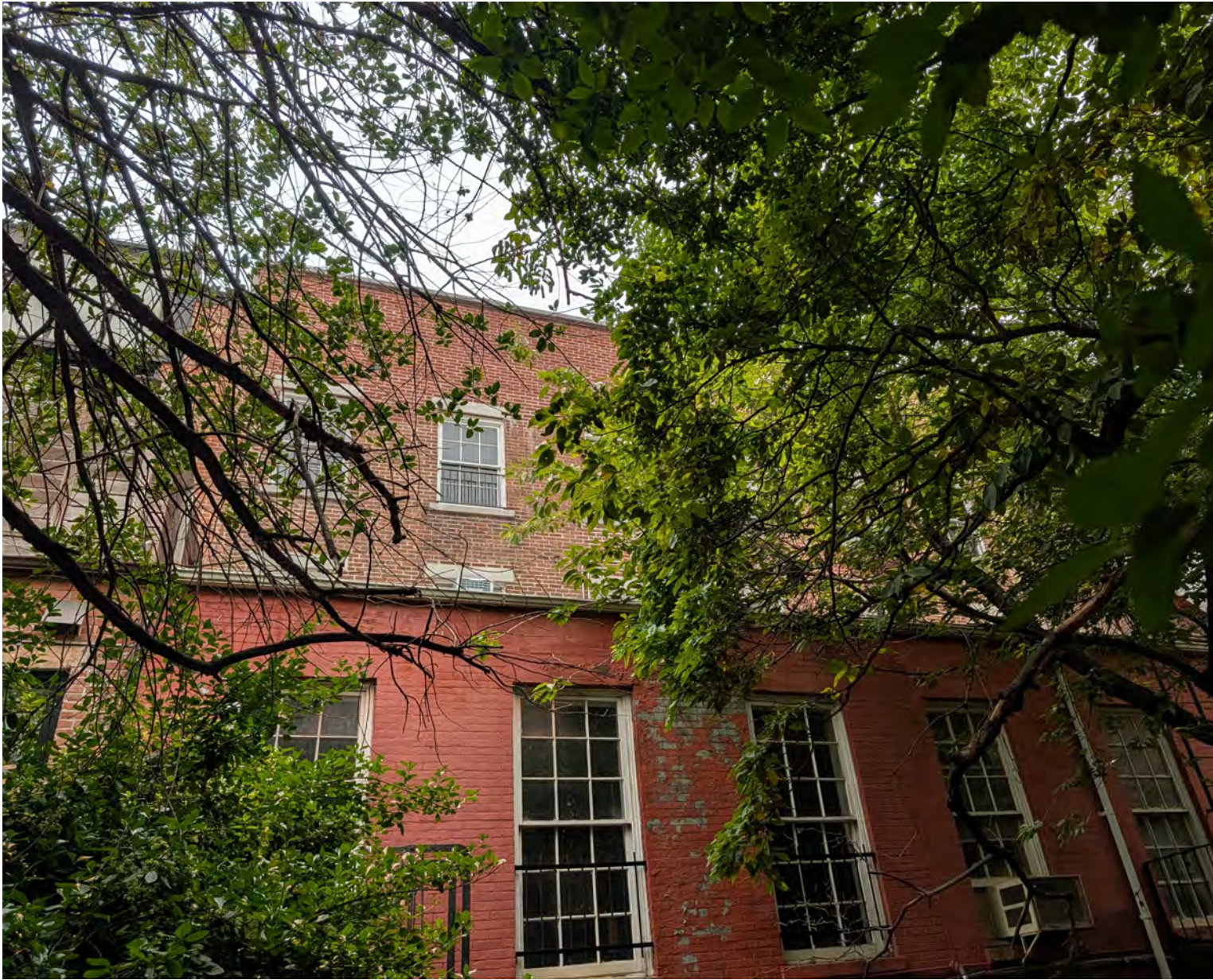
VIEW OF REAR FACADE VISIBLE BEYOND FOLIAGE & ABOVE EXISTING EXTENSION
