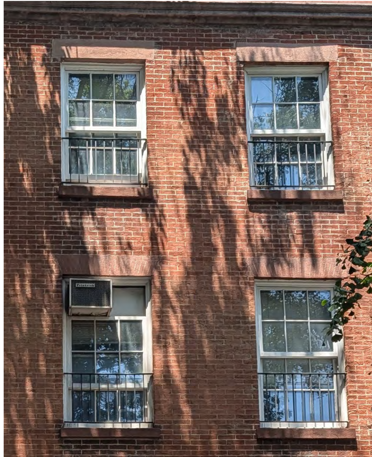
TYPICAL UPPER FLOOR WINDOWS AT NO. 46
