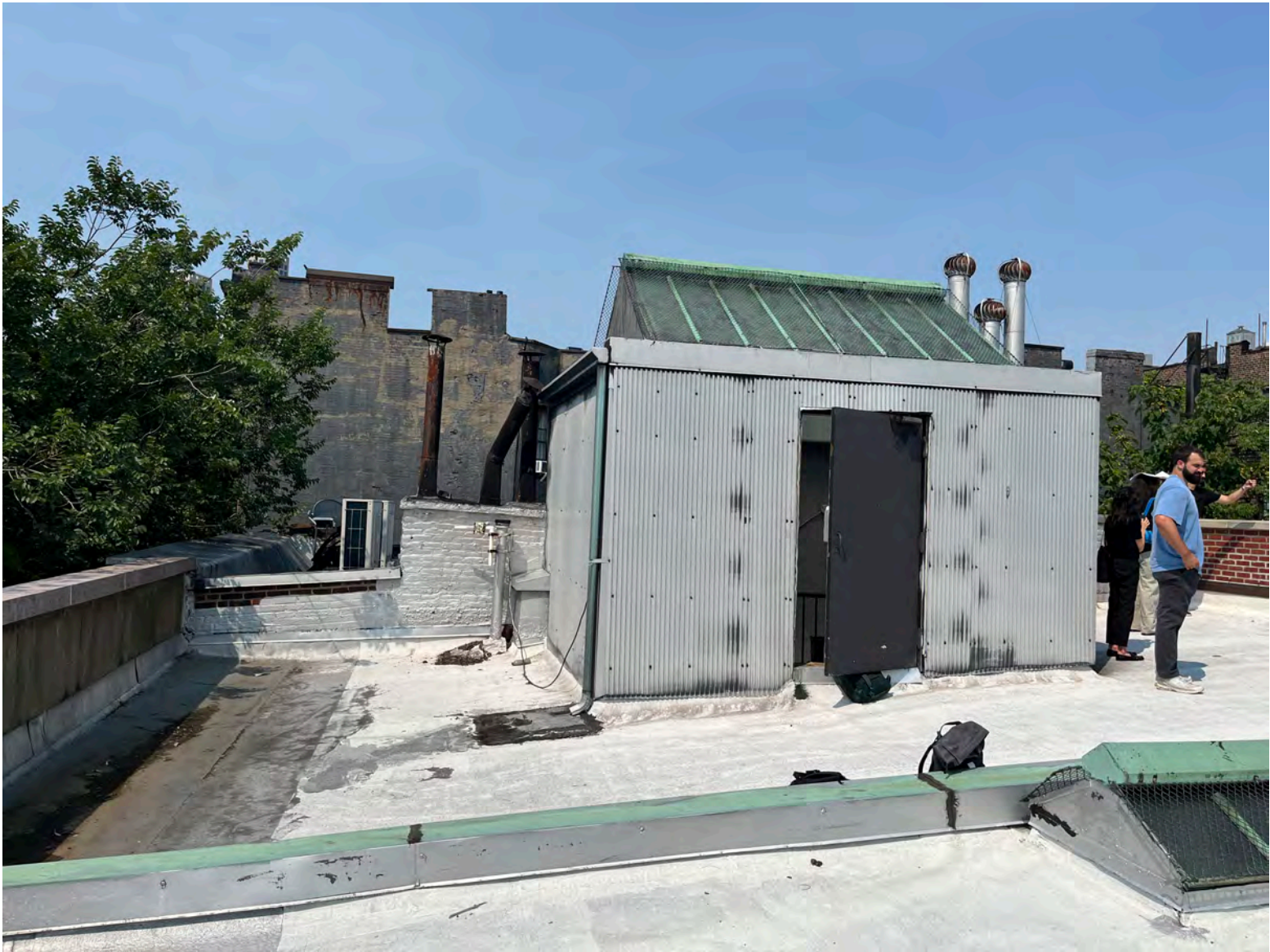
(B) VIEW OF ROOF AND EXISTING BULKHEAD LOOKING NORTHWEST
