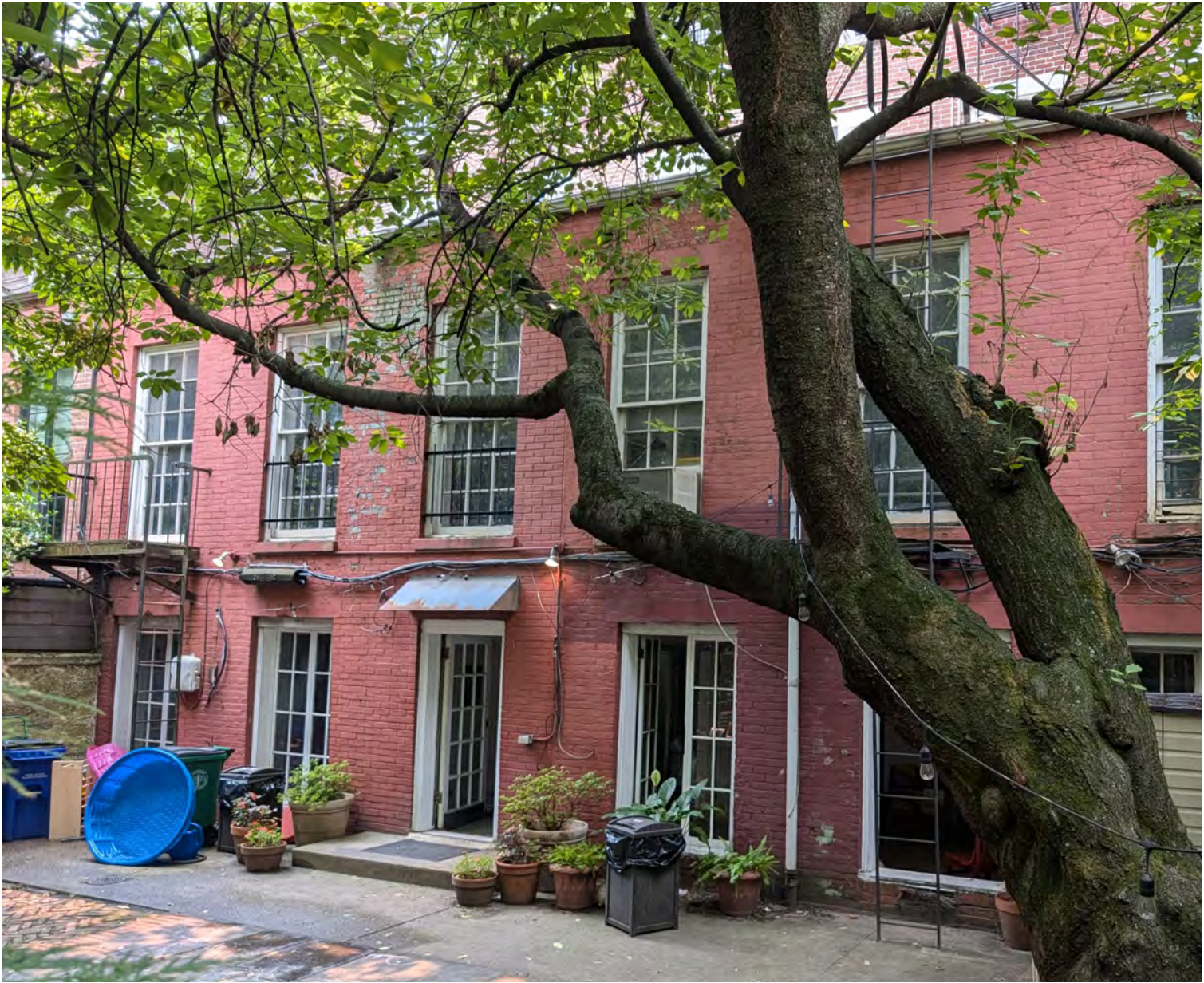
EXISTING REAR EXTENSION
