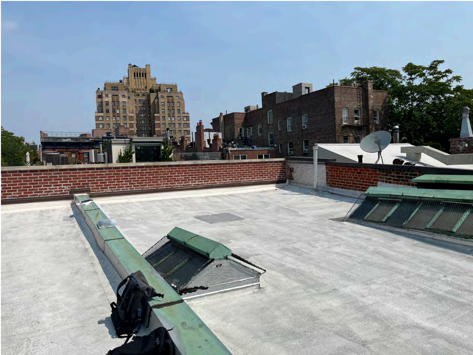
(A) VIEW OF ROOF LOOKING NORTHEAST
