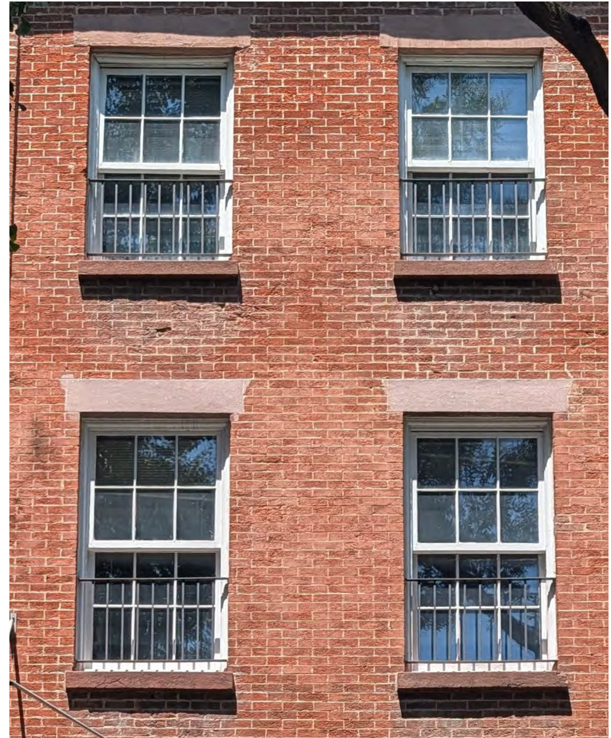
TYPICAL UPPER FLOOR WINDOWS AT NO. 44
