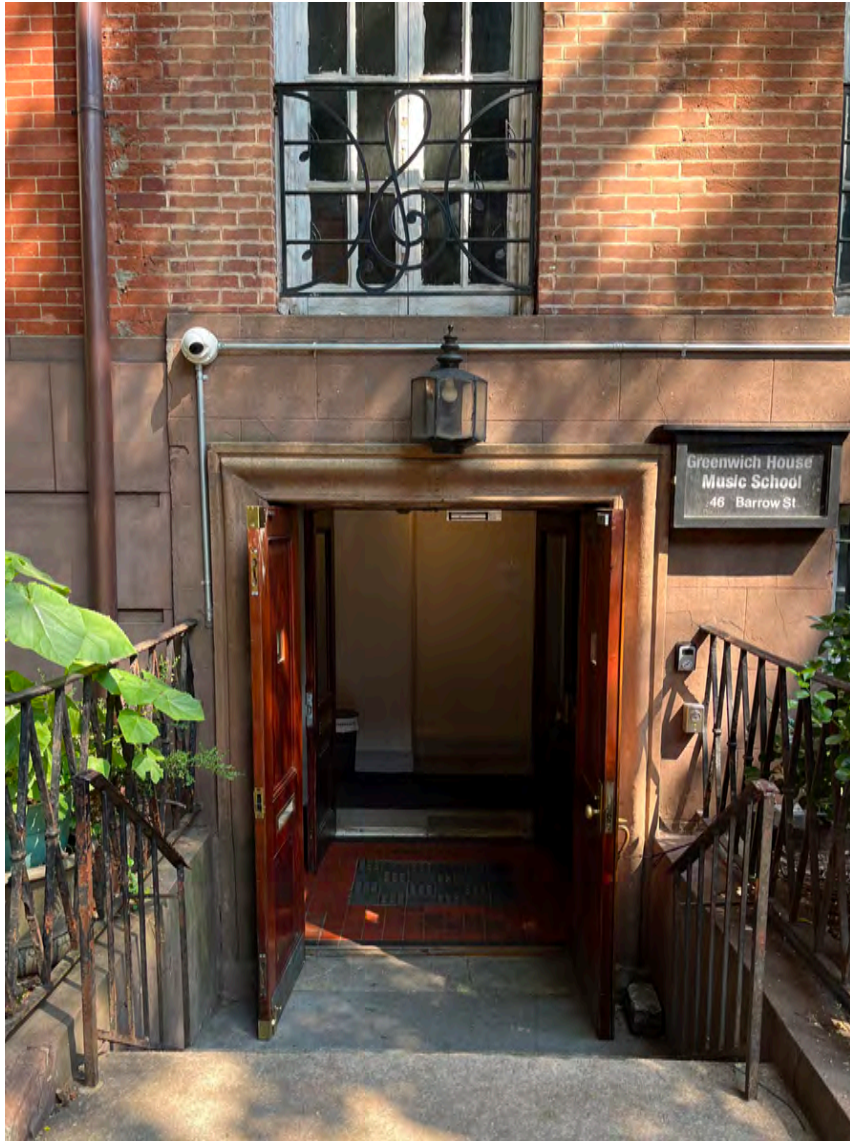
ENTRANCE AT 46 BARROW STREET
