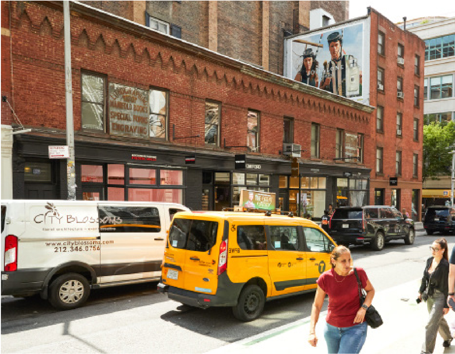
CURRENT CONDITION OF FACADE
