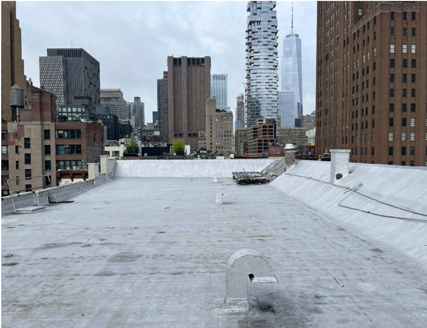
VIEW FROM ROOF VIEW G
