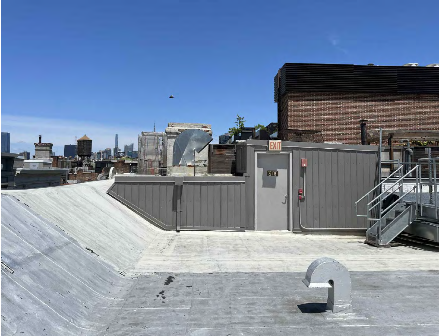
VIEW FROM ROOF VIEW H1
