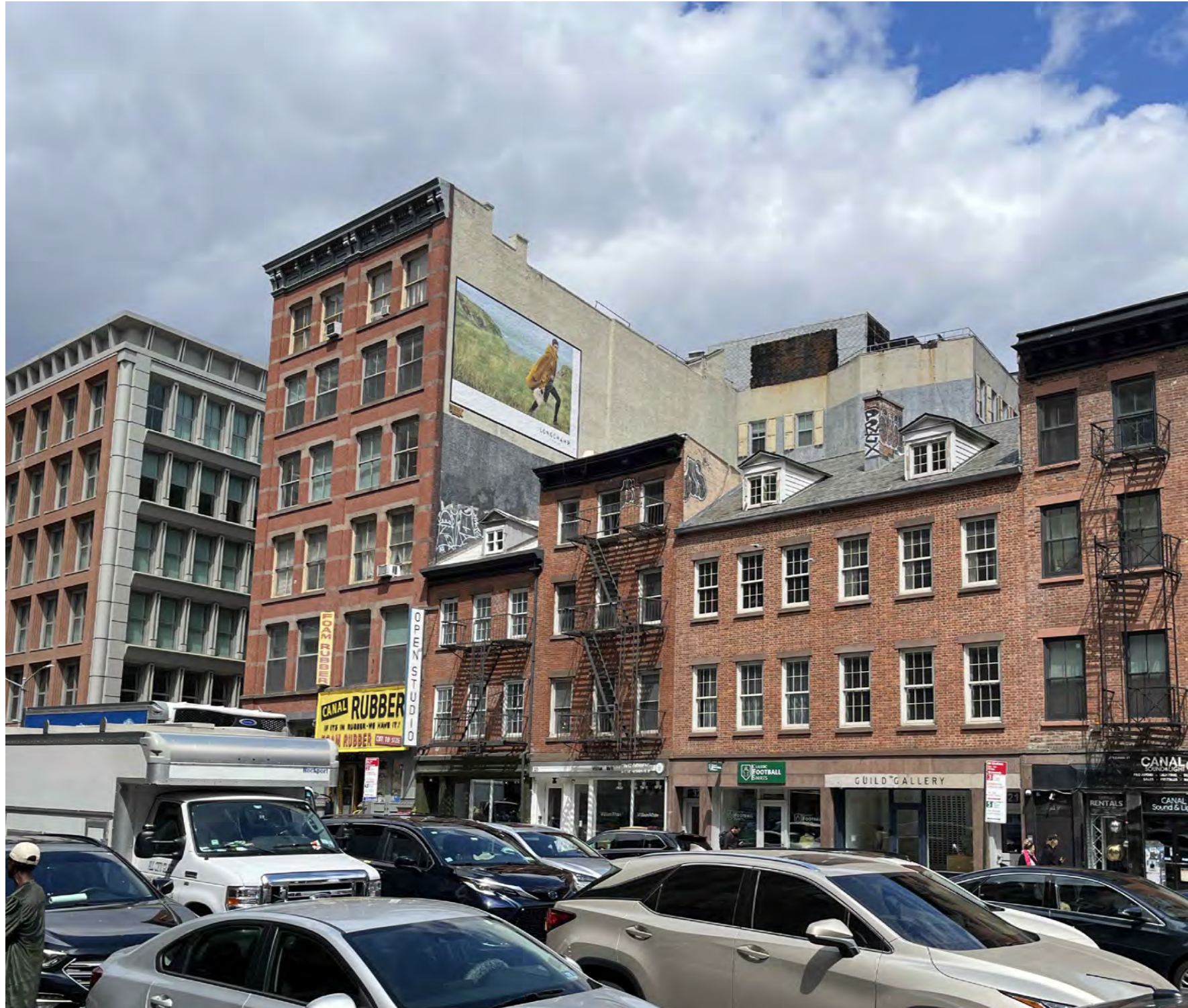
VIEW FROM CANAL STREET VIEW A1
