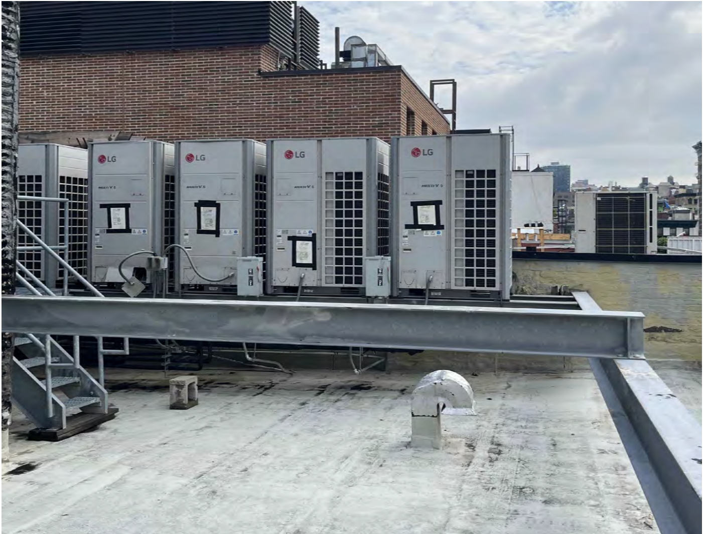
VIEW FROM ROOF VIEW K
