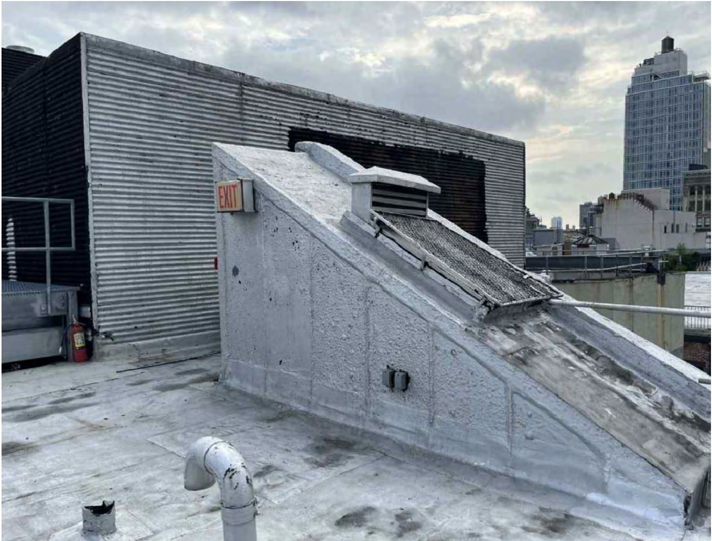
VIEW FROM ROOF VIEW I1
