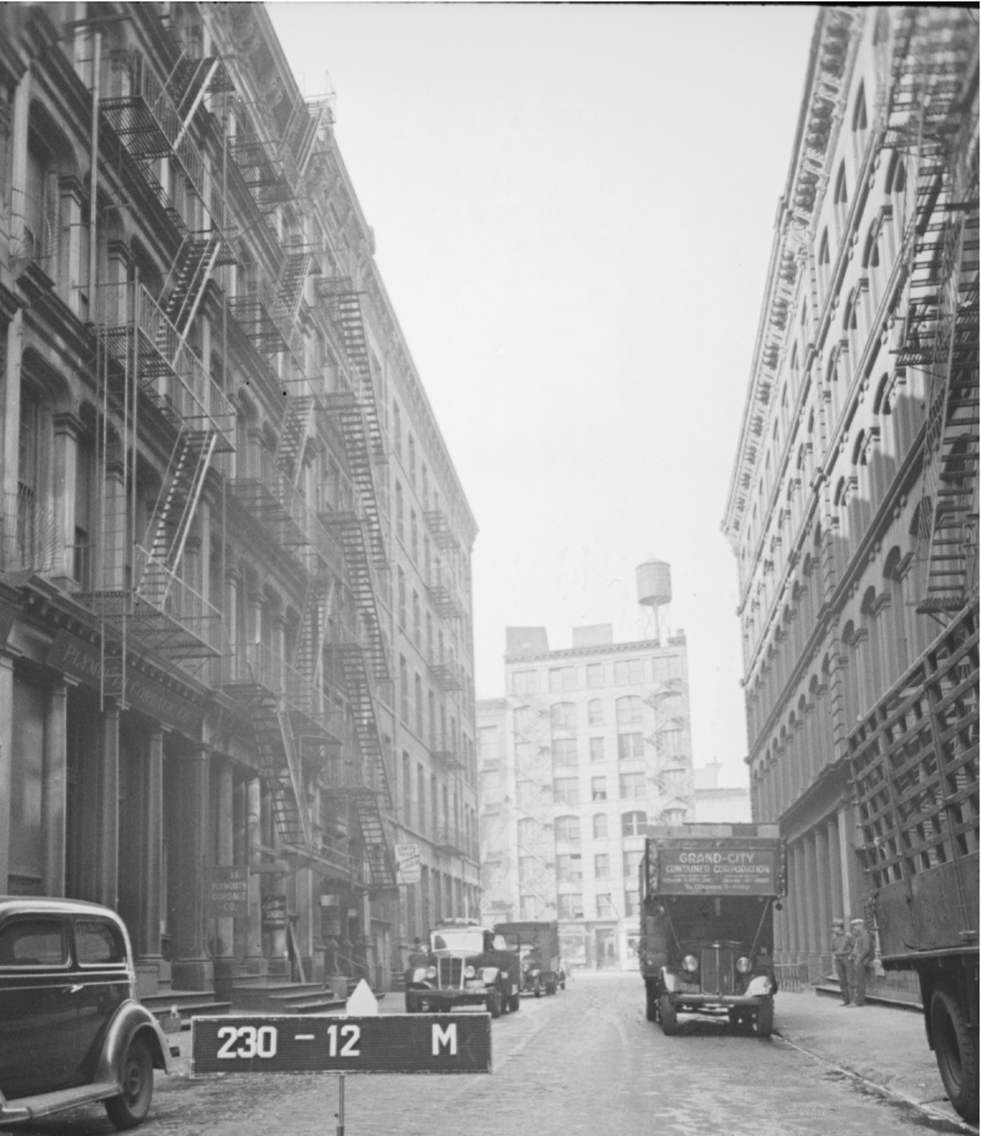
VIEW TO SOUTH ON GREENE STREET, 1940 (MUNICIPAL ARCHIVES)
