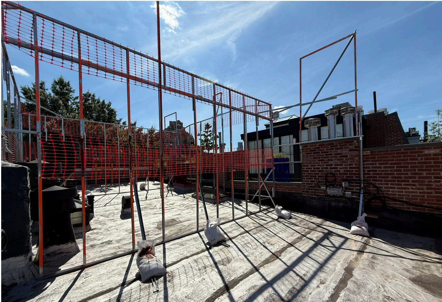
View to Southwest
