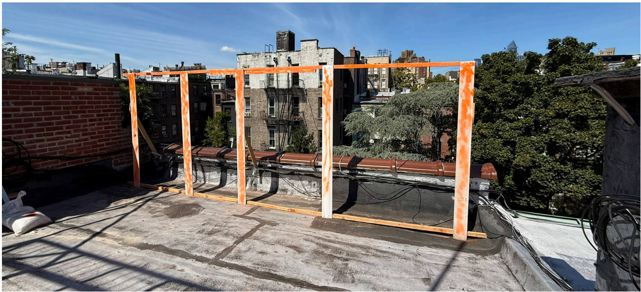
View of North Guardrail
