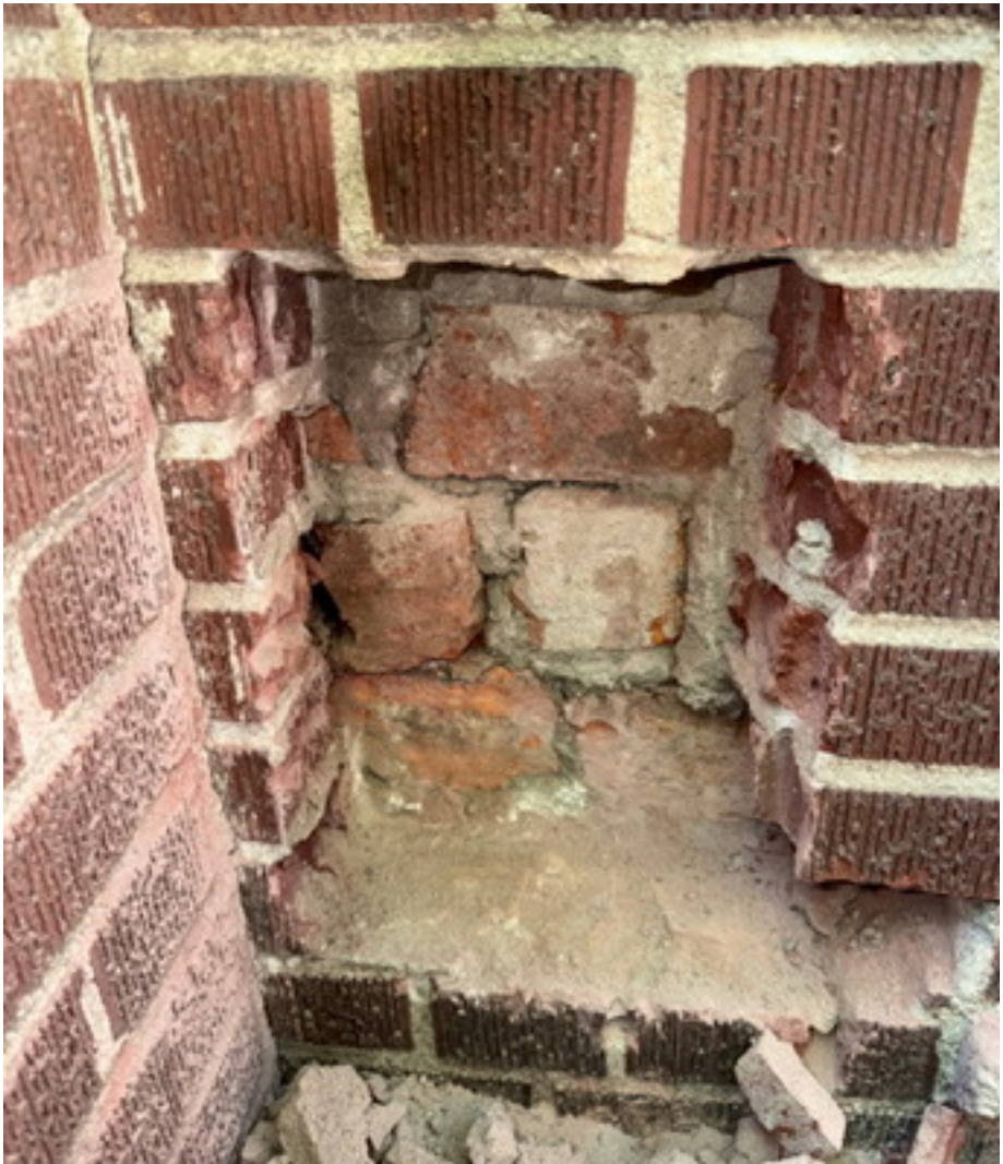
Basement Floor Probe from Exterior
