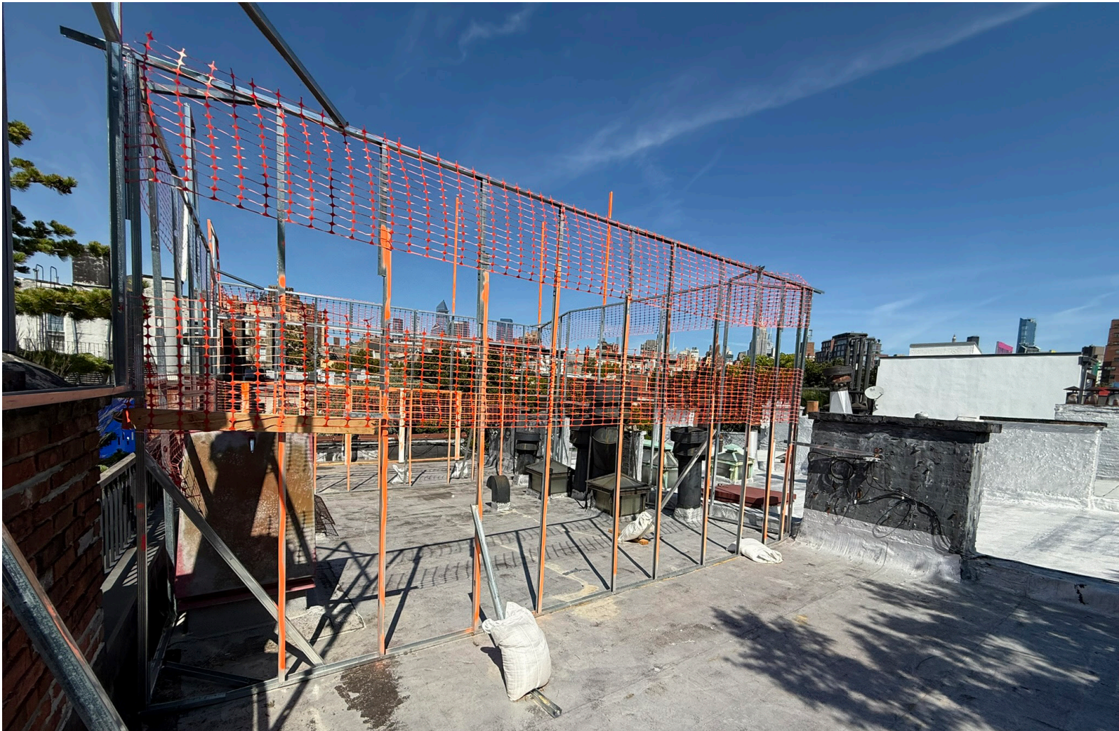
View to Northeast
