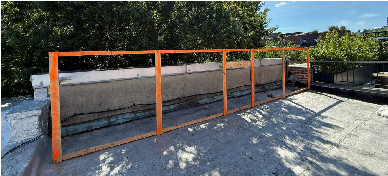
View of South Guardrail
