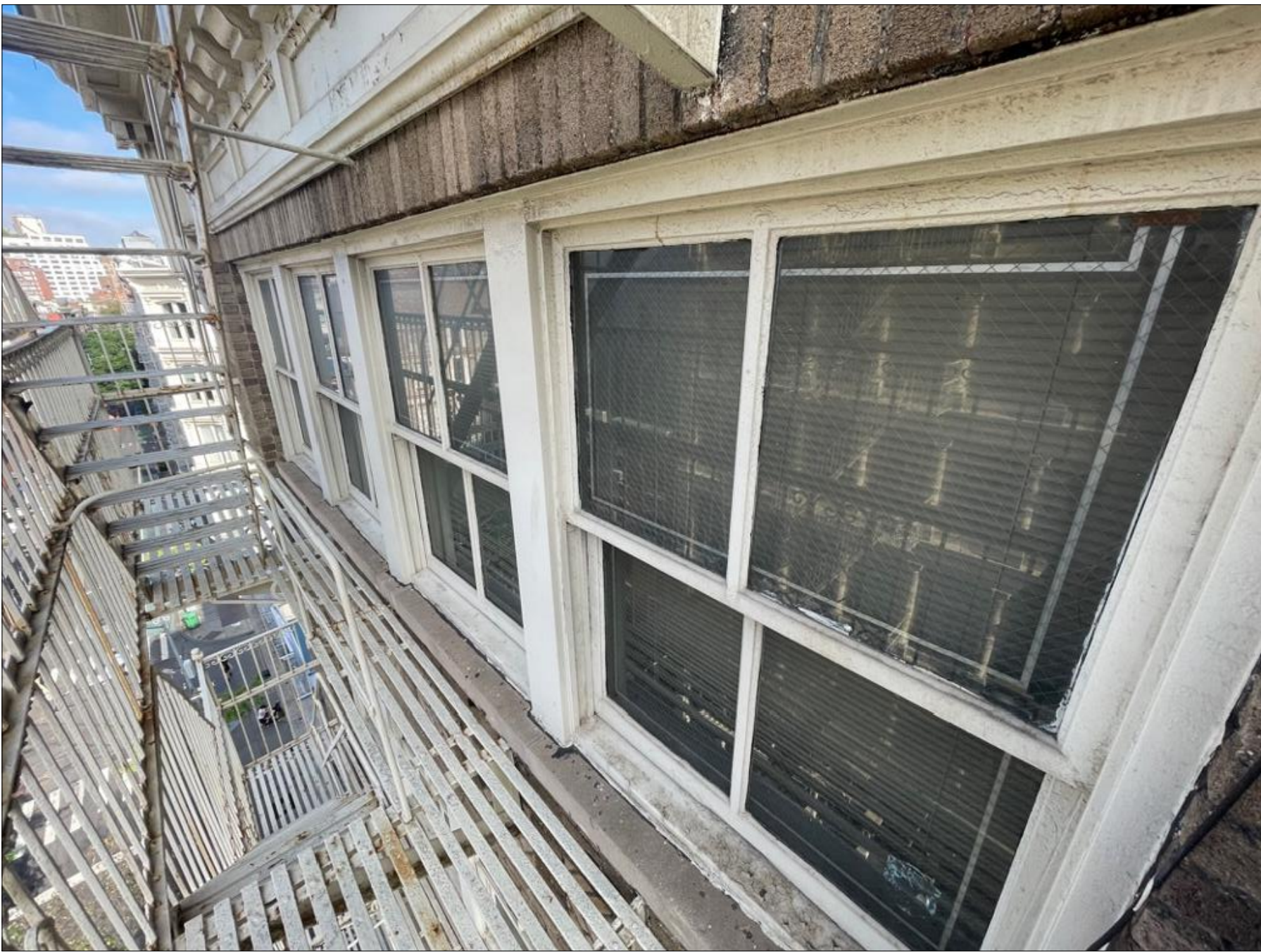
EXISTING WINDOW EXTERIOR VIEW
