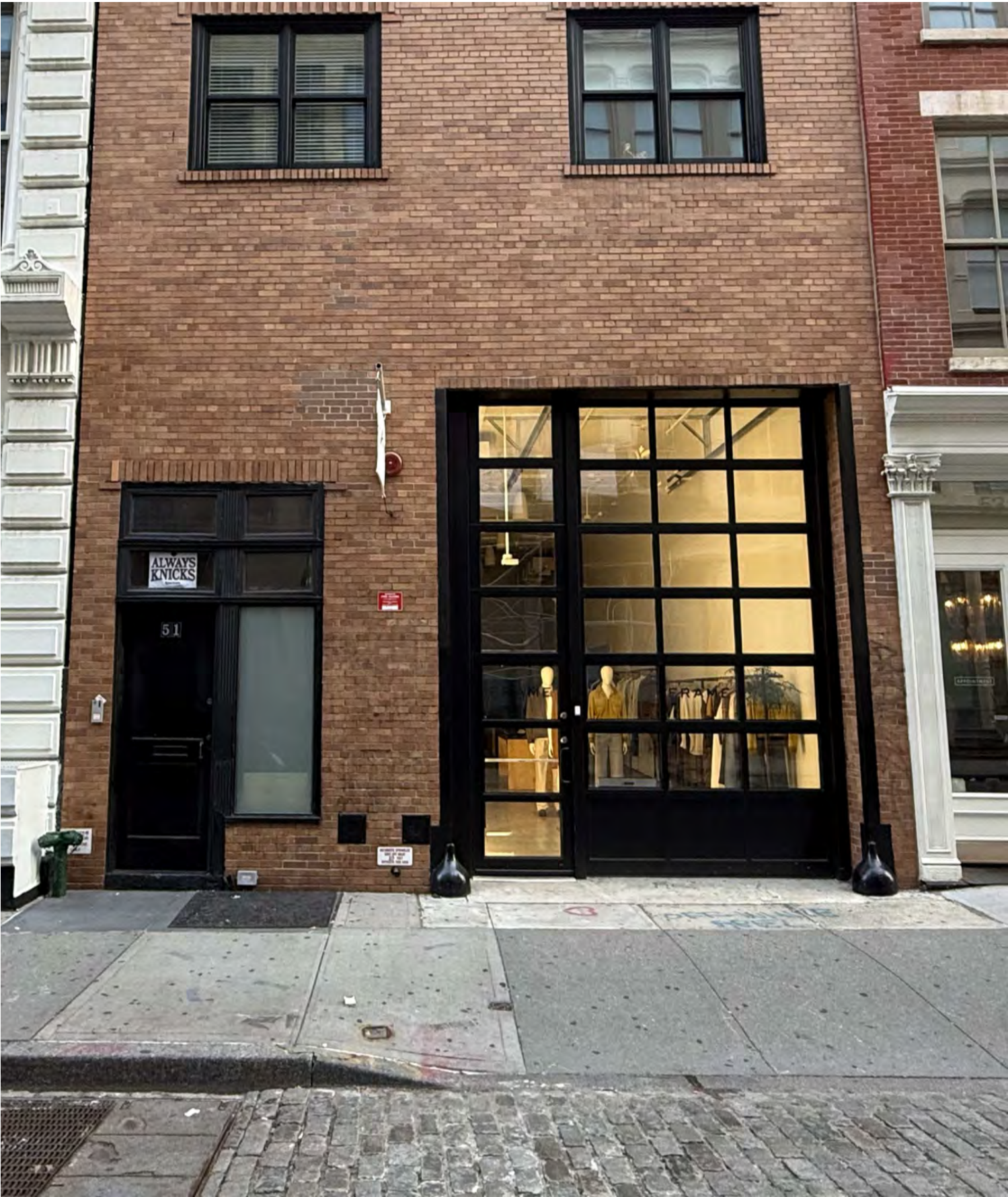
51 MERCER STREET - TODAY
