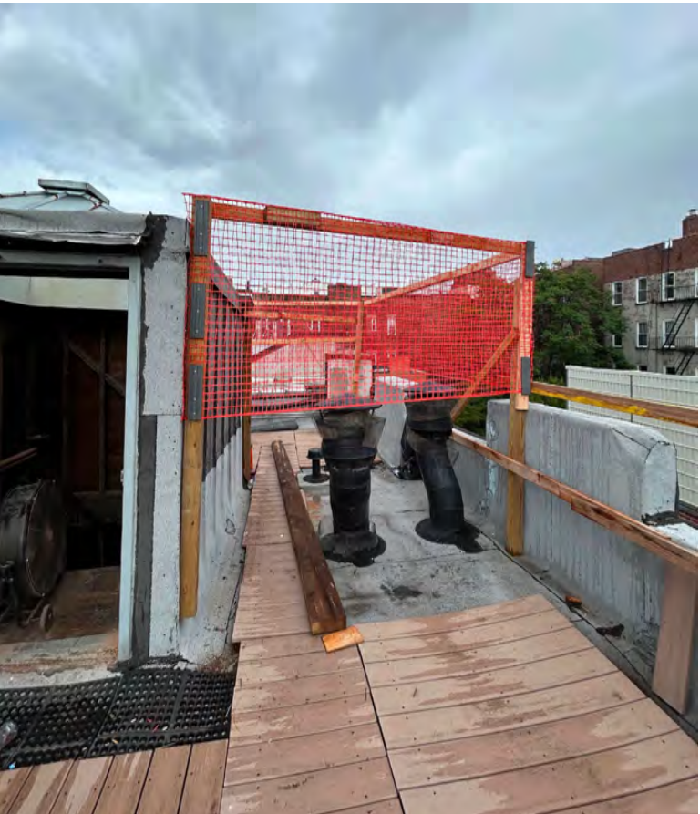
VIEW OF STAIR BULKHEAD MOCKUP FRONT
