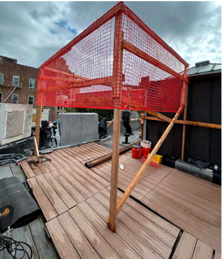
VIEW OF STAIR BULKHEAD MOCKUP REAR
