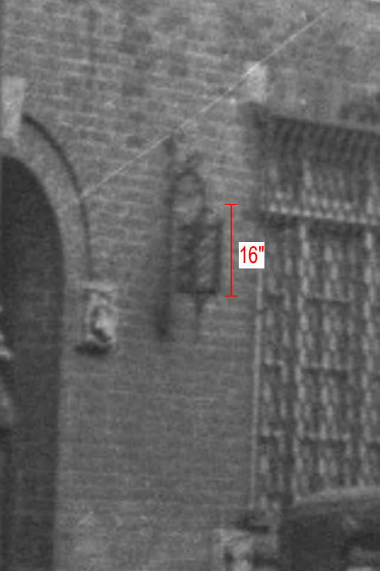
LIGHT FIXTURE HEIGHT ESTIMATED BASED ON BRICK COURSING
