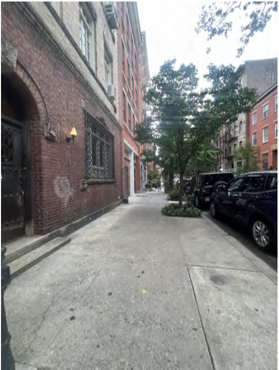
EXISTING SIDEWALK CONDITIONS - CONCRETE
