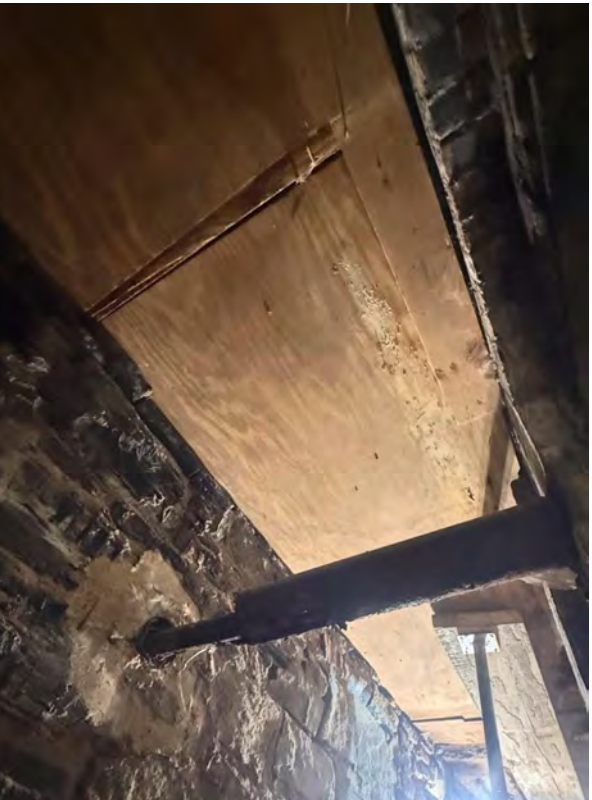
PHOTO #5 TAKEN AT THE INTERIOR OF THE VAULT FACING THE UNDERSIDE OF THE STREETSCAPE.
