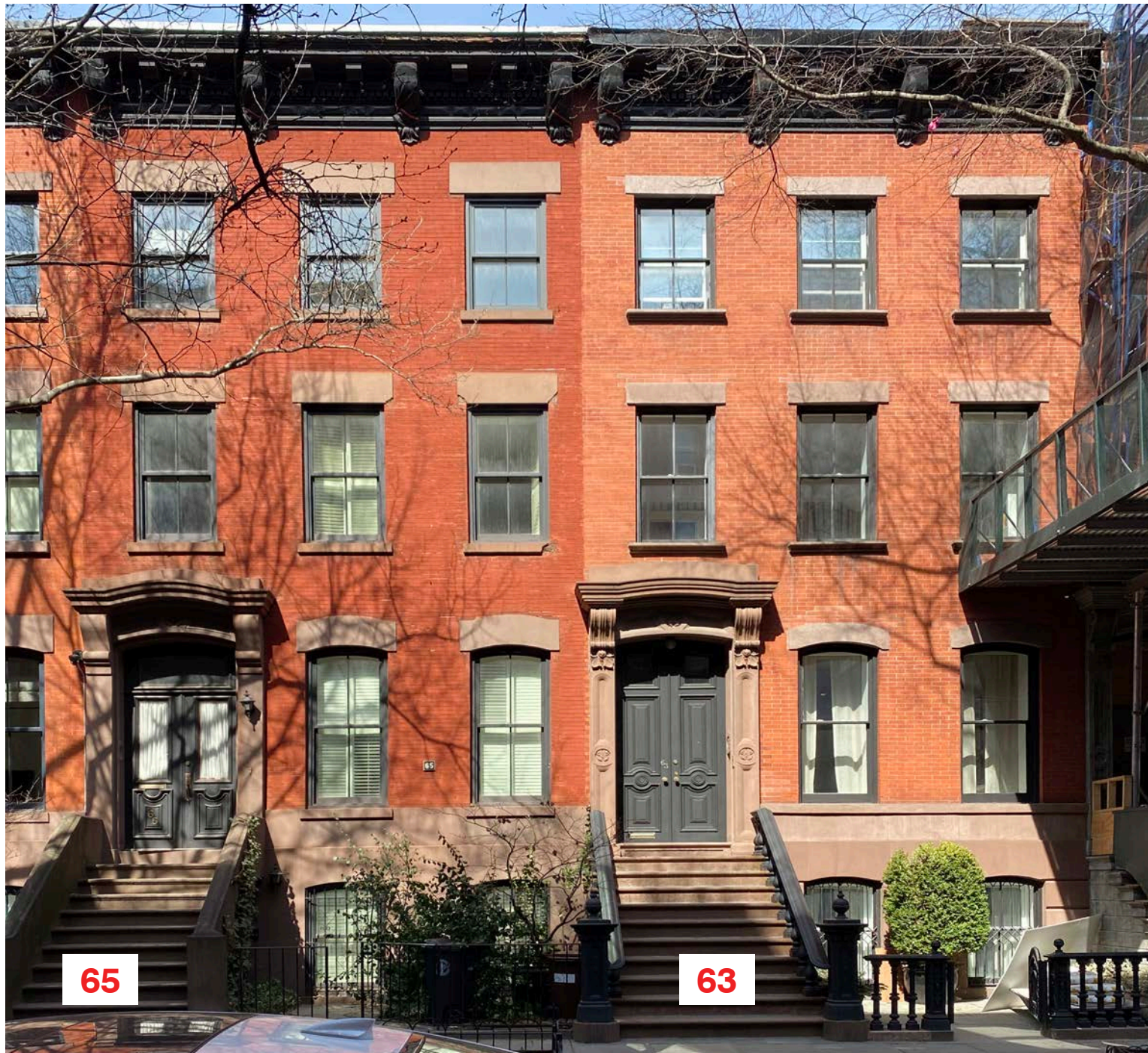
Existing Street Facade
