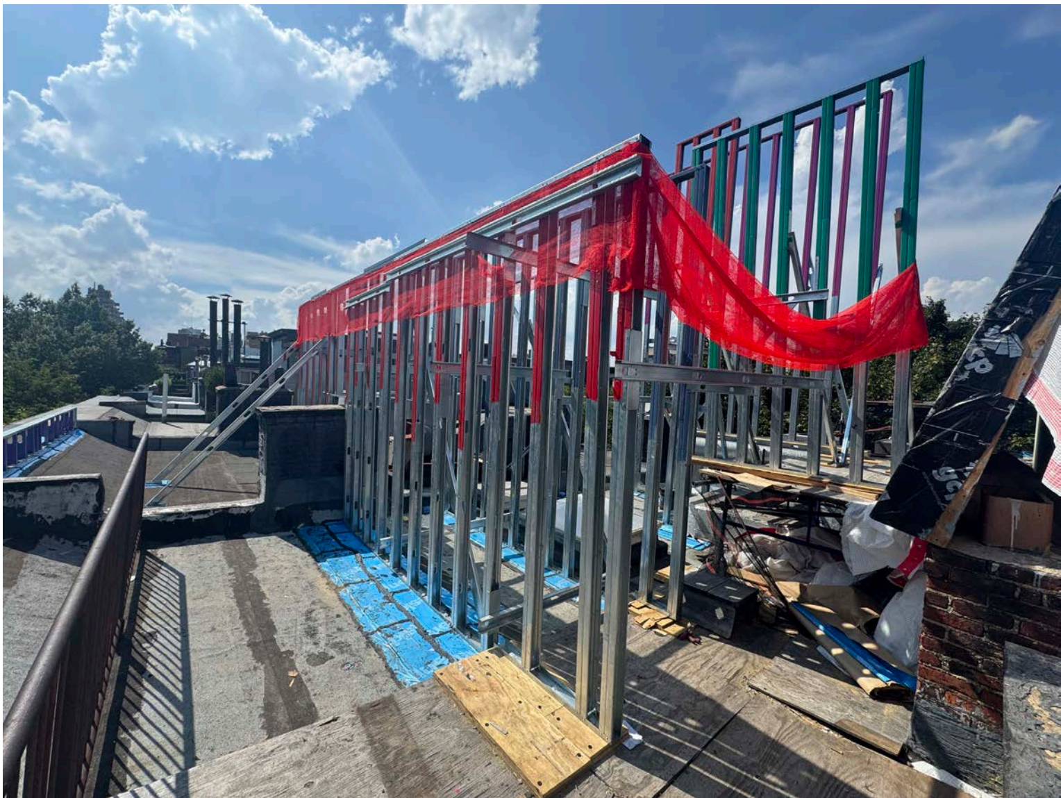
View of Mock-up Facing Northwest
