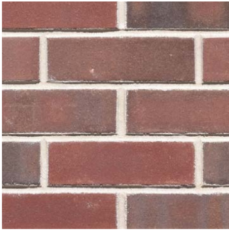
Atlantic Series Bristol (M) Type 2 (modular) Brick at rear facade extension
