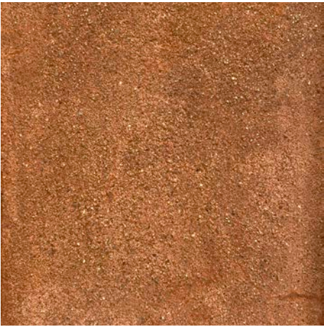
Brownstone New lintels and sills at rear facade
