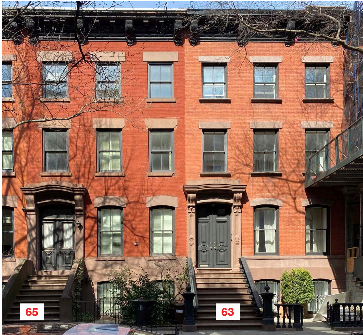
Existing Street Facade
