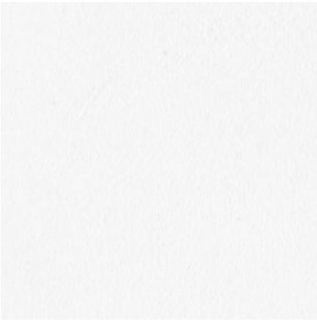
Plaster Penthouse roof soffit
