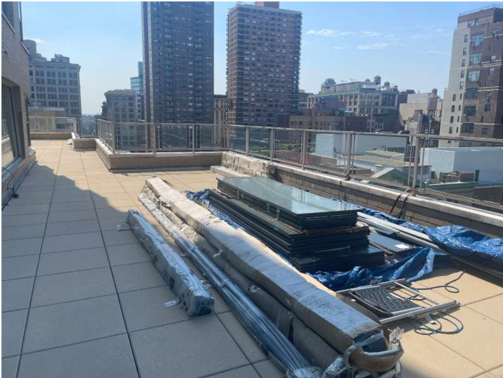
Replacement Glass Panels/Sliding Doors
