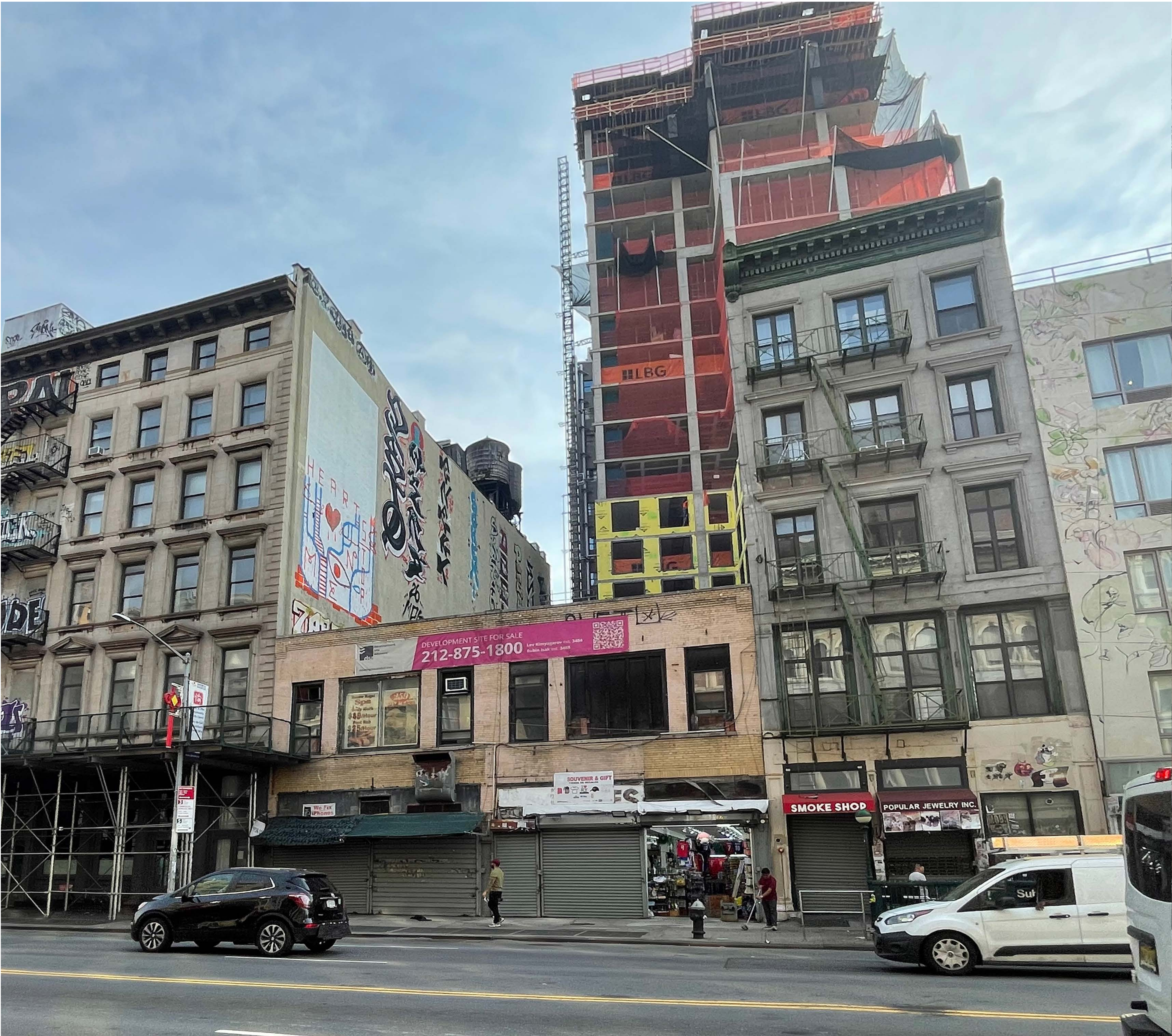
EXISTING SITE CONDITIONS
