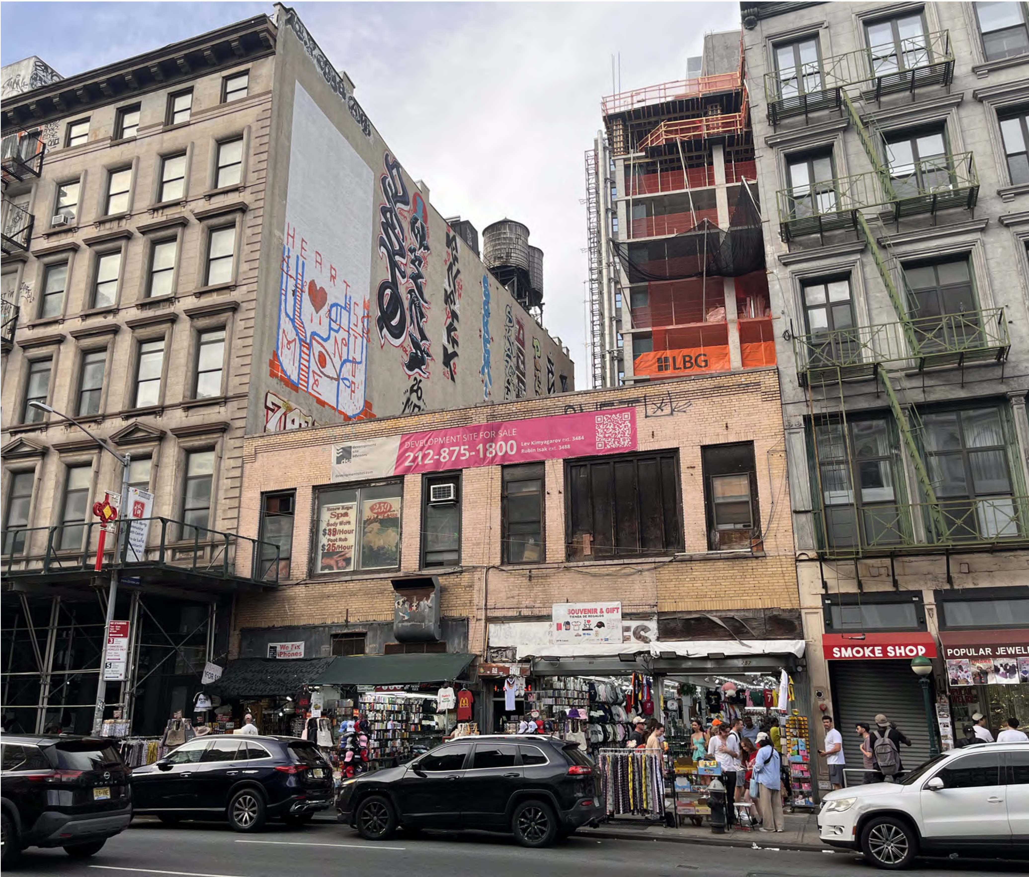
EXISTING SITE CONDITIONS
