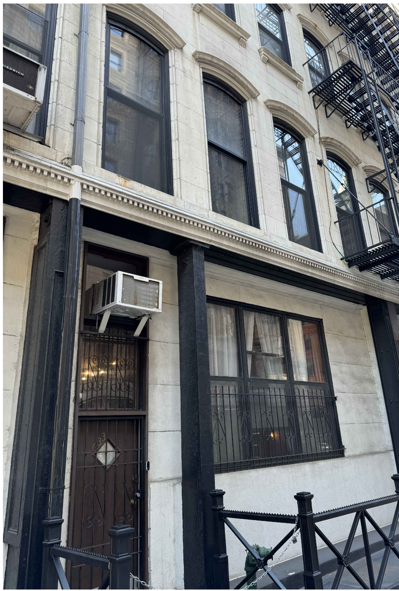
01 633 BROADWAY EX'G FRONT FACADE AT GROUND LEVEL N.T.S.
