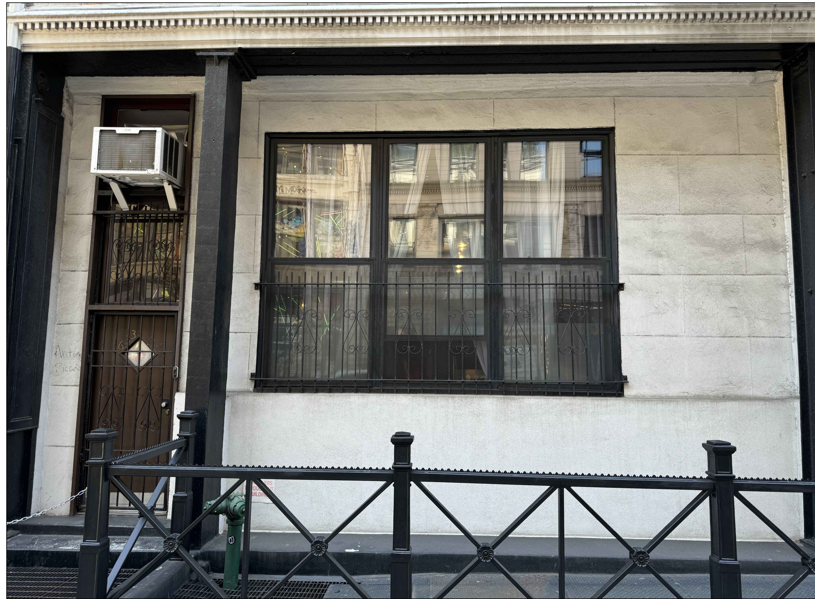
06 633 BROADWAY EXISTING FRONT FACADE AT GROUND LEVEL N.T.S.
