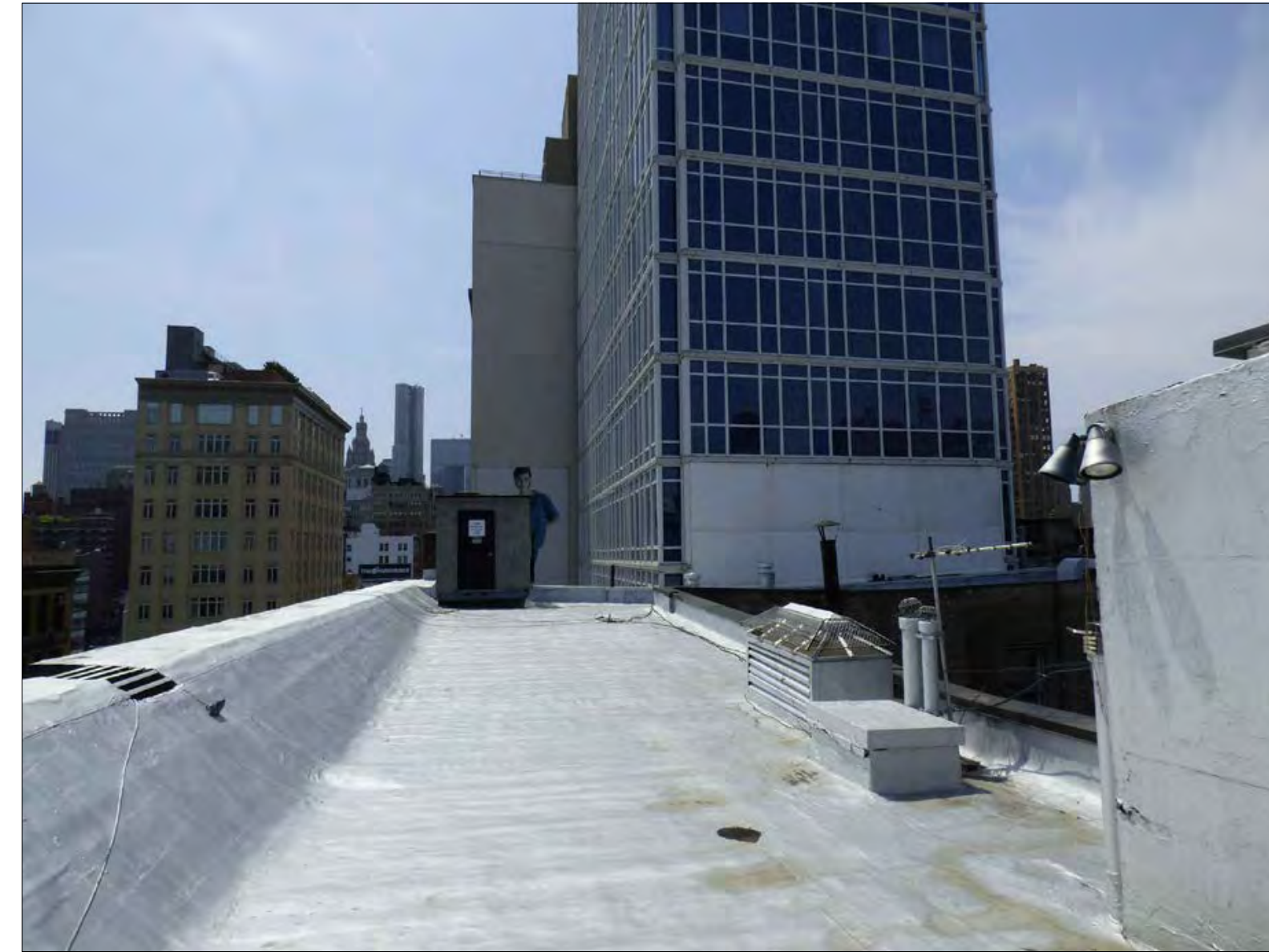
2 - ROOF-EXISTING CONDITIONS LOOKING SOUTH
