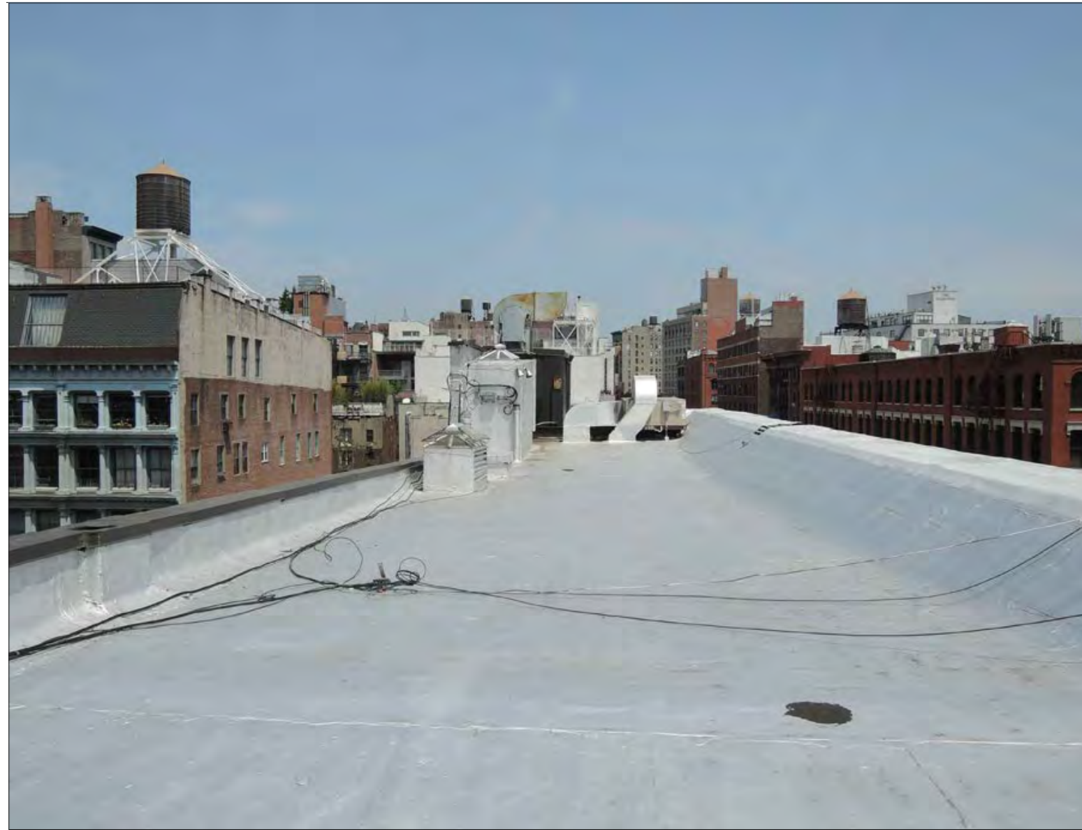
3 - ROOF-EXISTING CONDITIONS LOOKING NORTH
