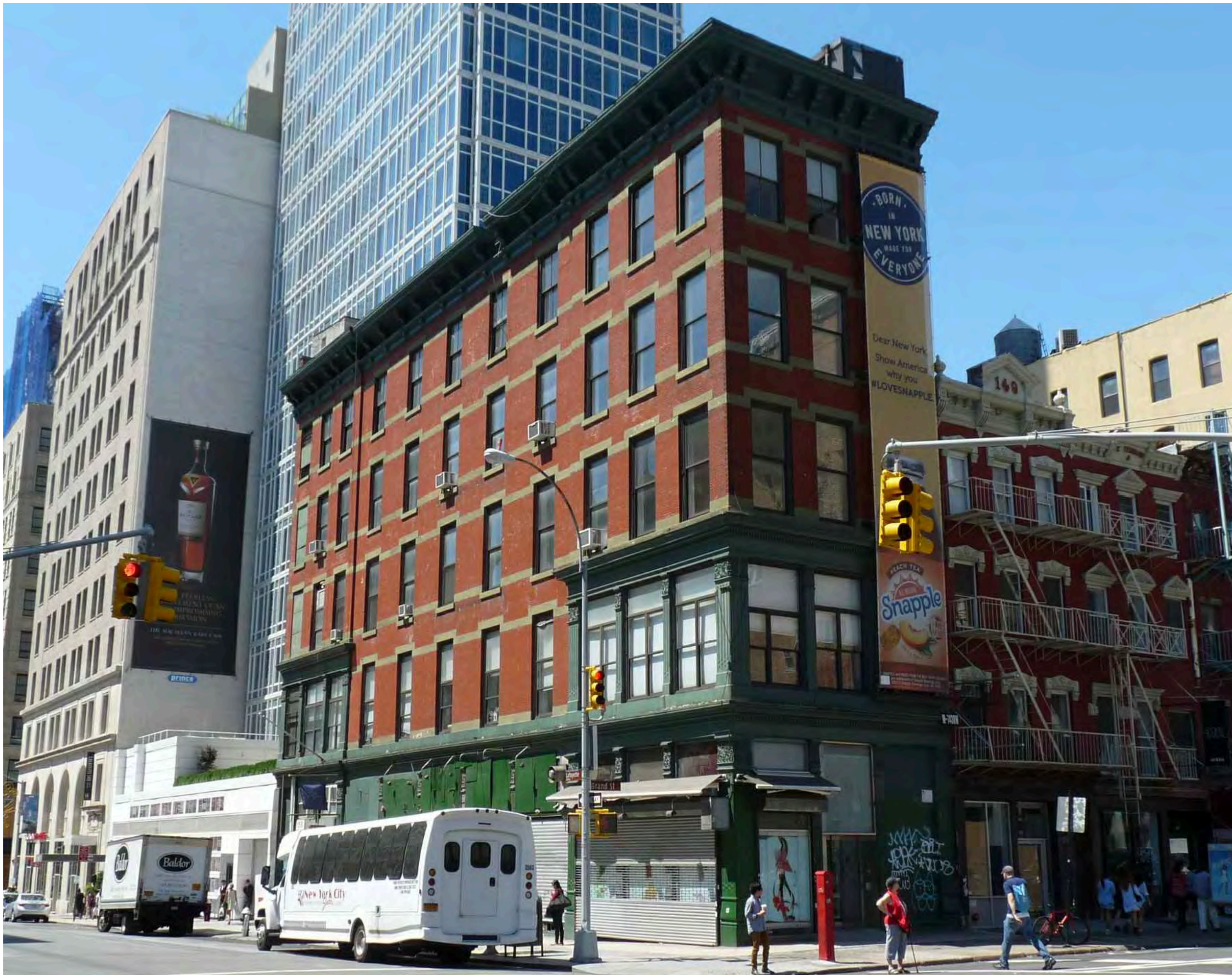
LAFAYETTE STREET CONDITIONS, 2016
