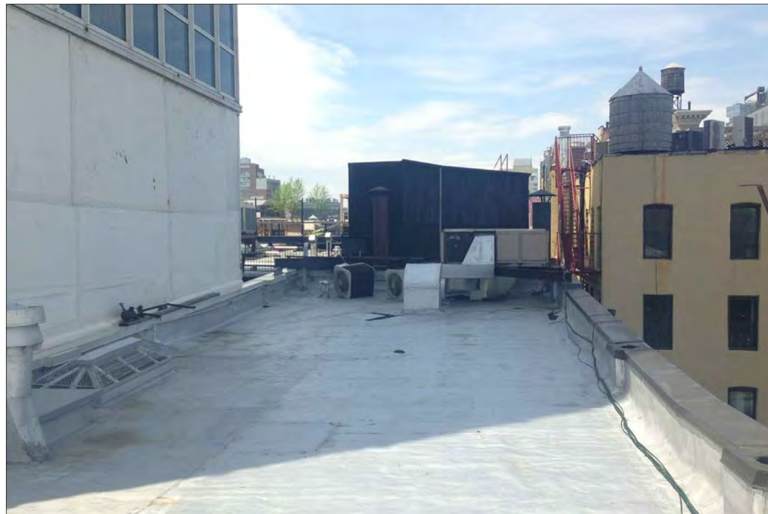
1 - ROOF - EXISTING CONDITIONS LOOKING WEST
