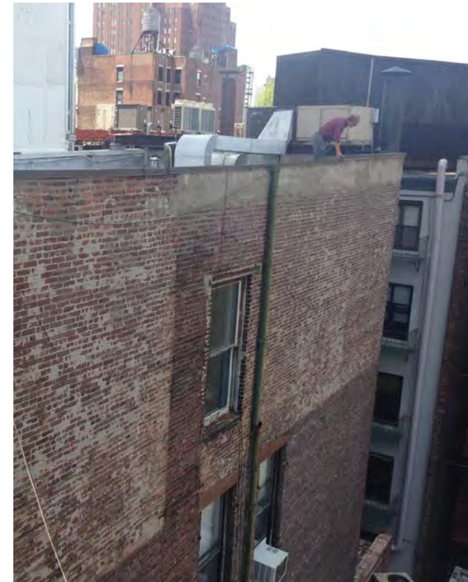
South inner wall
