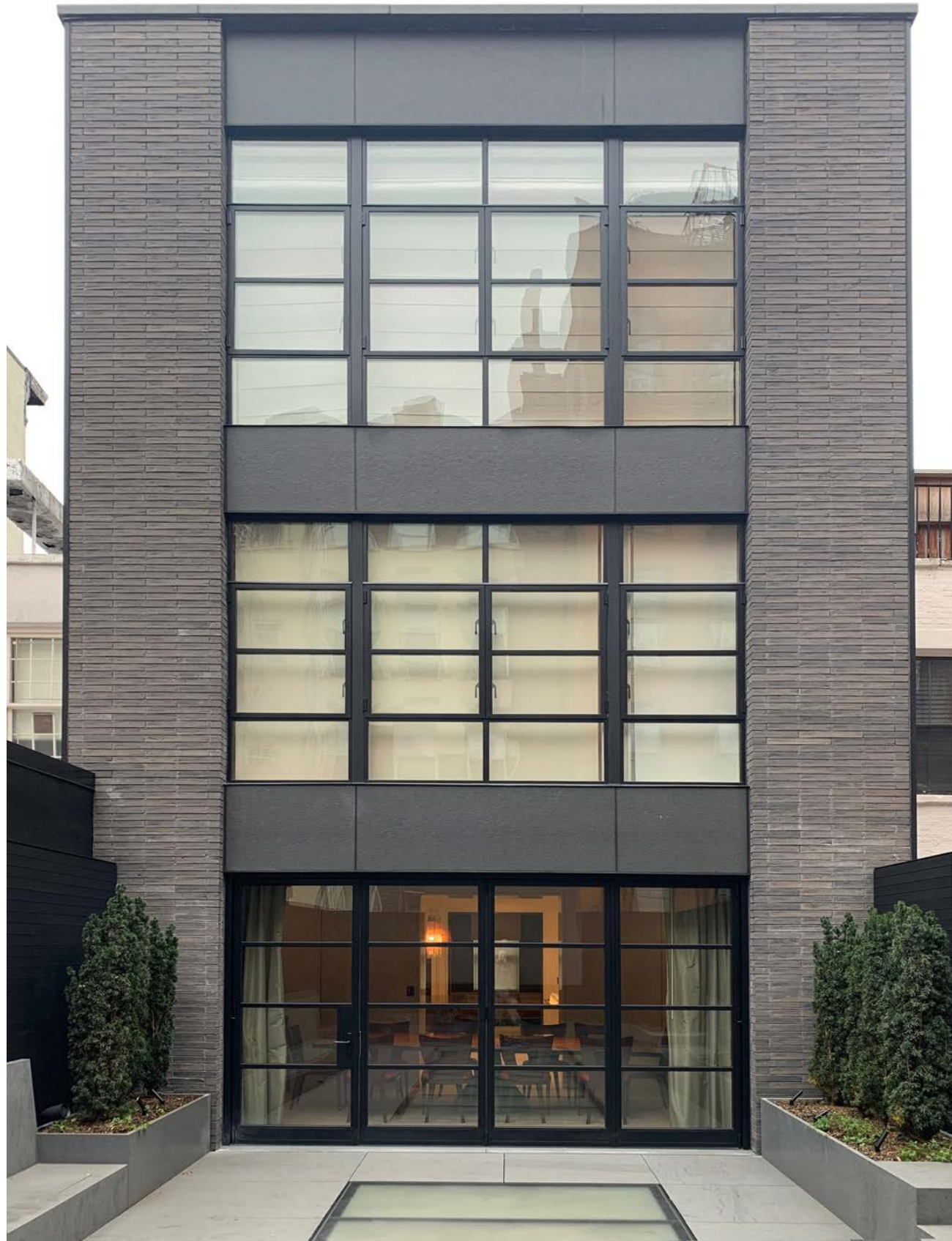
46 MACDOUGAL ST REAR FACADE
