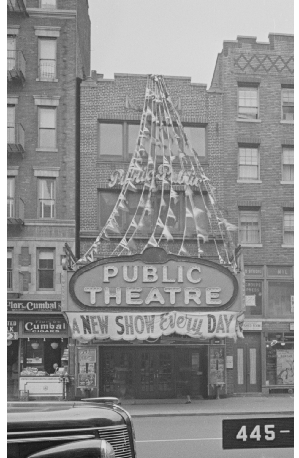
Public Theatre, 66 Second Avenue (H. Craig Severance, architect, David Oltarsh, consulting engineer, 1927)
