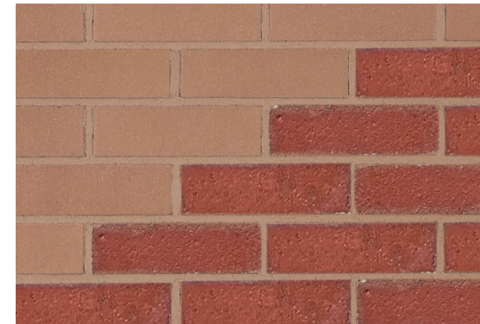
Brick - At Lot Line & Rear Wall
