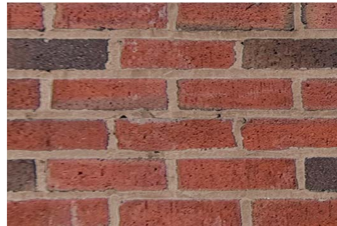
Brick - At Street Facade
