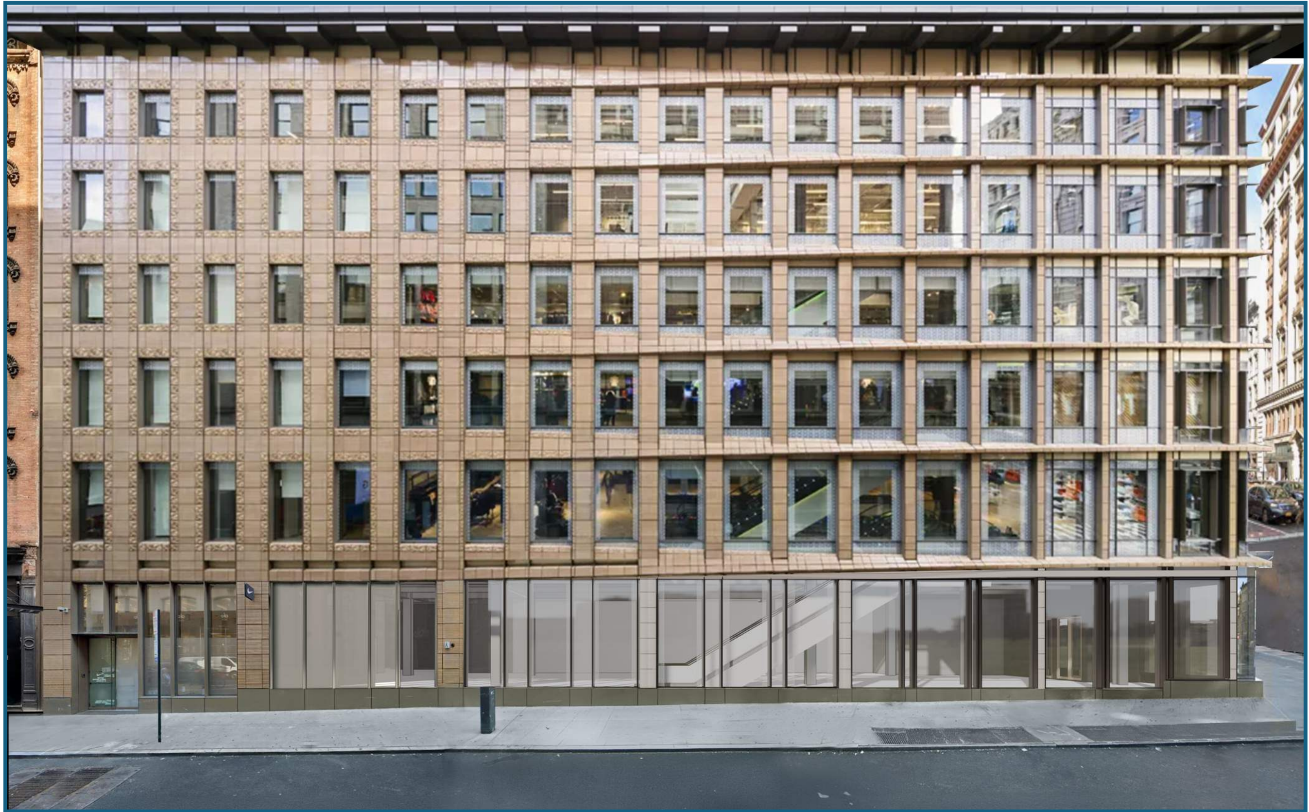
EXISTING FAÇADE ON SPRING STREET
