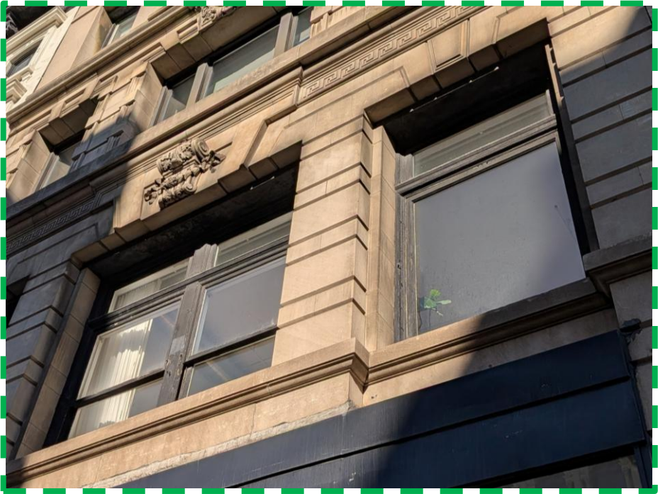
491 Broadway, east elevation second floor windows, April 2026. (J. Peu-Duvallon)
