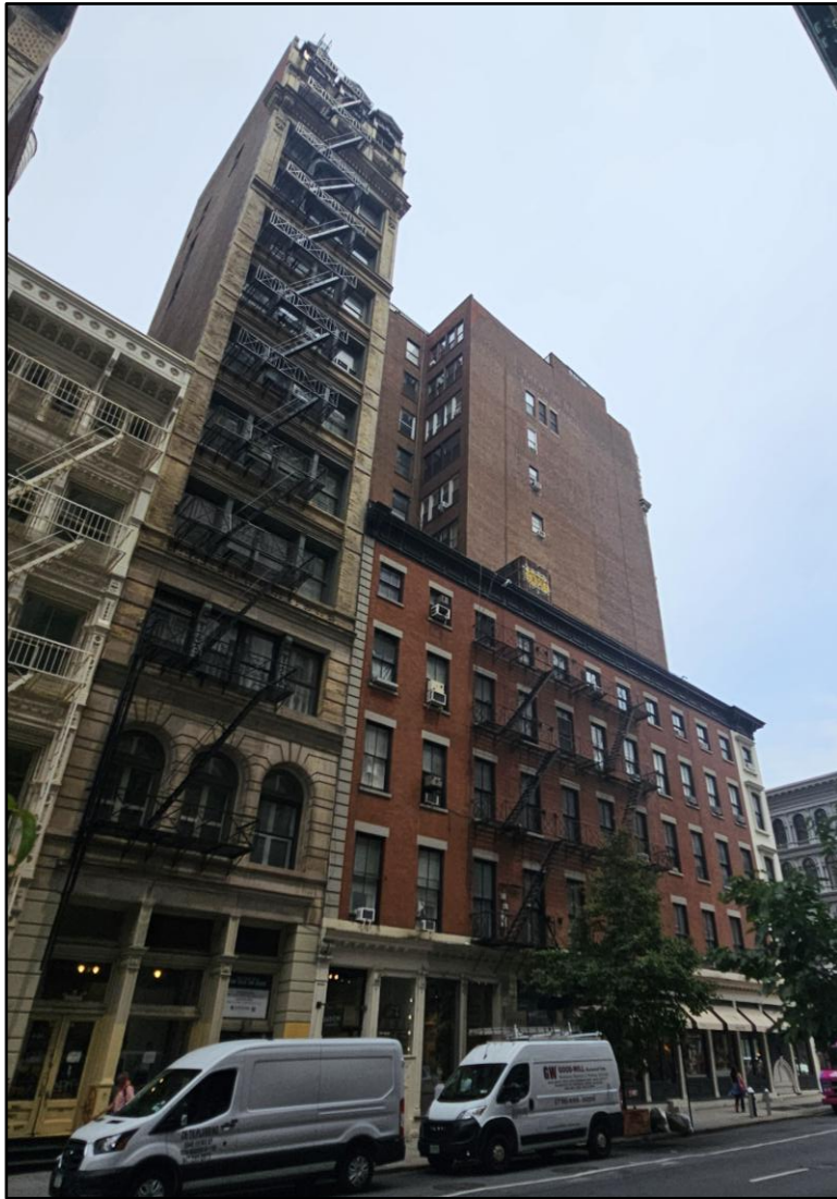
Previous windows at west lot line return wall. Summer 2025. (Metamechanics)
