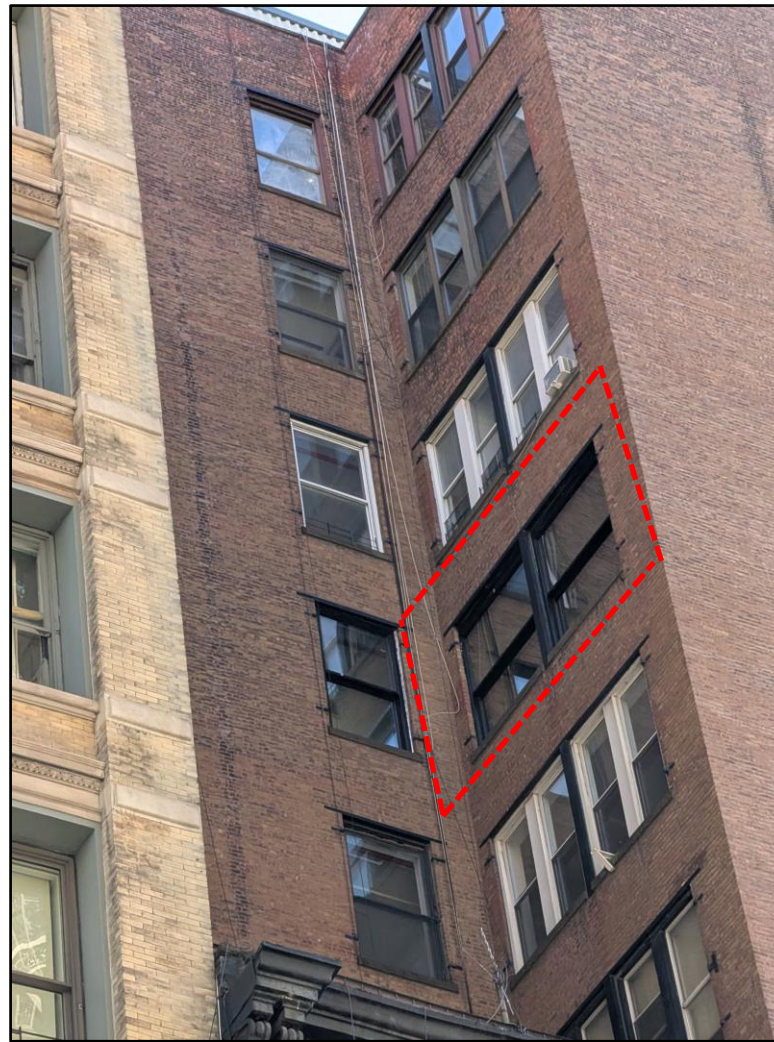
Windows replaced at west lot line return wall, zoomed in. April 2026. (J. Peu-Duvallon)
