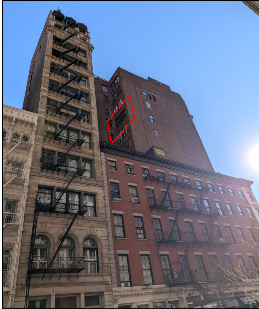
Windows replaced at west lot line return wall. April 2026. (J. Peu-Duvallon)
