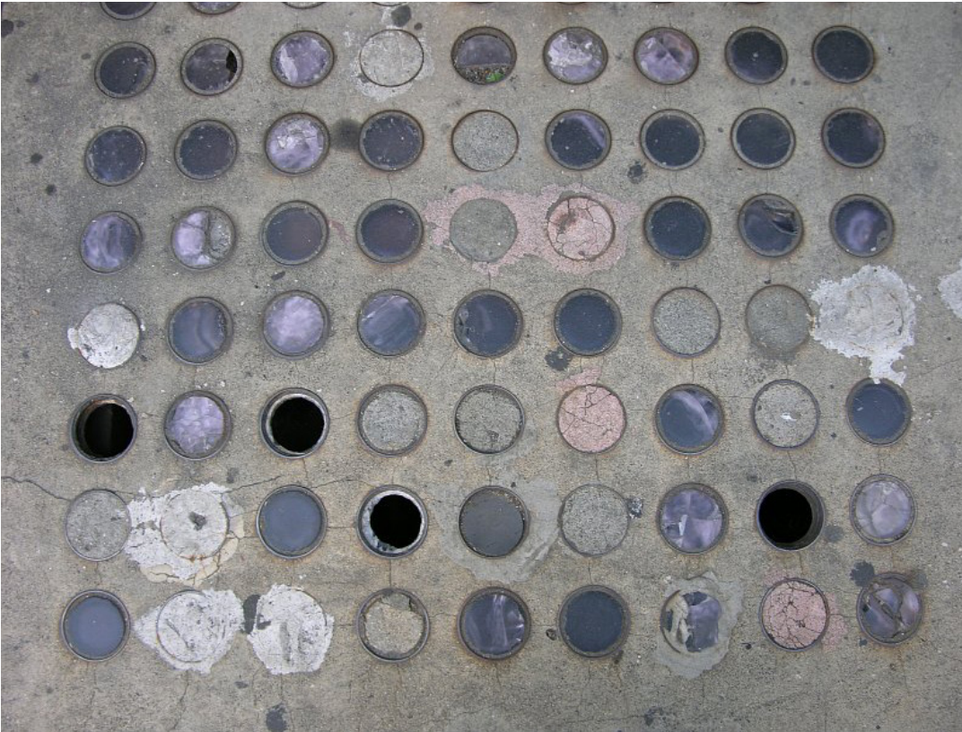
Typical concrete vault lights
