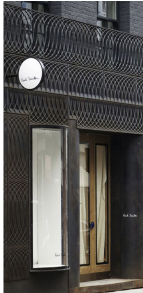
Facade of Paul Smith Store in London
