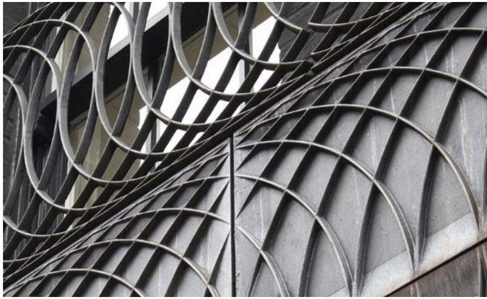
Facade of Paul Smith Store in London
