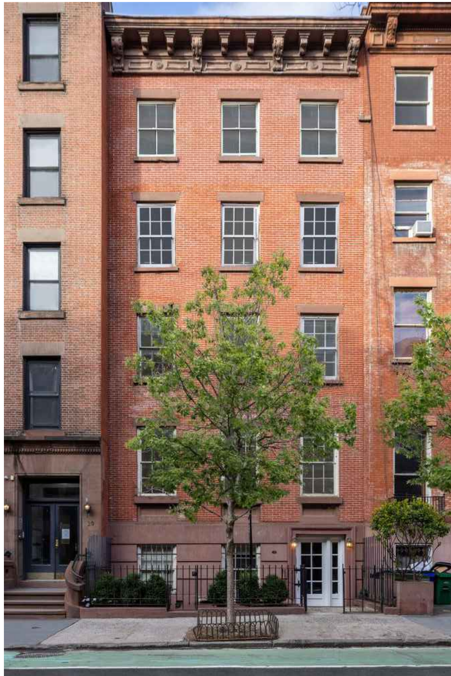
23 WEST 12TH STREET EXISTING PHOTOS (FRONT FACADE)
