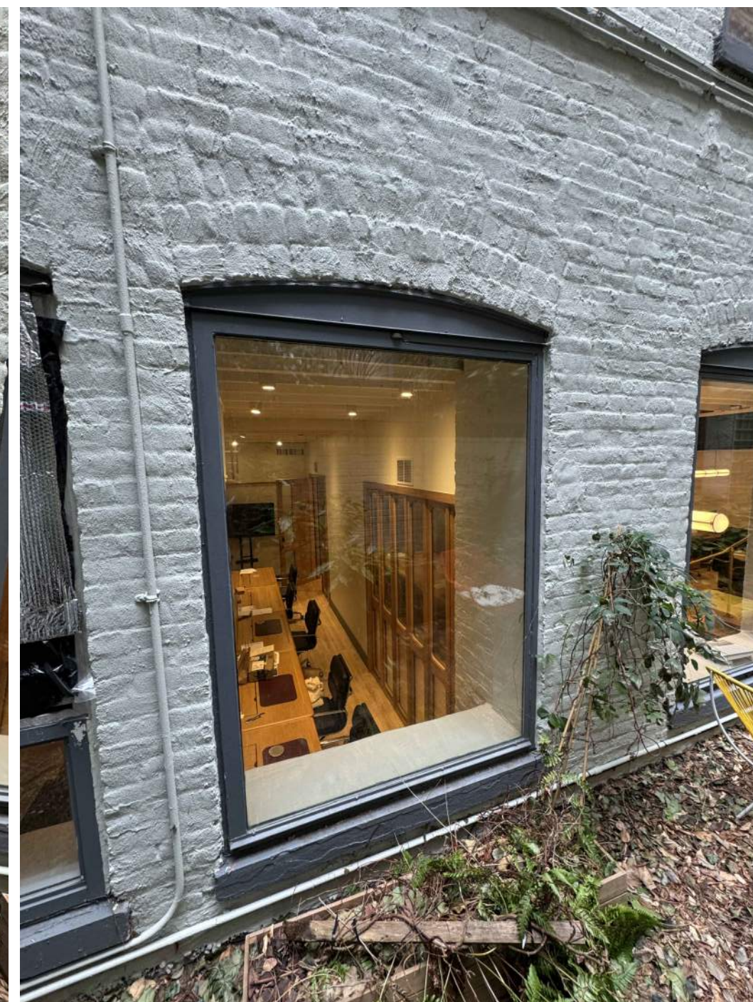
5 EX. CELLAR WINDOW-W 9 F
