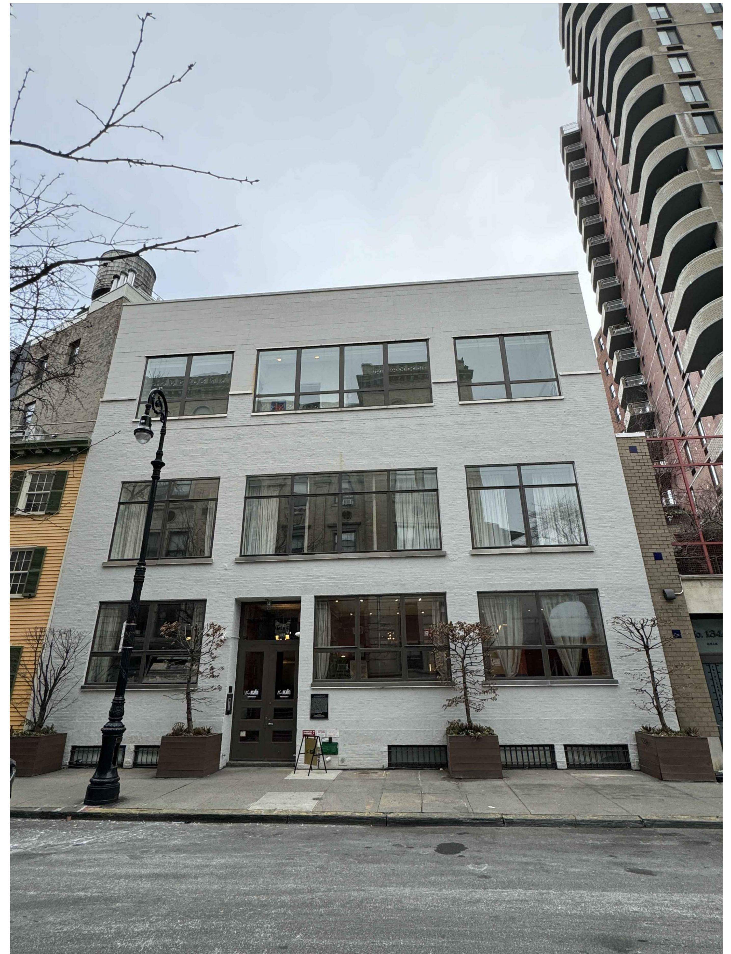
Existing Conditions - Front Facade
