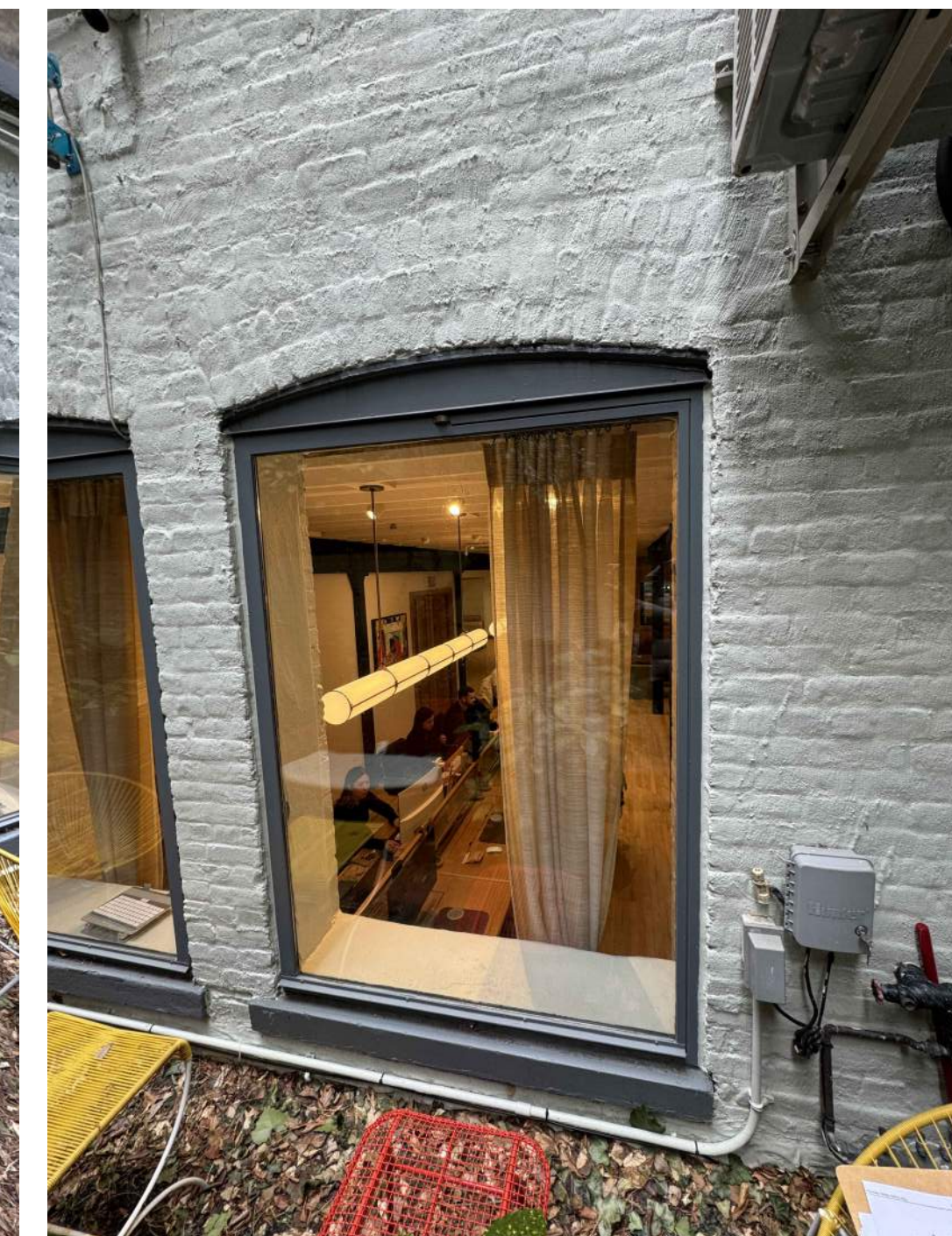
6 EX. CELLAR WINDOW-W 9 F
