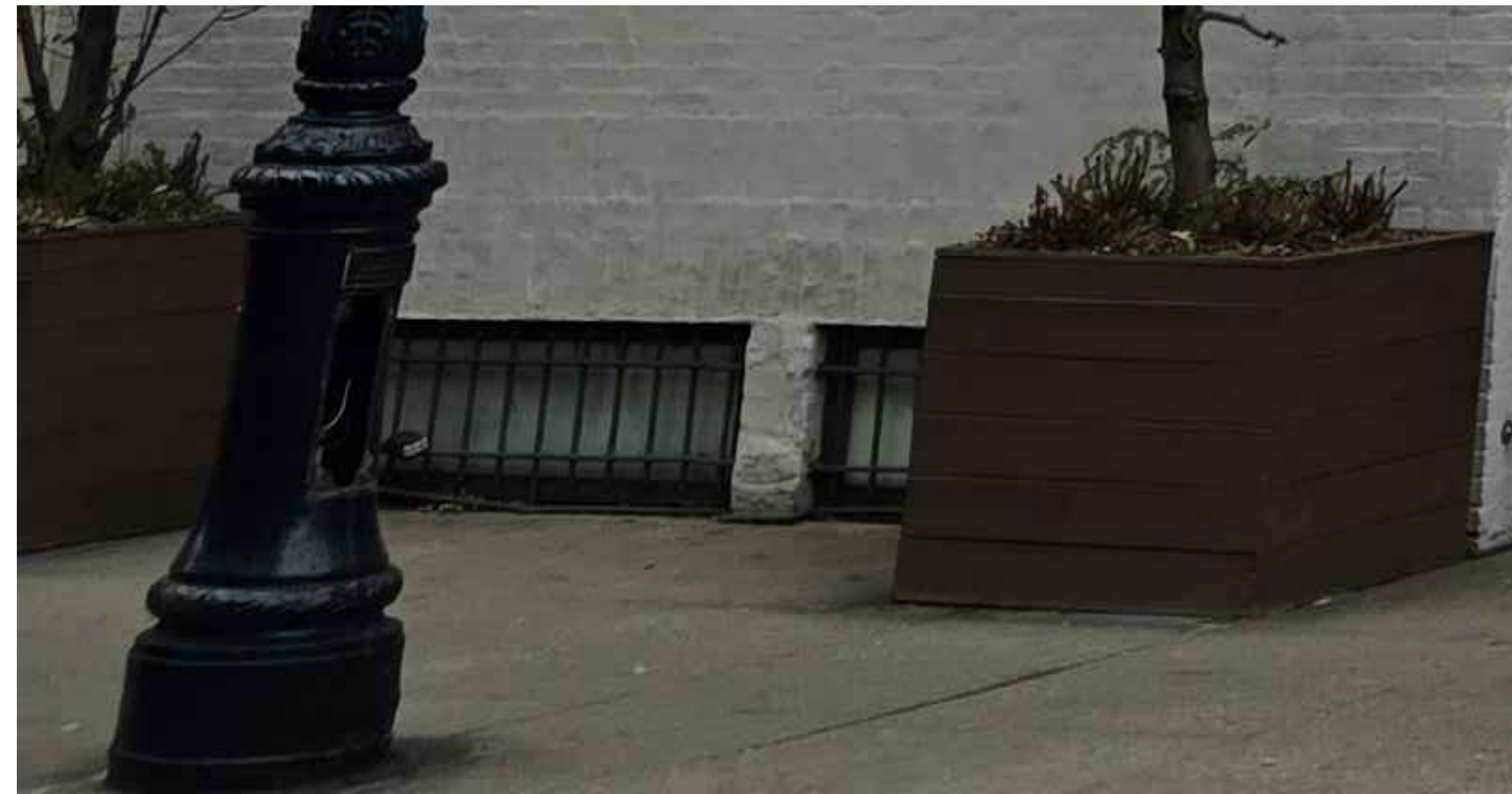
1 EXISTING CELLAR WINDOW- W 1 A (A)
