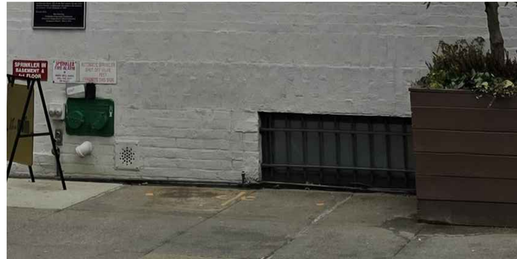
2 EXISTING CELLAR WINDOW- W 1 B (A)
