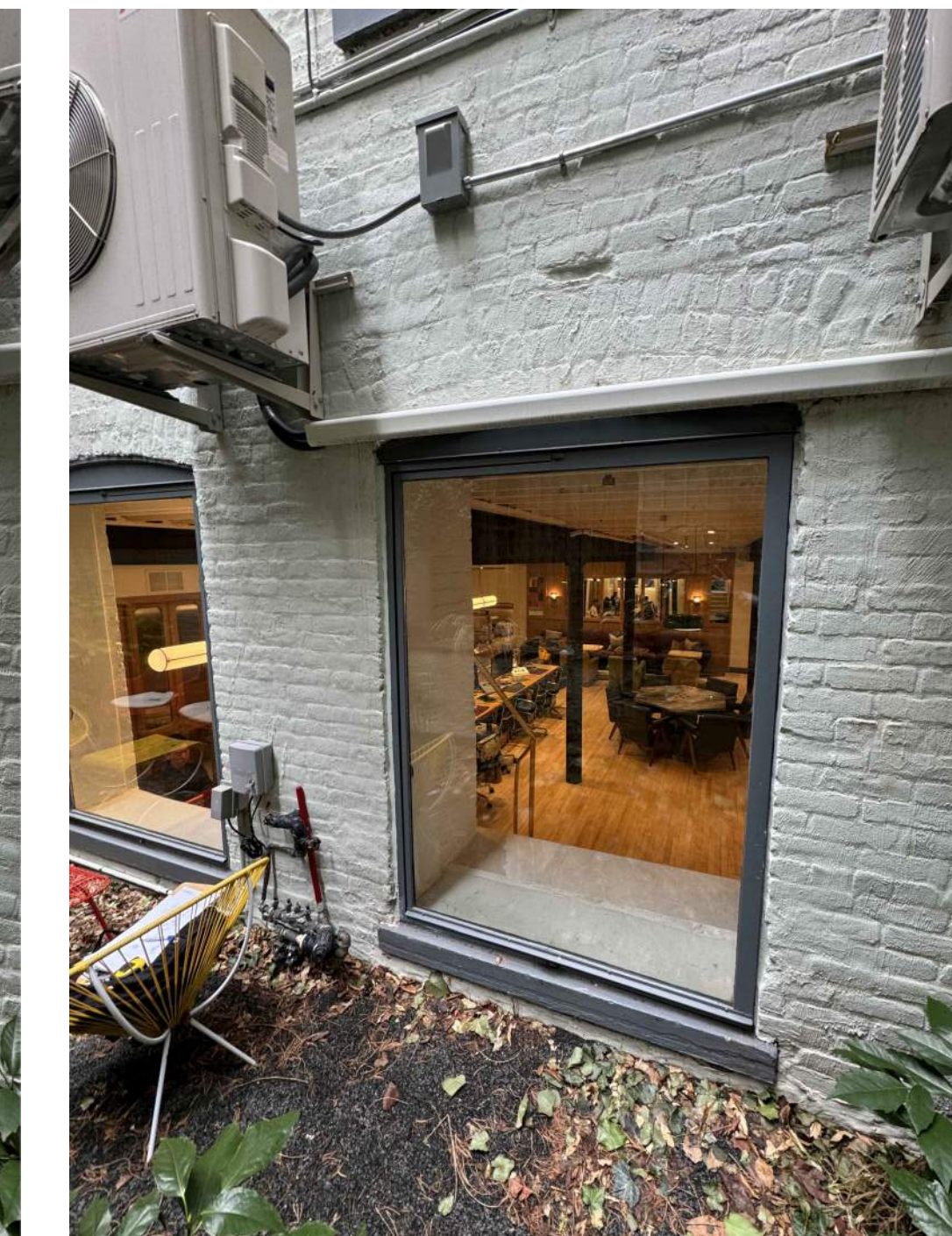
8 EX. CELLAR WINDOW-W 9 F
