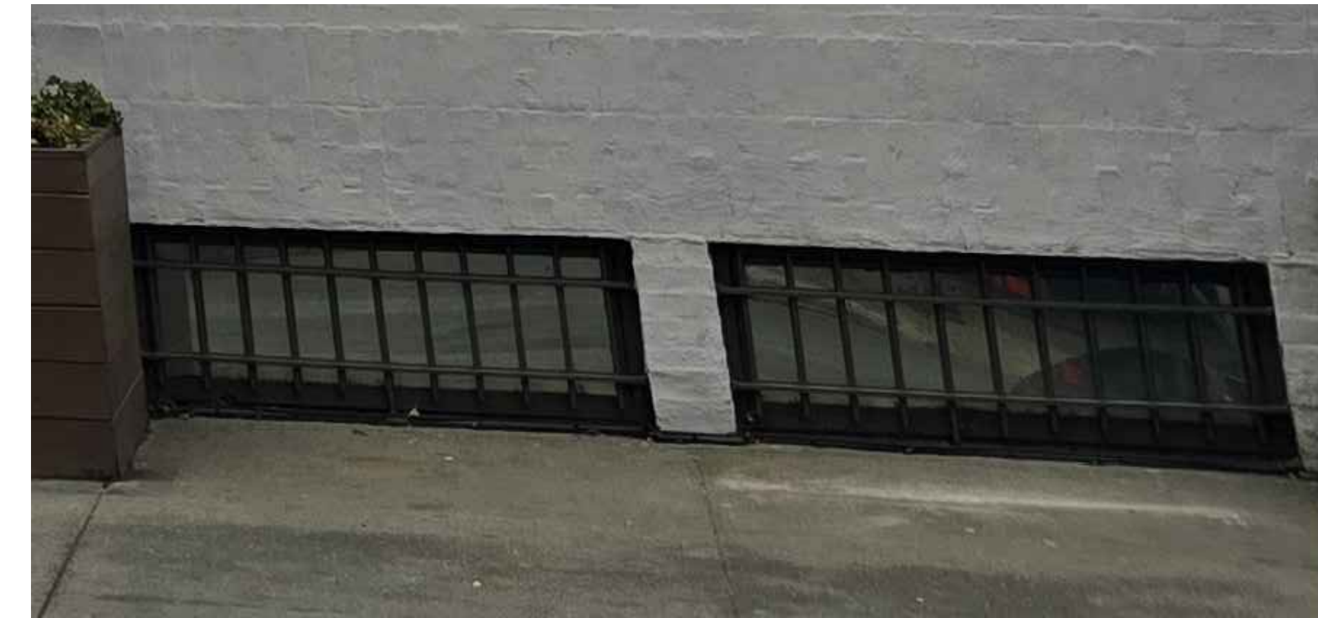
3 EXISTING CELLAR WINDOW-W 1 B (A)
