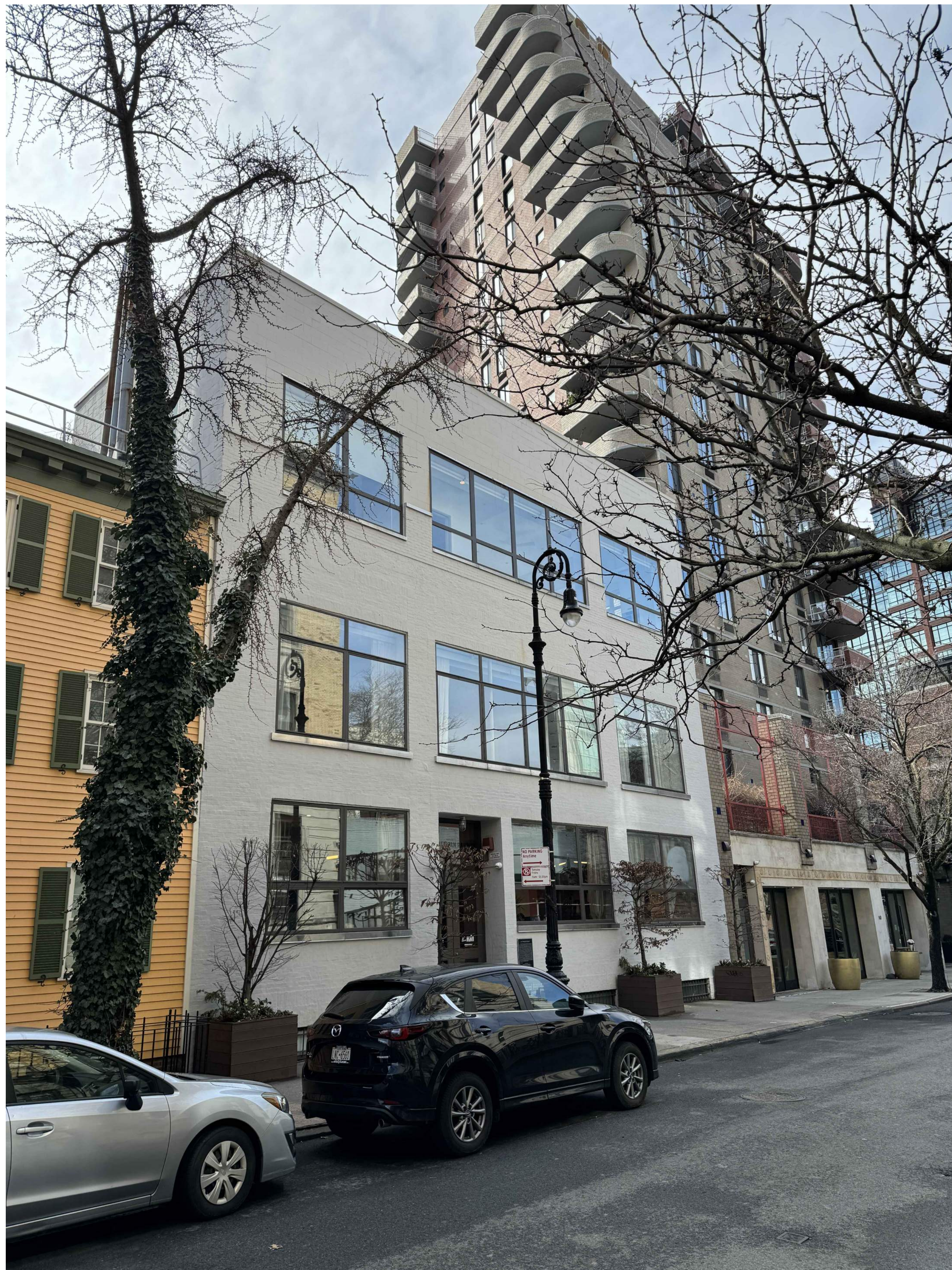
Existing Conditions - Front Facade
