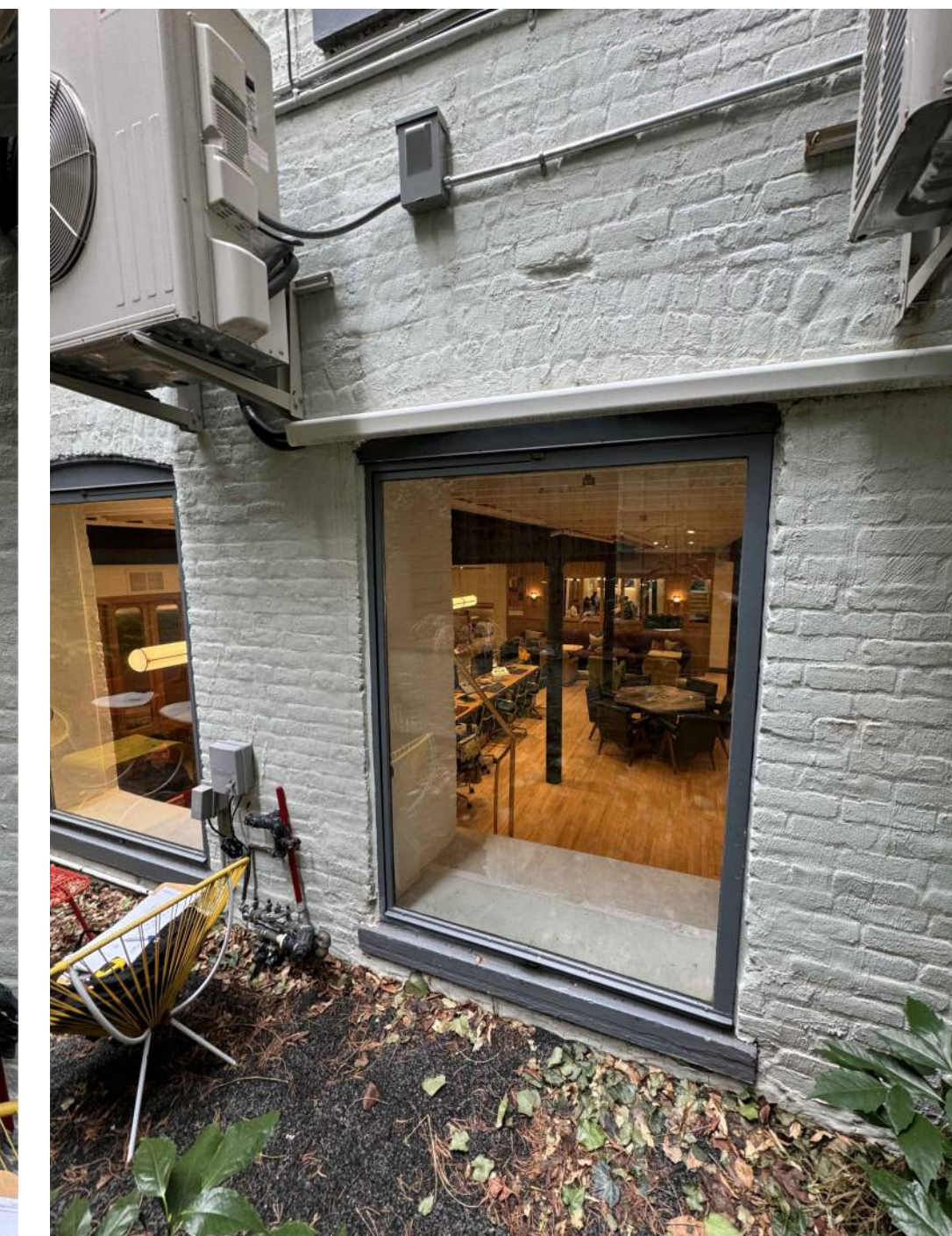
7 EX. CELLAR WINDOW-W 10 G
