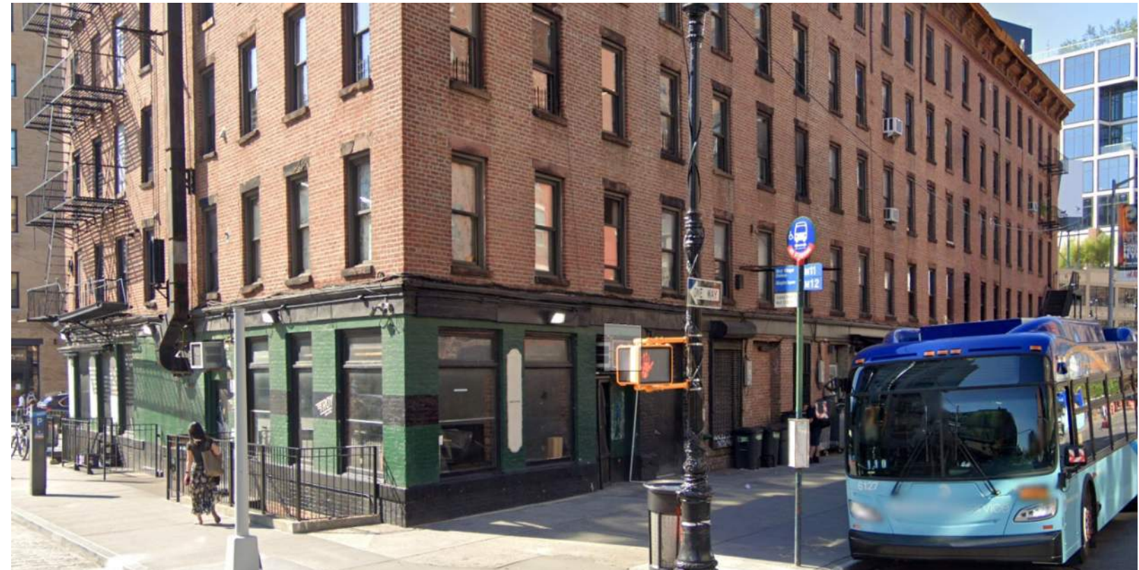
Hudson St / 13th St corner - 2022
