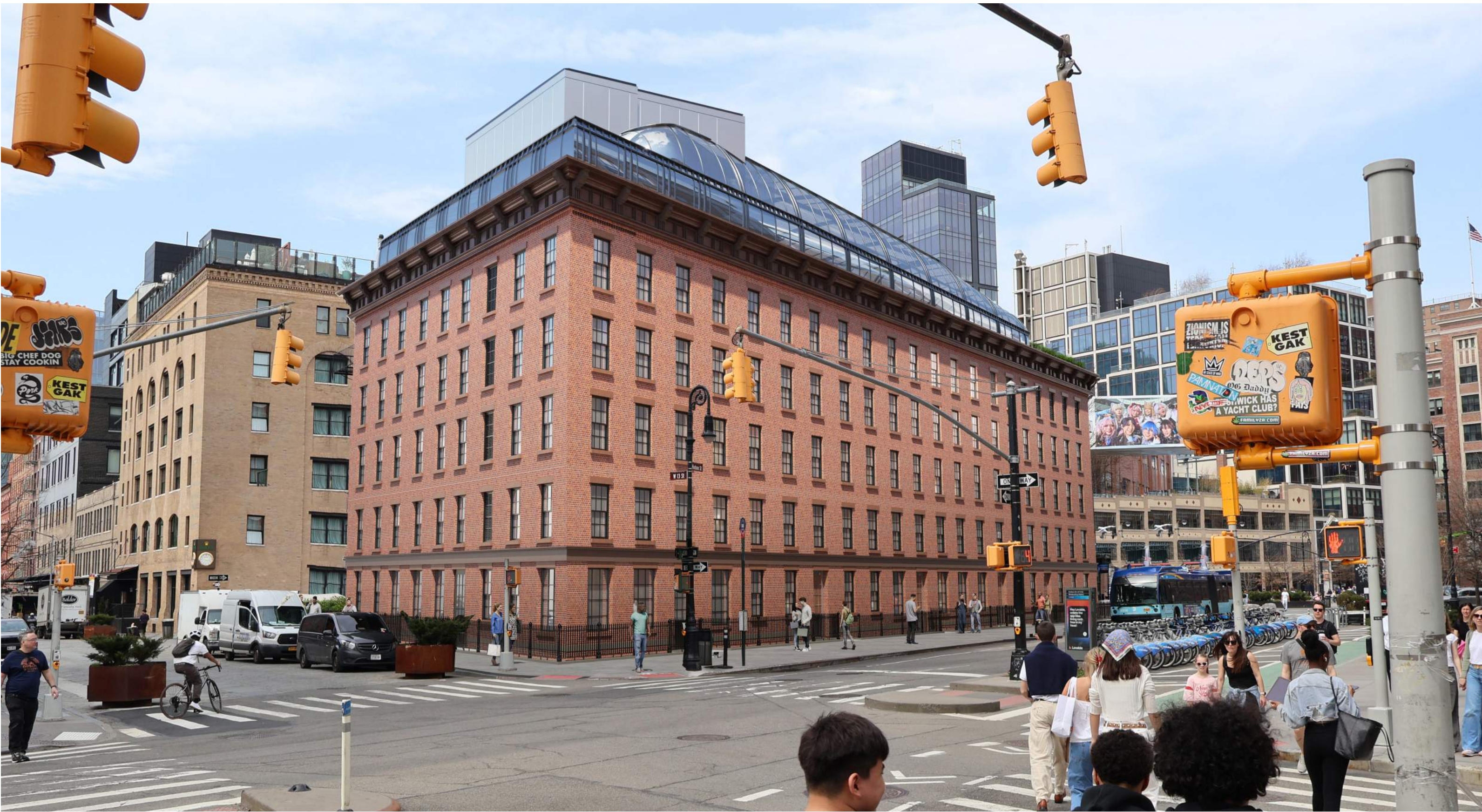
STREET VIEW: HUDSON & WEST 13TH ST. 675 HUDSON STREET
