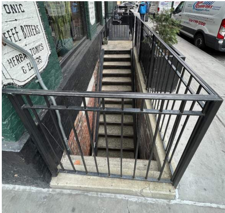
EXISTING AREAWAY RAILING
