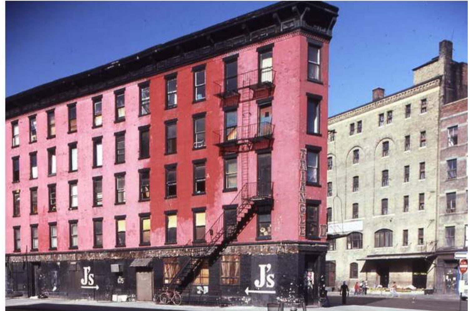
HUDSON STREET ca. 1990 (Village Preservation)
