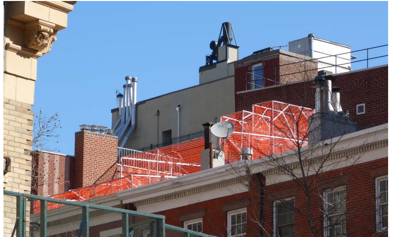
Detail view from west across Washington and Bank Streets
