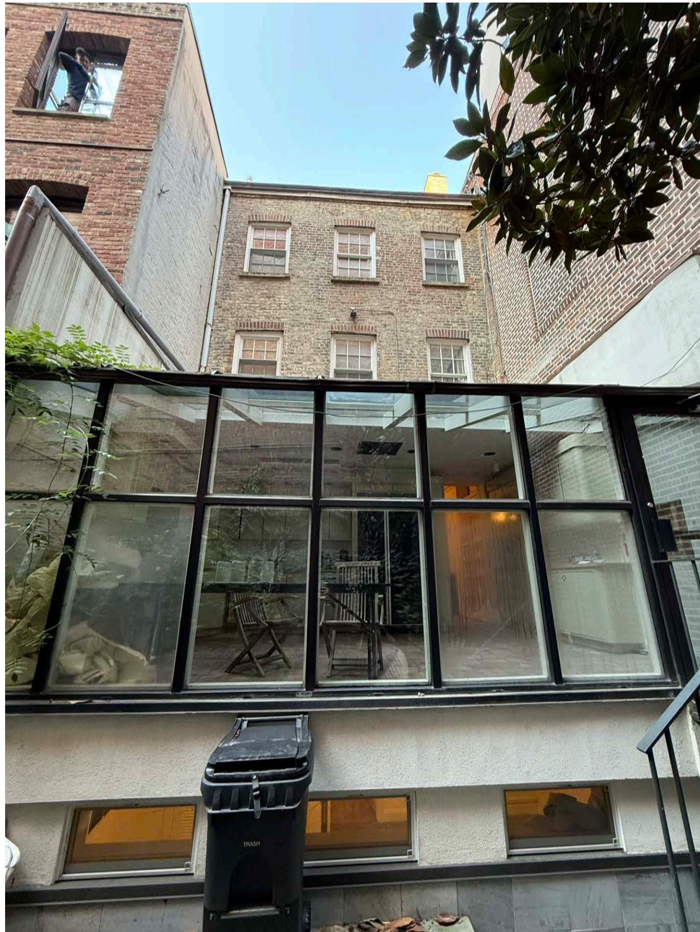
Existing rear extension
