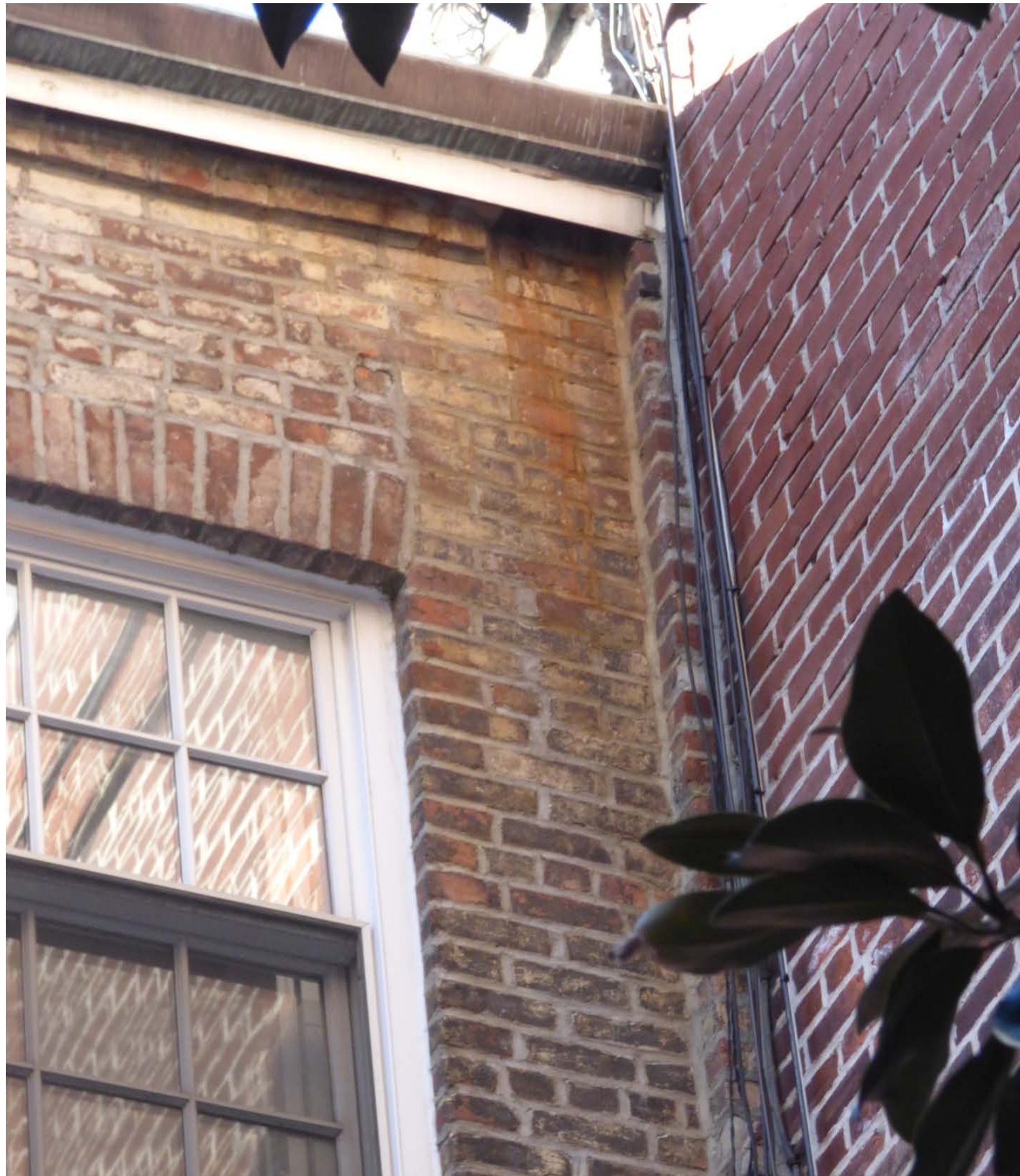
Existing Conditions - Rear Facade Details
