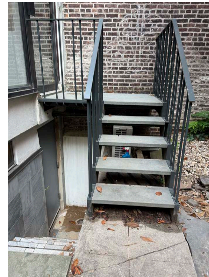
View of rear yard cellar stairs, looking north
