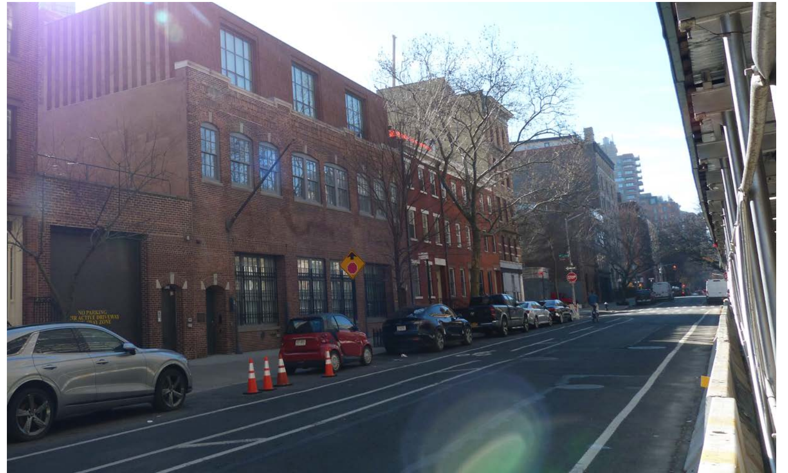
View to the southeast along Washington with the guardrail visible at the primary facade roof deck
