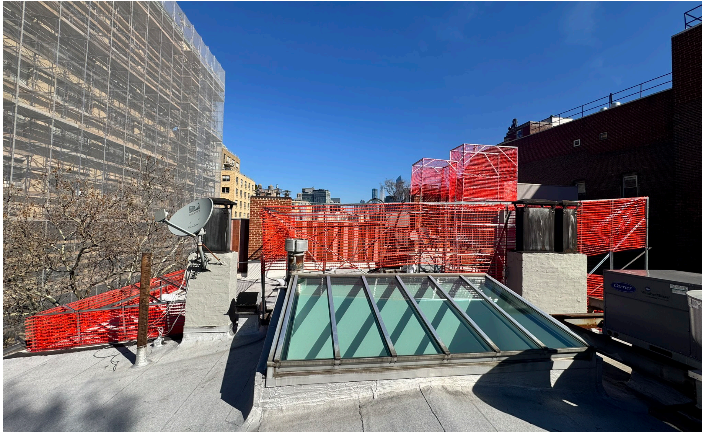
View of mockup on the roof facing north
